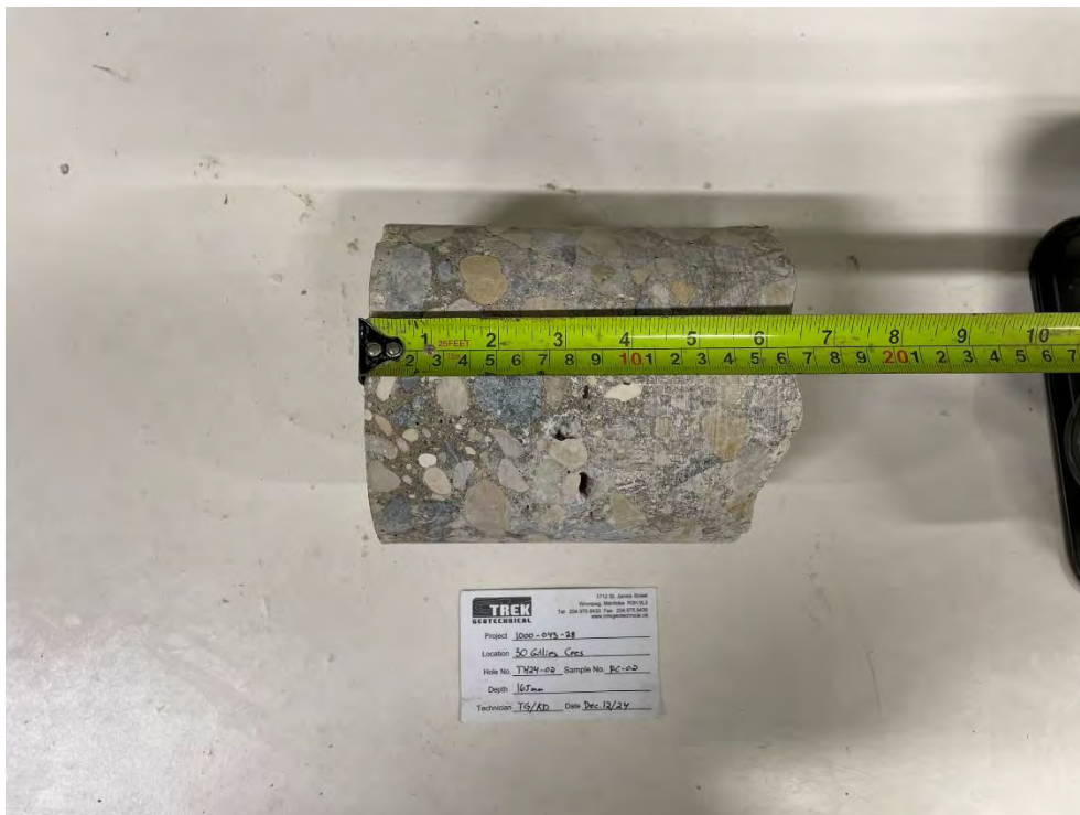
Photo 2: Pavement Core Sample at Test Hole TH24-02
