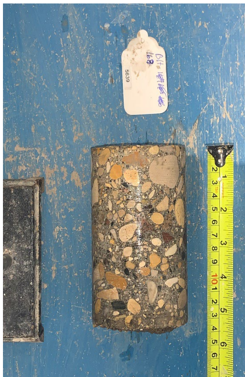
Figure 5 – Core Sample No. 168 – Perth Ave
