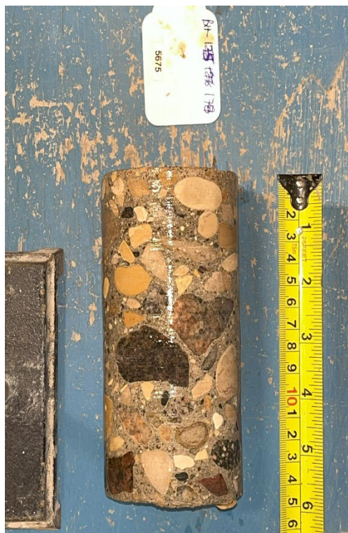
Figure 15 – Core Sample No. 178 – Seaforth Ave
