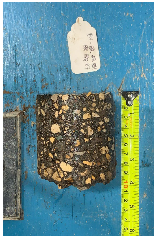
Figure 7 – Core Sample No. 87 – Middle Gate
