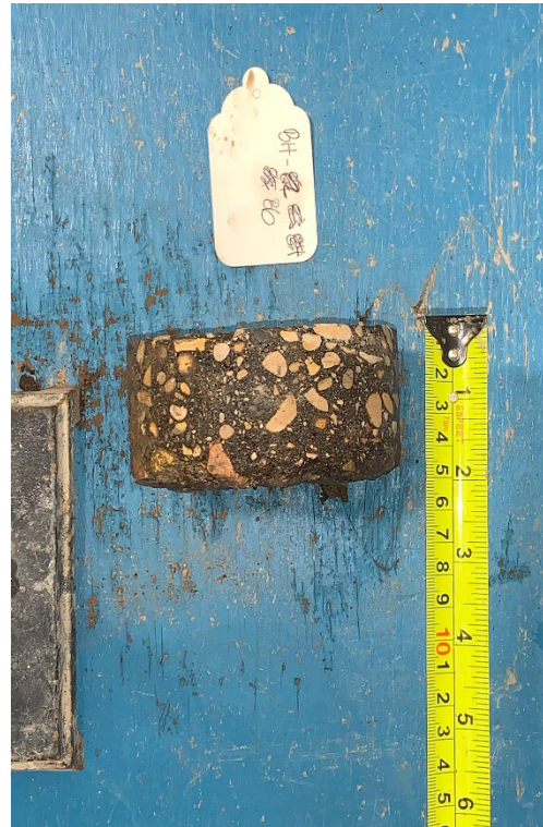
Figure 6 – Core Sample No. 86 – West Gate
