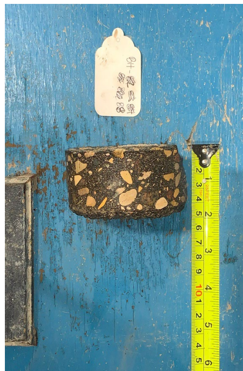
Figure 8 – Core Sample No. 88 – Middle Gate
