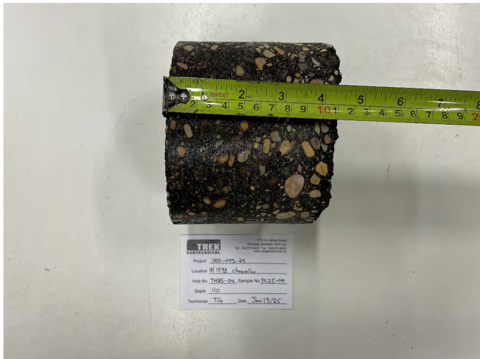
Photo 2: Pavement Core Sample at TH25-04
