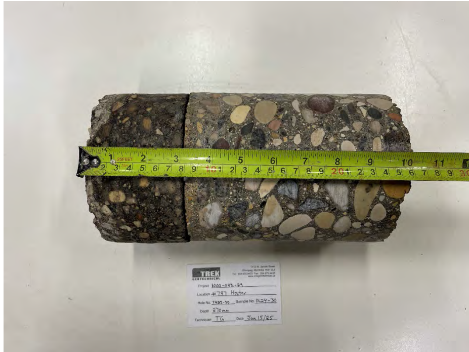
Photo 1: Pavement Core Sample at PC25-30
