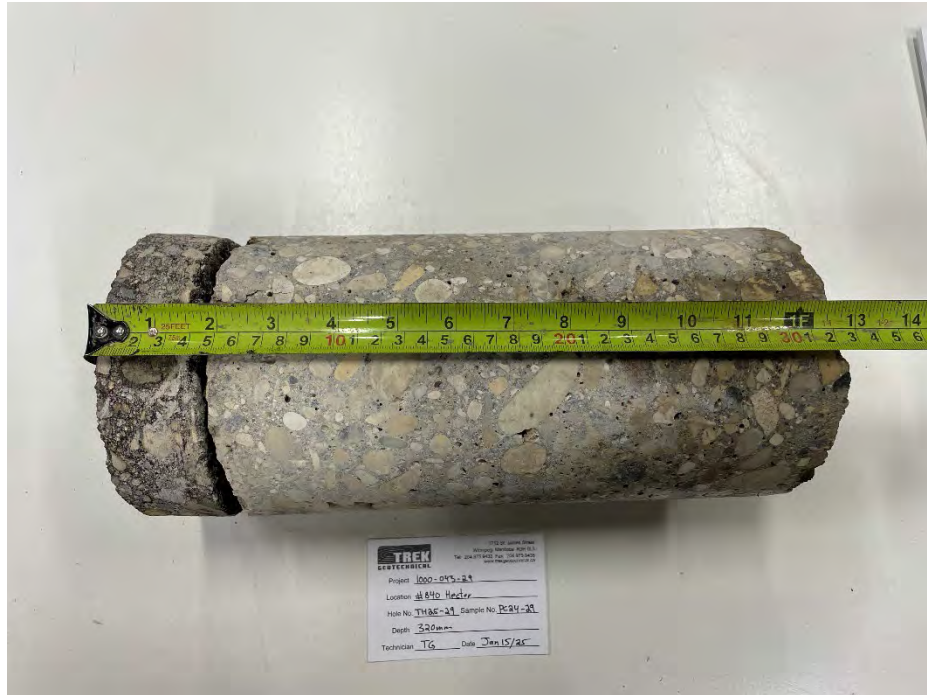
Photo 1: Pavement Core Sample at PC25-29
