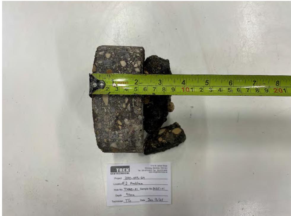
Photo 1: Pavement Core Sample at TH25-01
