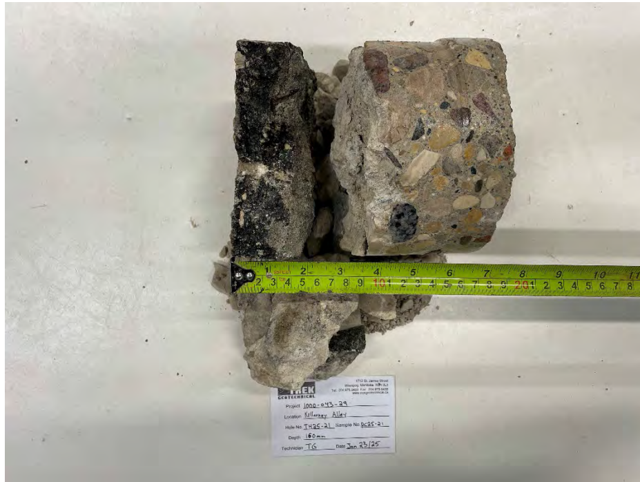
Photo 1: Pavement Core Sample at TH25-21
