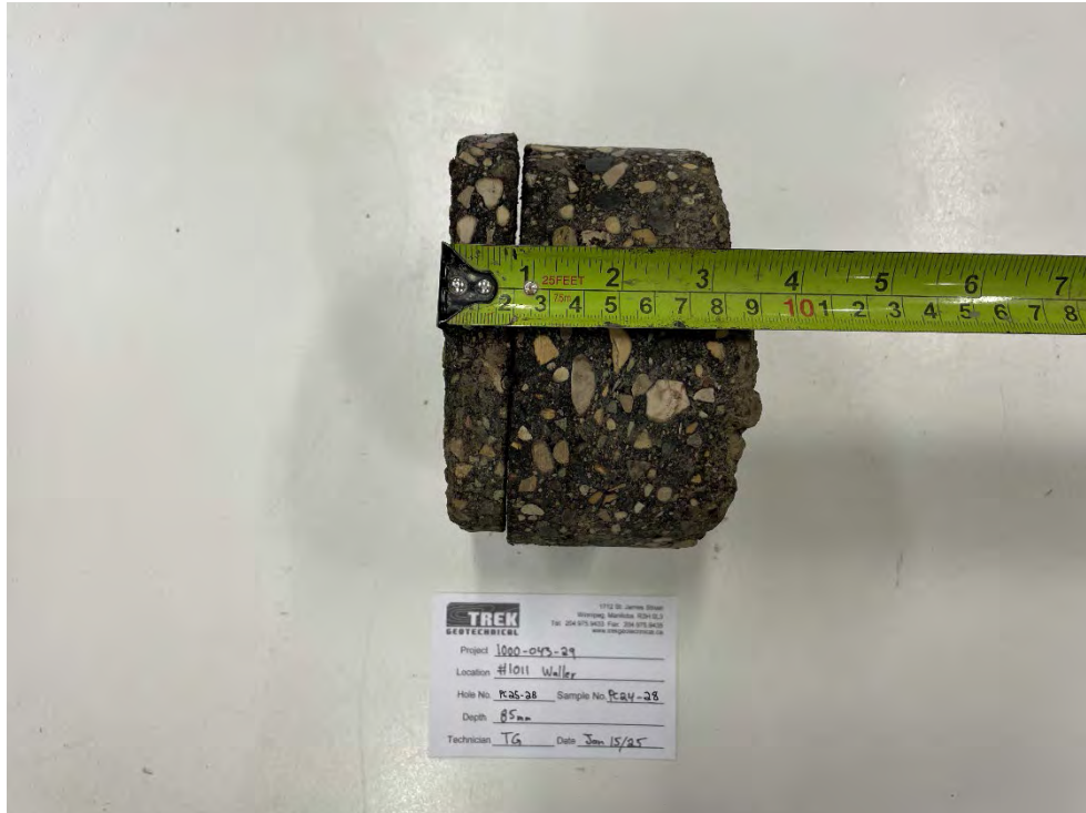
Photo 3: Pavement Core Sample at PC25-28
