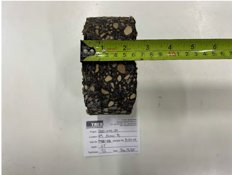
Photo 1: Pavement Core Sample at TH25-02
