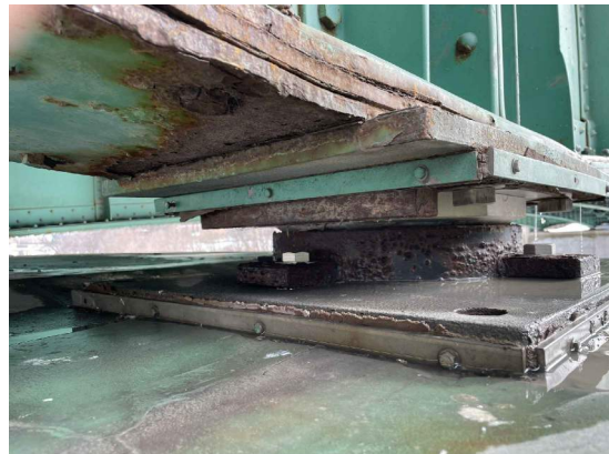
PHOTO OF EXISTING MK. 11 BEARING AT PIER 2 (LOOKING SOUTHEAST)
