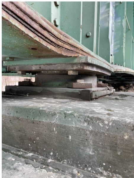
PHOTO OF EXISTING MK. 10 BEARING AT PIER 1 (LOOKING SOUTHEAST)
