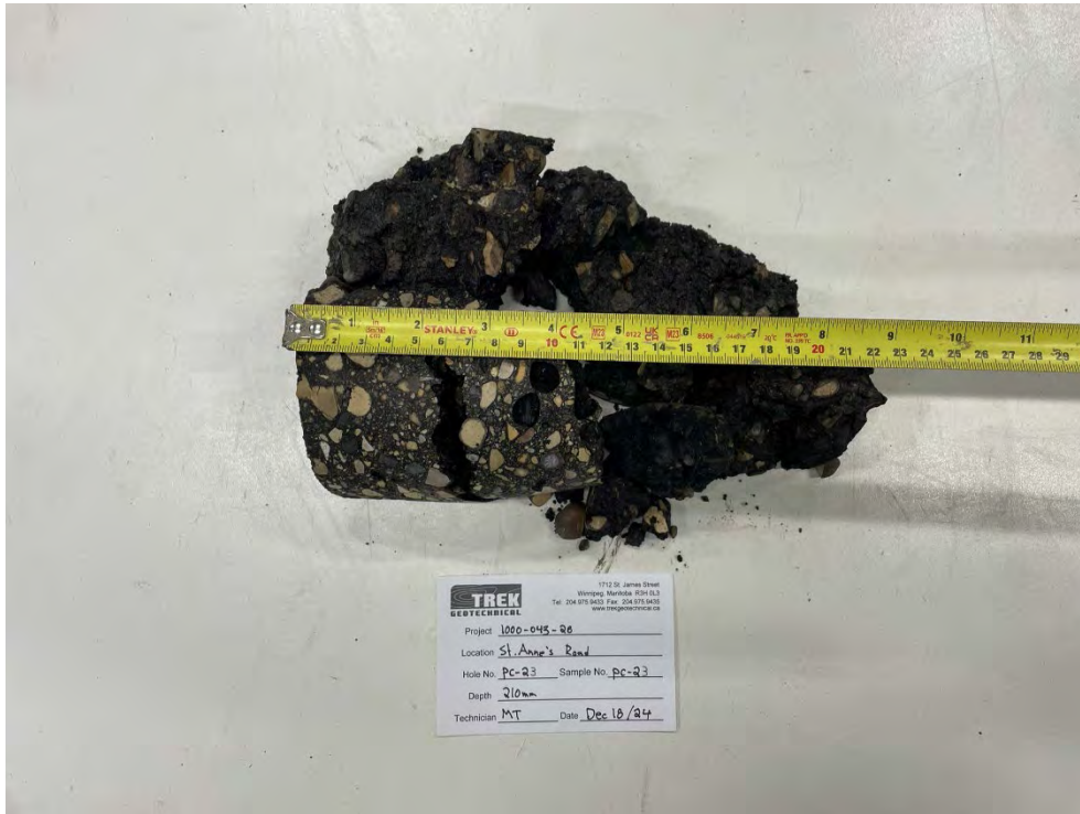
Photo 23: Pavement Core Sample at PC-23
