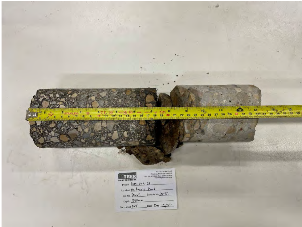
Photo 27: Pavement Core Sample at PC-27
