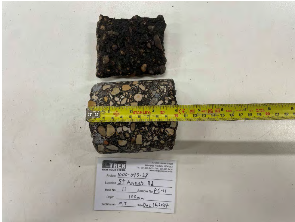
Photo 11: Pavement Core Sample at PC-11
