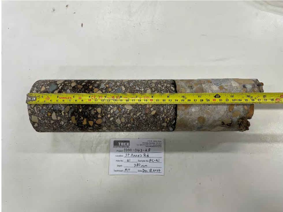
Photo 21: Pavement Core Sample at PC-21
