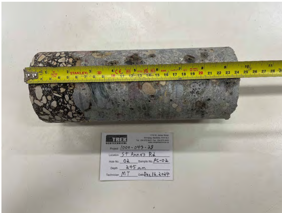
Photo 2: Pavement Core Sample at PC-02
