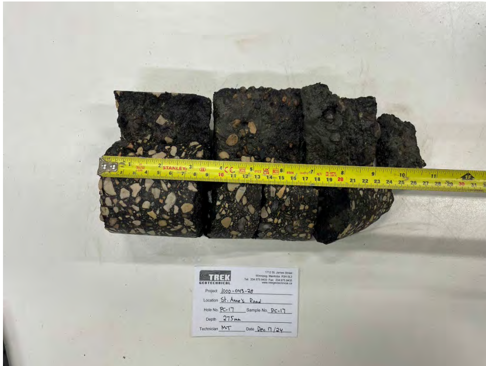
Photo 17: Pavement Core Sample at PC-17
