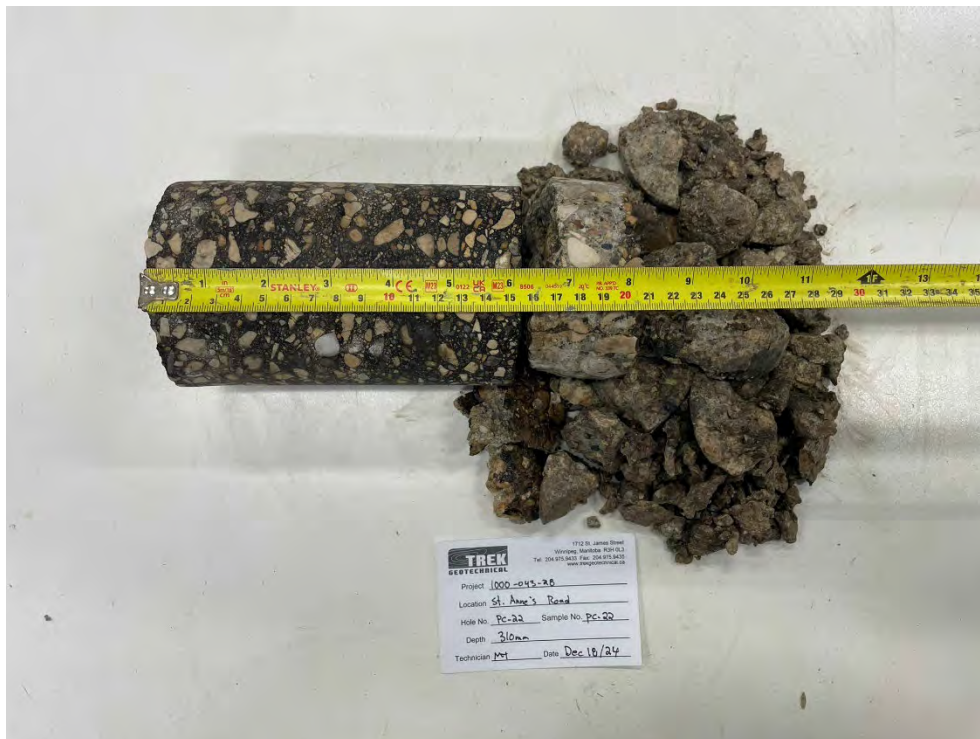
Photo 22: Pavement Core Sample at PC-22
