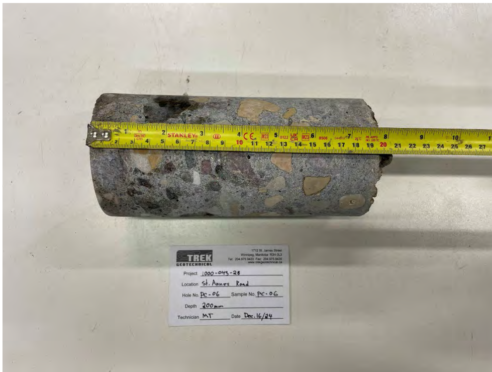
Photo 6: Pavement Core Sample at PC-06
