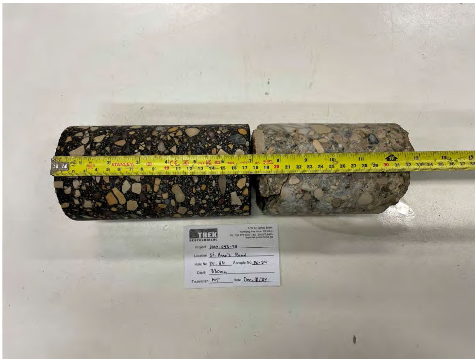
Photo 24: Pavement Core Sample at PC-24
