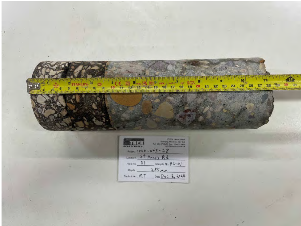
Photo 1: Pavement Core Sample at PC-01
