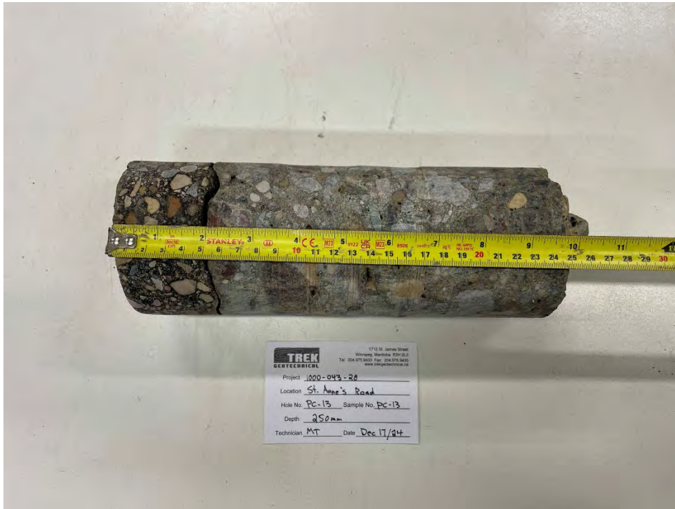
Photo 13: Pavement Core Sample at PC-13
