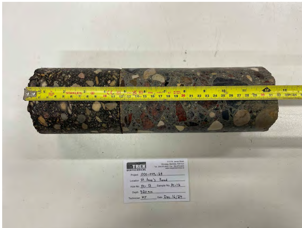
Photo 12: Pavement Core Sample at PC-12
