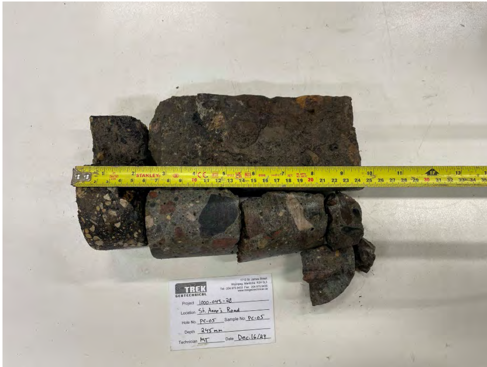
Photo 5: Pavement Core Sample at PC-05
