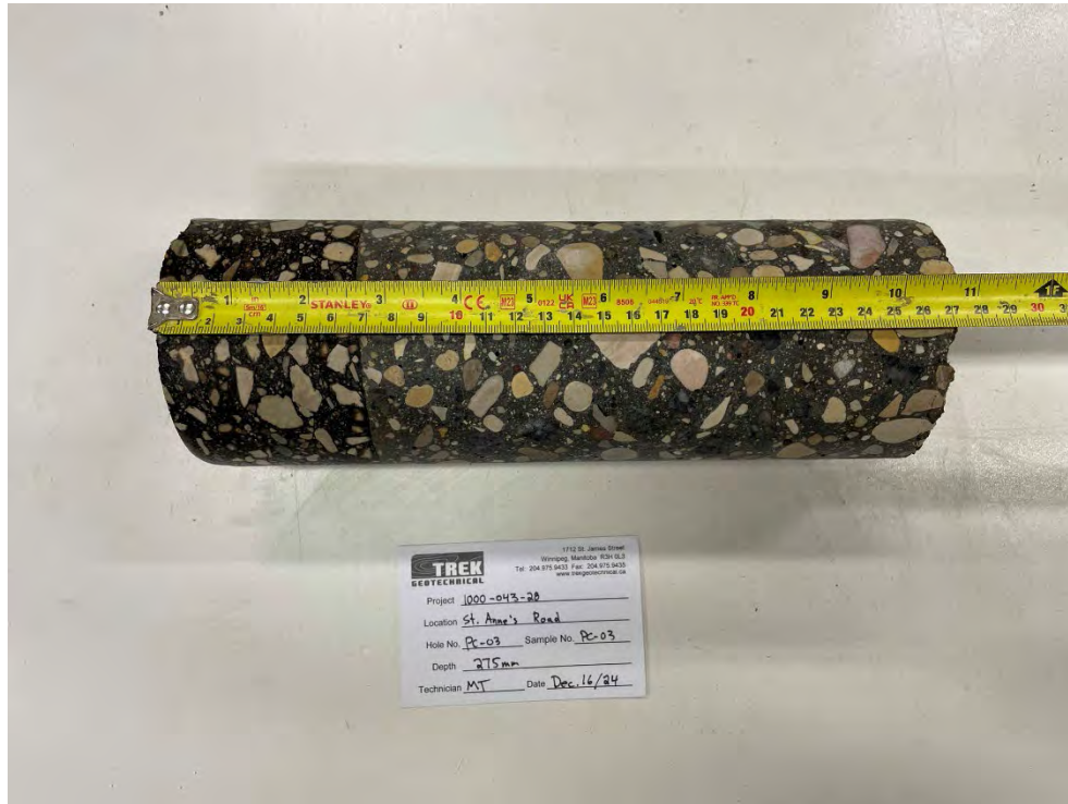
Photo 3: Pavement Core Sample at PC-03
