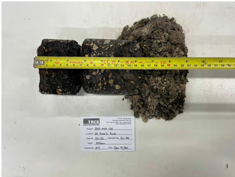
Photo 26: Pavement Core Sample at PC-26
