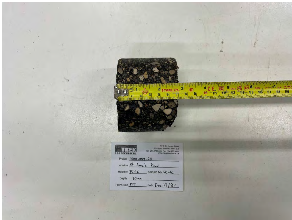
Photo 16: Pavement Core Sample at PC-16
