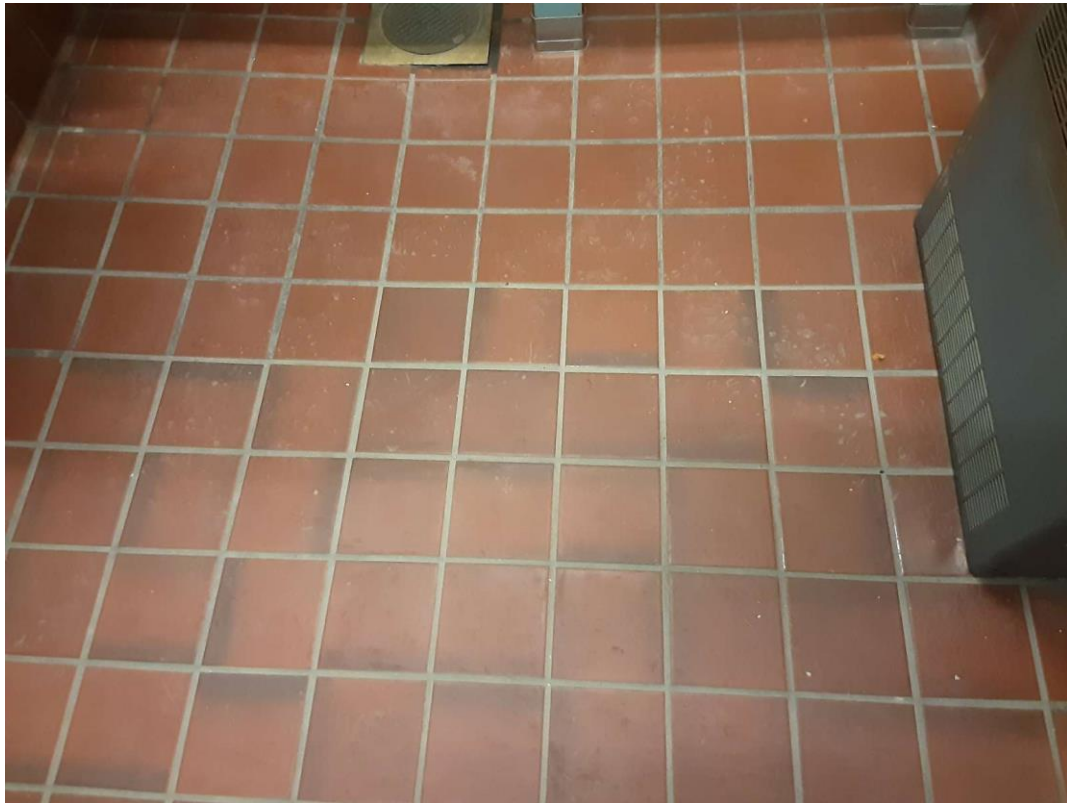
V9500 (Presumed Asbestos), Floor, All, Mortar, Washroom (Location #: 3)
