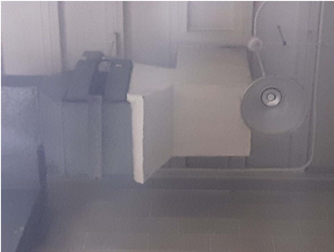
V0005 (Confirmed Asbestos), Duct, Fresh Air Intake, Fiberglass w/Parging, Ammonia Room (Location #: 11)
