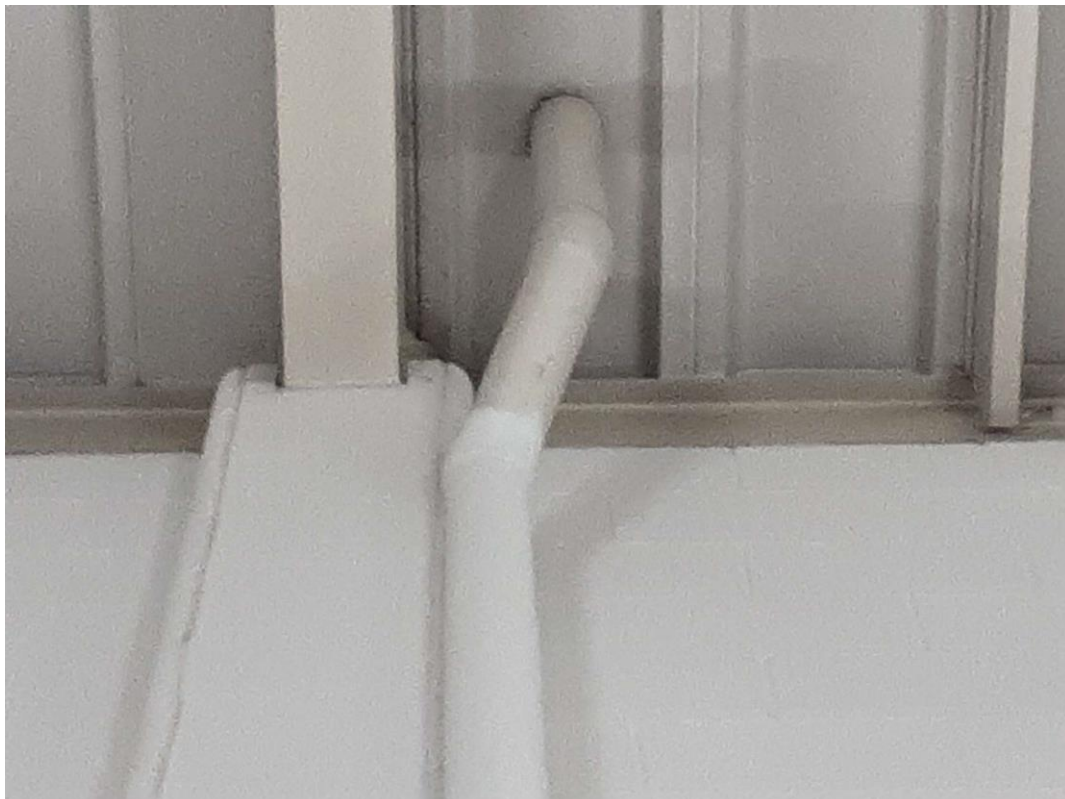
V0004 (Confirmed Asbestos), Piping, Rain Water Leader, Parging over Fiberglass, Chlorine Tonner Room (Location #: 9)
