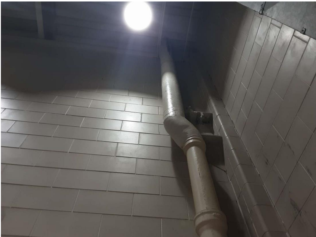
V0004 (Confirmed Asbestos), Piping, Rain Water Leader, Parging over Fibreglass, Ammonia Room (Location #: 11)
