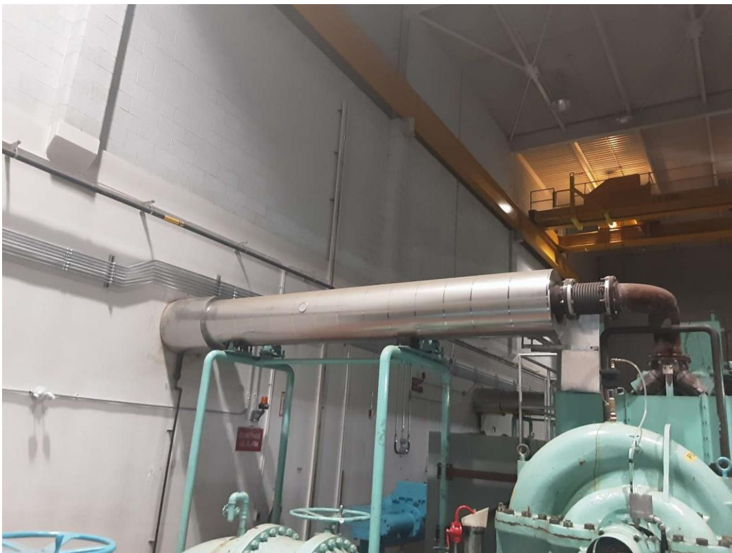
S0003 (Confirmed Asbestos), Duct, Generator Exhaust, Magnesia block, Pump Building - Basement (Location #: 1)
