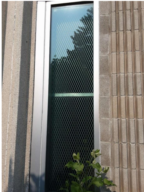
S0010 (Confirmed Asbestos), Wall, Window Liner, Caulking, Hurst Pump Station Main Building Exterior (Location #: 19)
