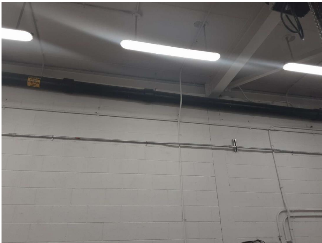
V0001 (Confirmed Asbestos), Piping, Rain Water Leader, Chlorine Building - Chlorine Tonner Room (Location #: 8)
