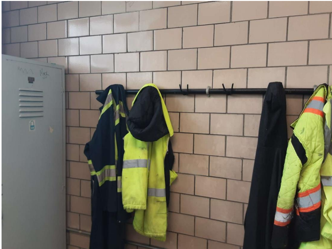
V9500 (Presumed Asbestos), Wall, All, Mortar, Old Pump Building - Locker Room (Location #: 29) setting compound
