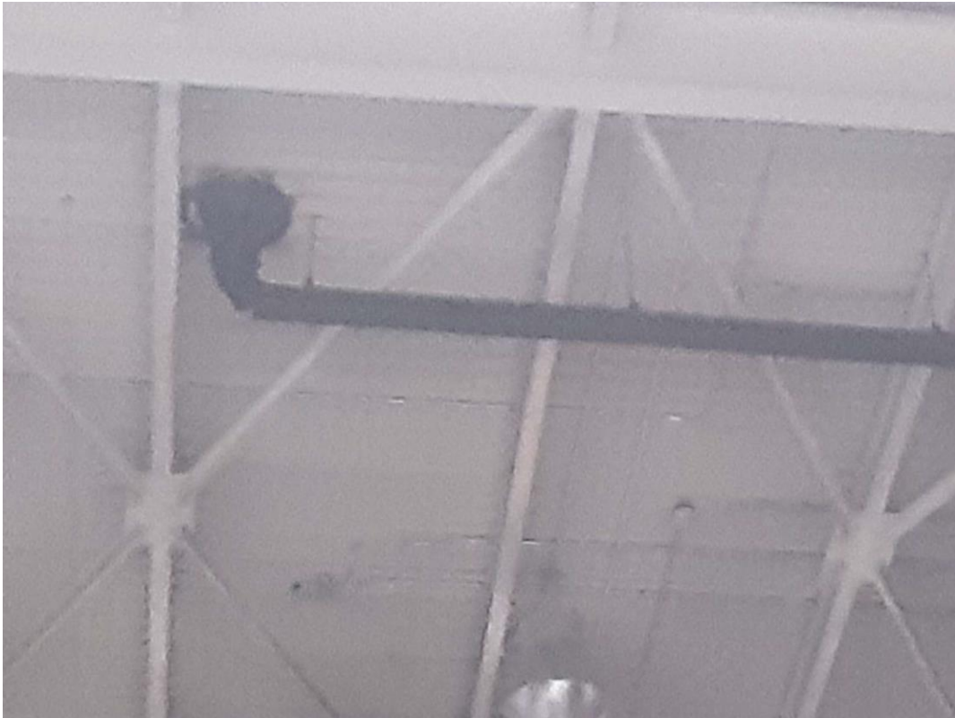
S0001 (Confirmed Asbestos), Piping, Rain Water Leader, Pump Building - Basement (Location #: 1)
