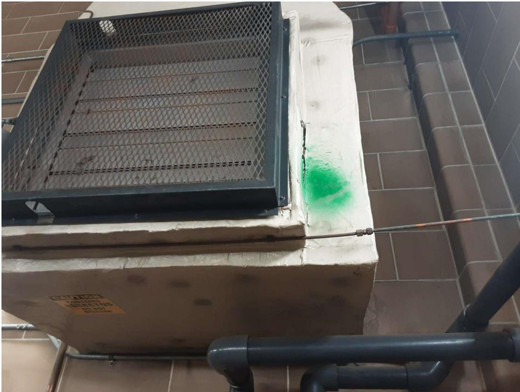
V0005 (Confirmed Asbestos), Duct, Fresh Air Intake, Fiberglass w/Parging, Chlorine Analyzer Room (Location #: 6)
