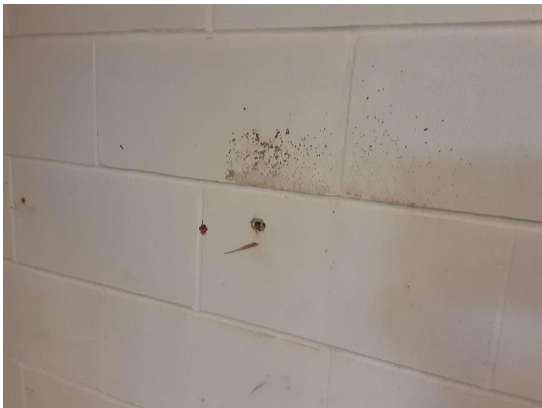
S0025 (Confirmed Asbestos), Wall, Vermiculite/concrete block walls, Old Pump Building - Electrical Room (Location #: 30)
