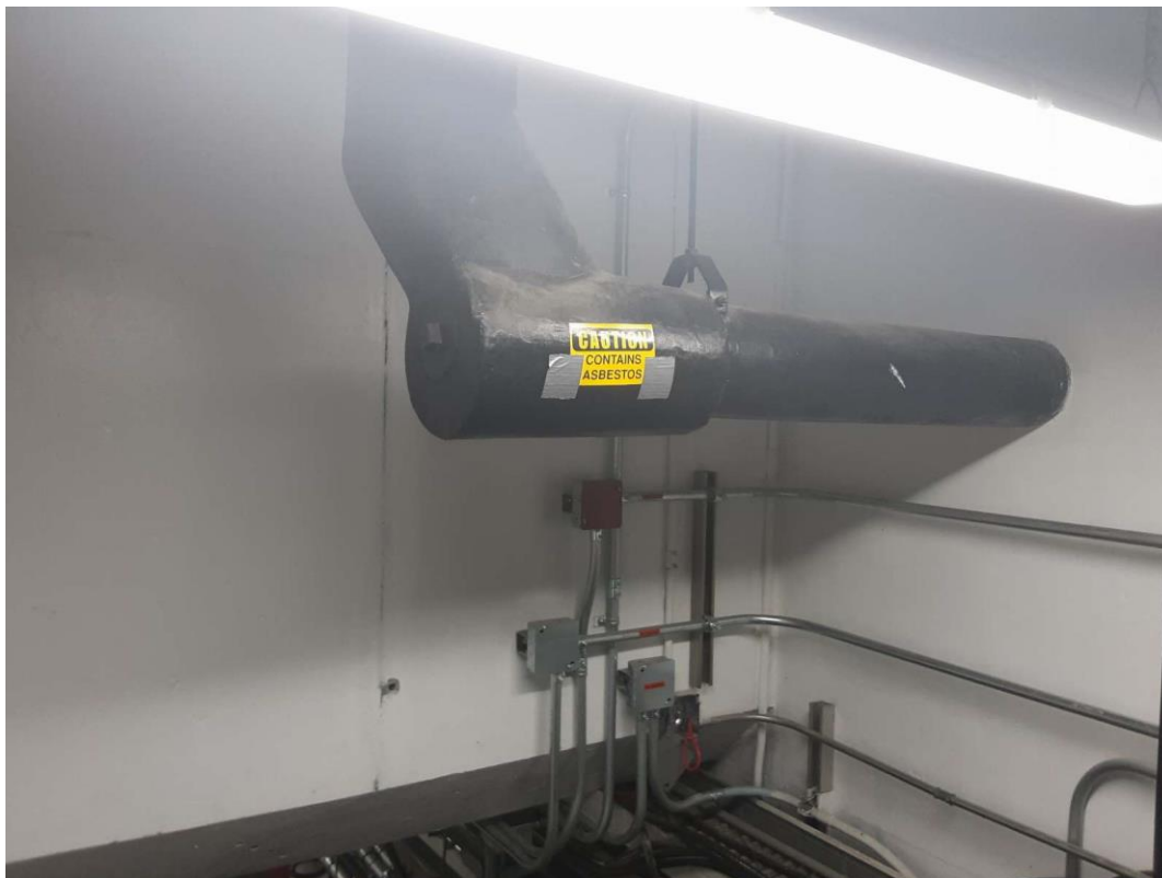
V0001 (Confirmed Asbestos), Piping, Rain Water Leader, Chlorine Building - Stairwell (Location #: 11)
