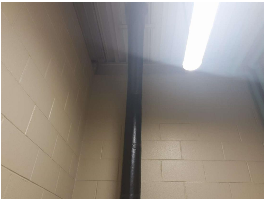
V0007 (Confirmed Asbestos), Piping, Rain Water Leader, Parging over Fibreglass, Pump Building - Chlorine Analyzer Room (Location #: 2)
