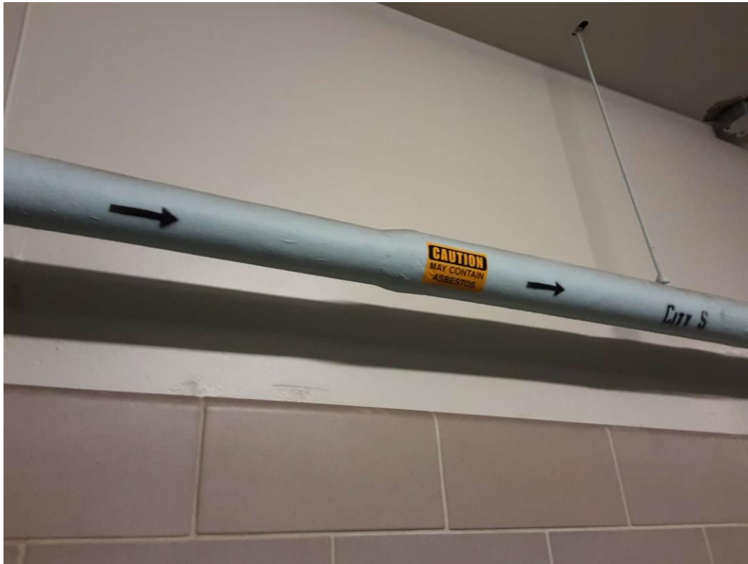
V0004 (None), Piping, Domestic Water (Hot and Cold), Abated Material, North Mezzanine (Location #: 15)
