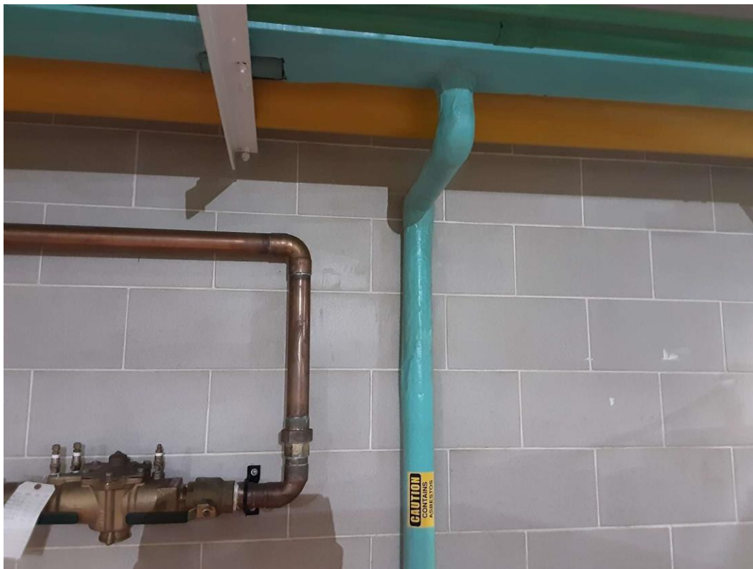
V0002 (Confirmed Asbestos), Piping, Domestic Water (Hot and Cold), Parging over Fiberglass, Pump Floor (Location #: 19)
