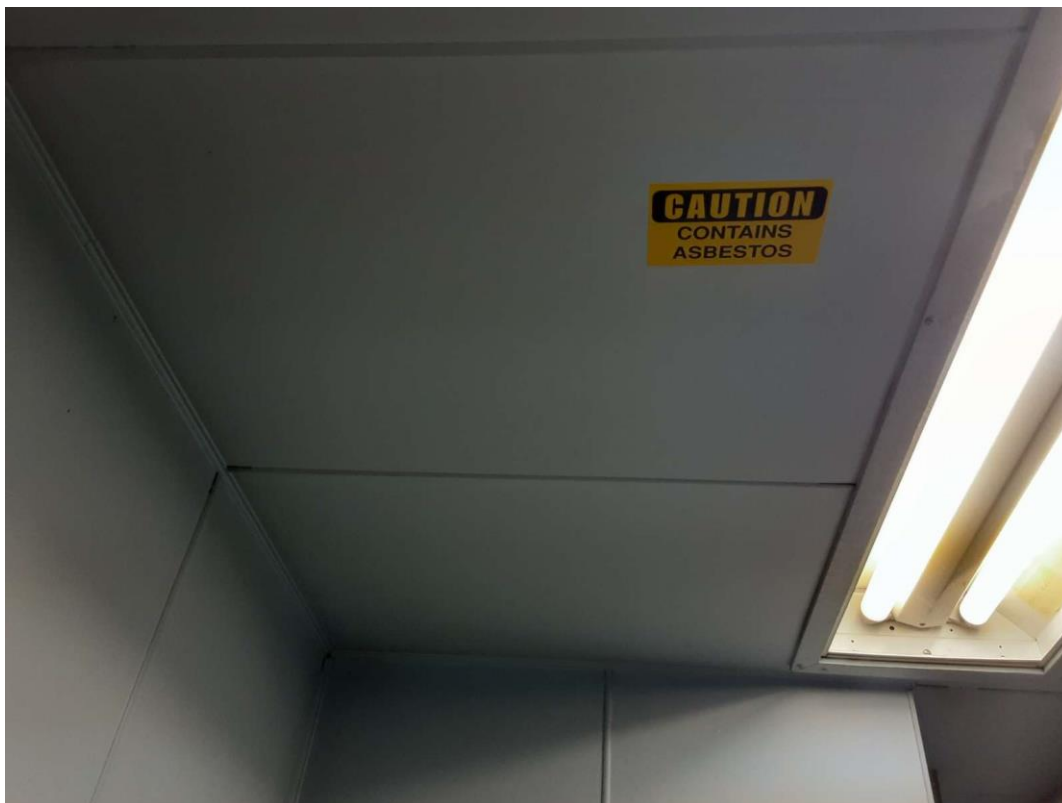
V9000 (Confirmed Asbestos), Ceiling, Cement Product, Old Pump Building - Washroom (Location #: 16)
