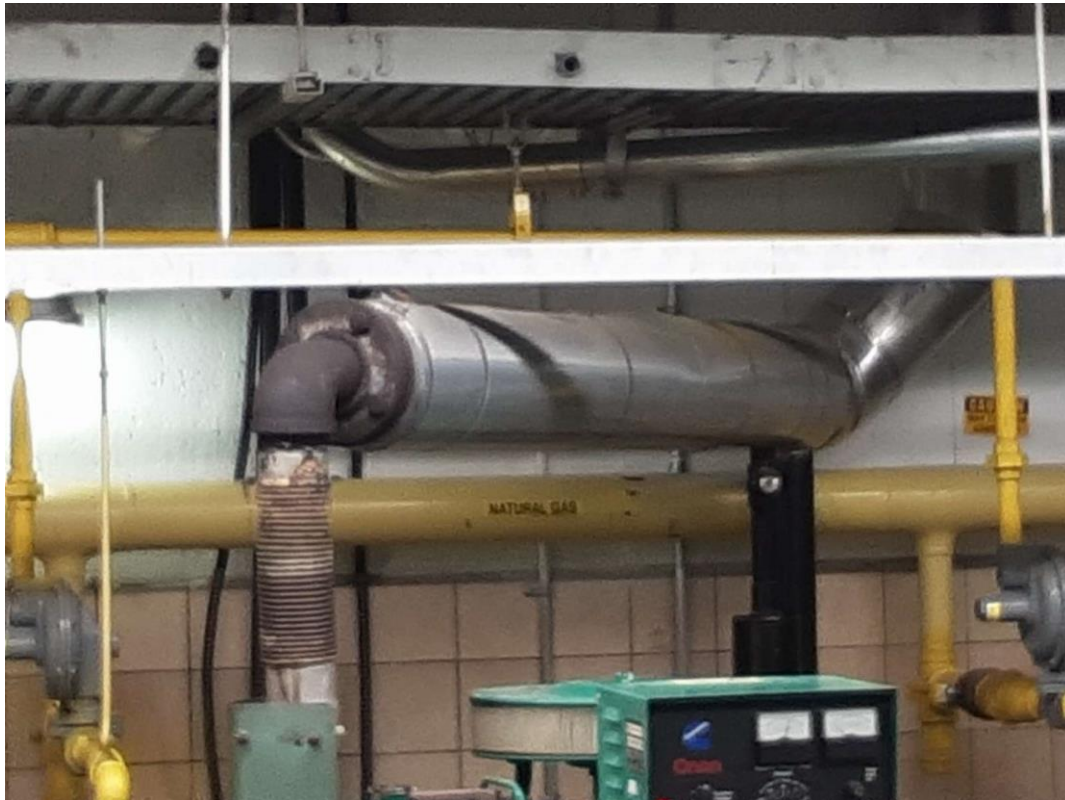
S0003 (Confirmed Asbestos), Mechanical Equipment, Generator Exhaust, Magnesia block, Main Building - Pump Room (Location #: 10)
