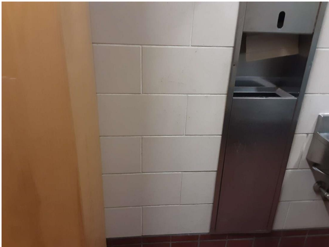
V9500 (Presumed Asbestos), Wall, All, Vermiculite/concrete block walls, Washroom (Location #: 3)
