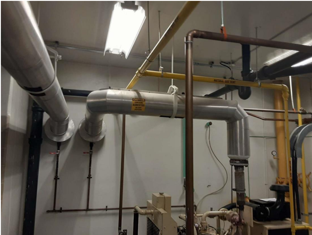
S0006 (Confirmed Asbestos), Mechanical Equipment, Generator Exhaust, Magnesia block, Generator Room (Location #: 18)
