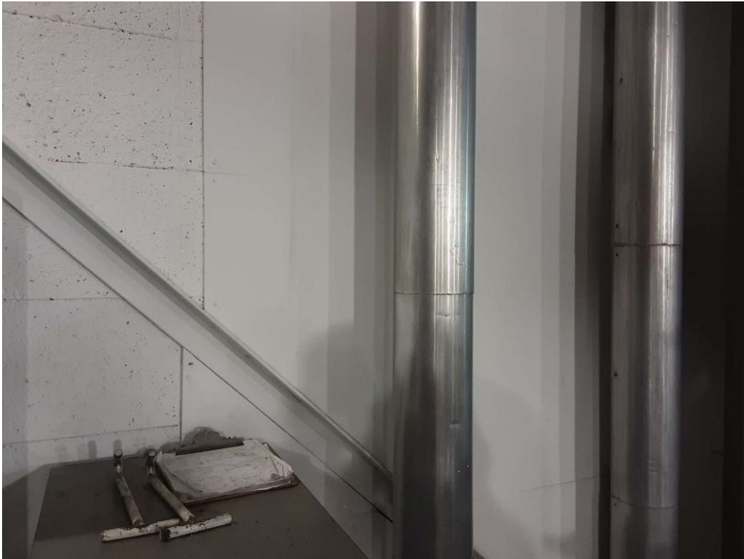
V0006 (Confirmed Asbestos), Wall, Cement Product, Main Building - Landing/Loading Area (Location #: 5)
