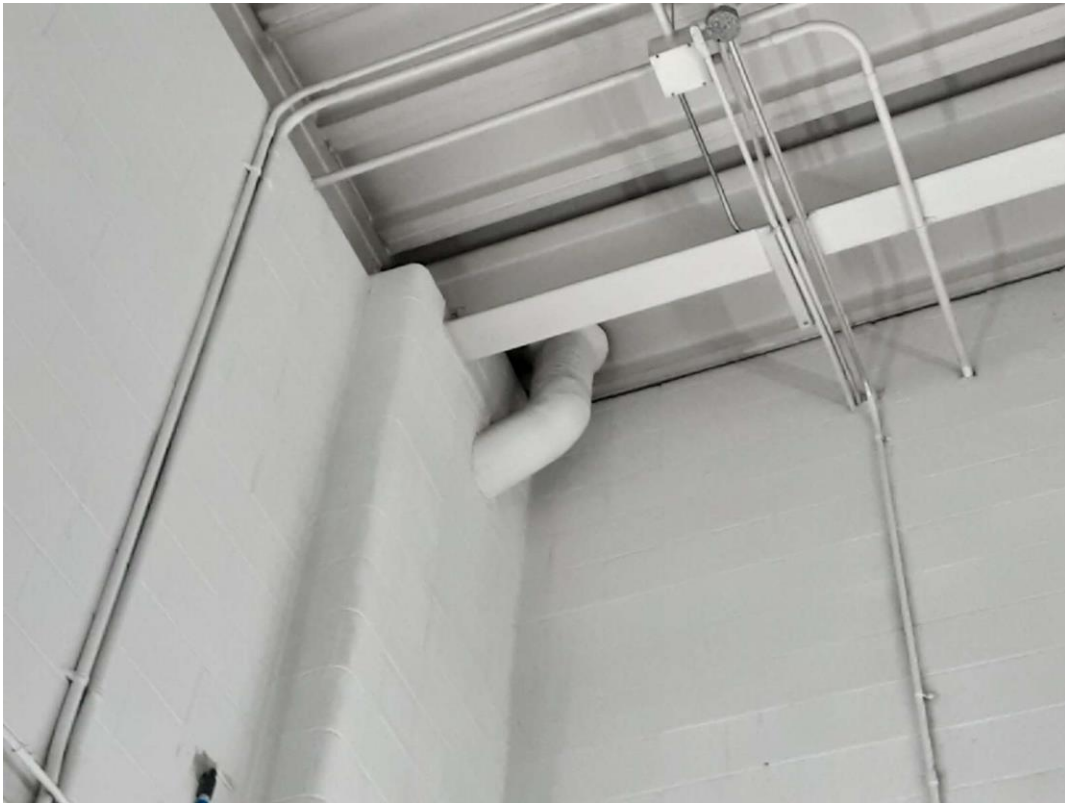
V0002 (Confirmed Asbestos), Piping, Rain Water Leader, Parging over Fibreglass, Chlorine Scale Room (Location #: 7)
