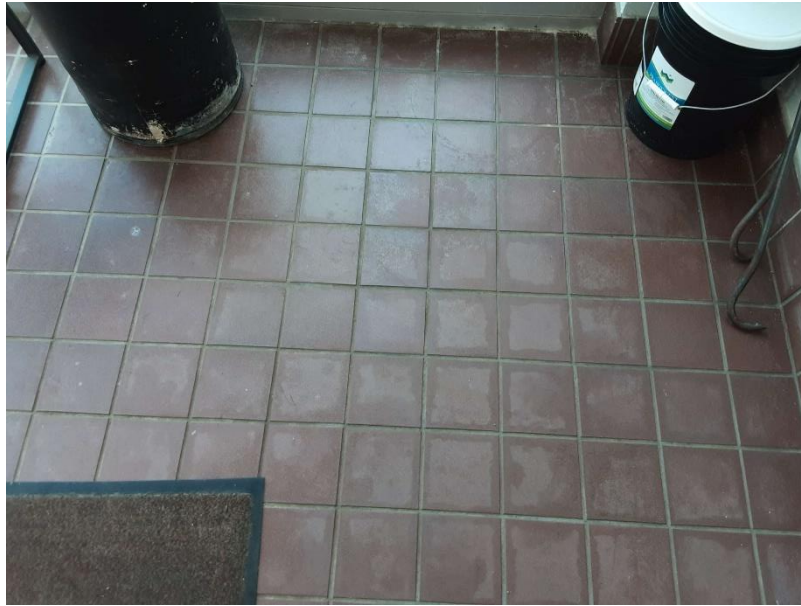
V9500 (Presumed Asbestos), Floor, All, Mortar, Main Building - Vestibule (Location #: 1) Setting compound
