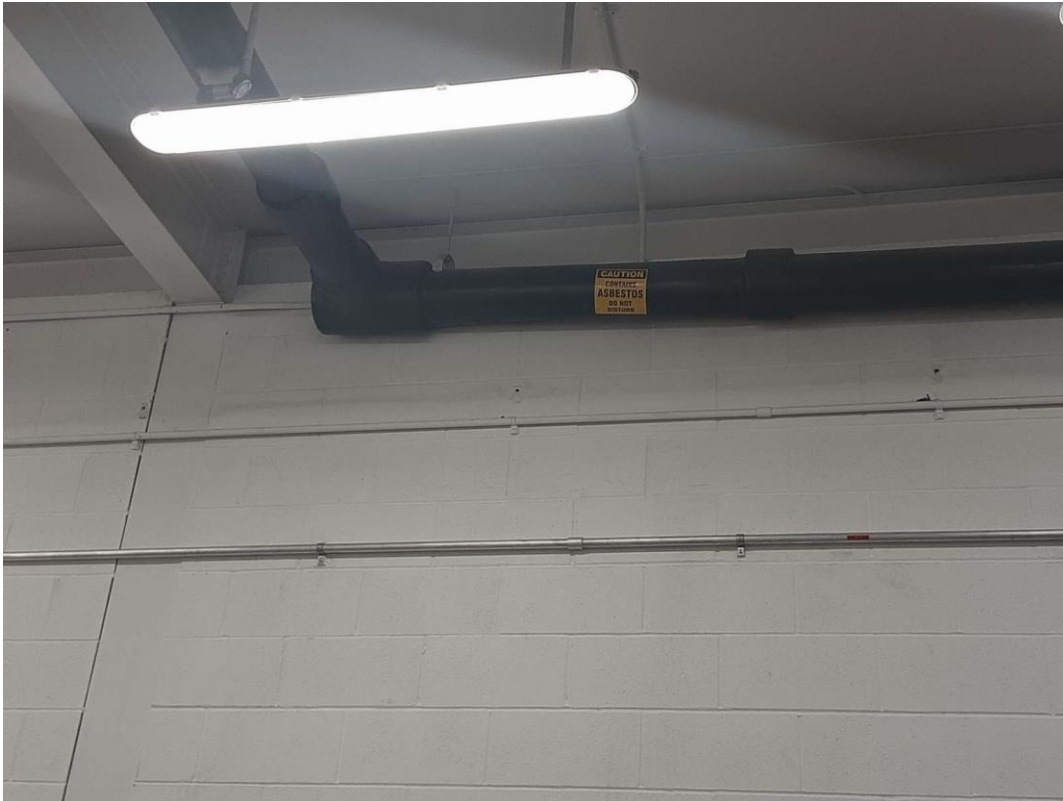
V0007 (Confirmed Asbestos), Piping, Rain Water Leader, Parging over Fibreglass, Chlorine Building - Chlorine Tonner Room (Location #: 8)
