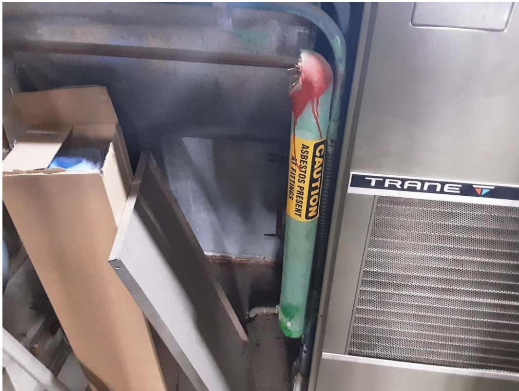
V0004 (Confirmed Asbestos), Damaged Piping, Domestic Water (Hot and Cold), Parging over Fibreglass, Old Pump Building - Furnace Room (Location #: 21)
