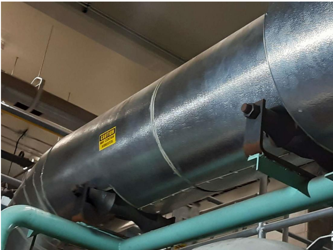
V0006 (Confirmed Asbestos), Duct, Exhaust, Magnesia block, Pump Floor (Location #: 19)
