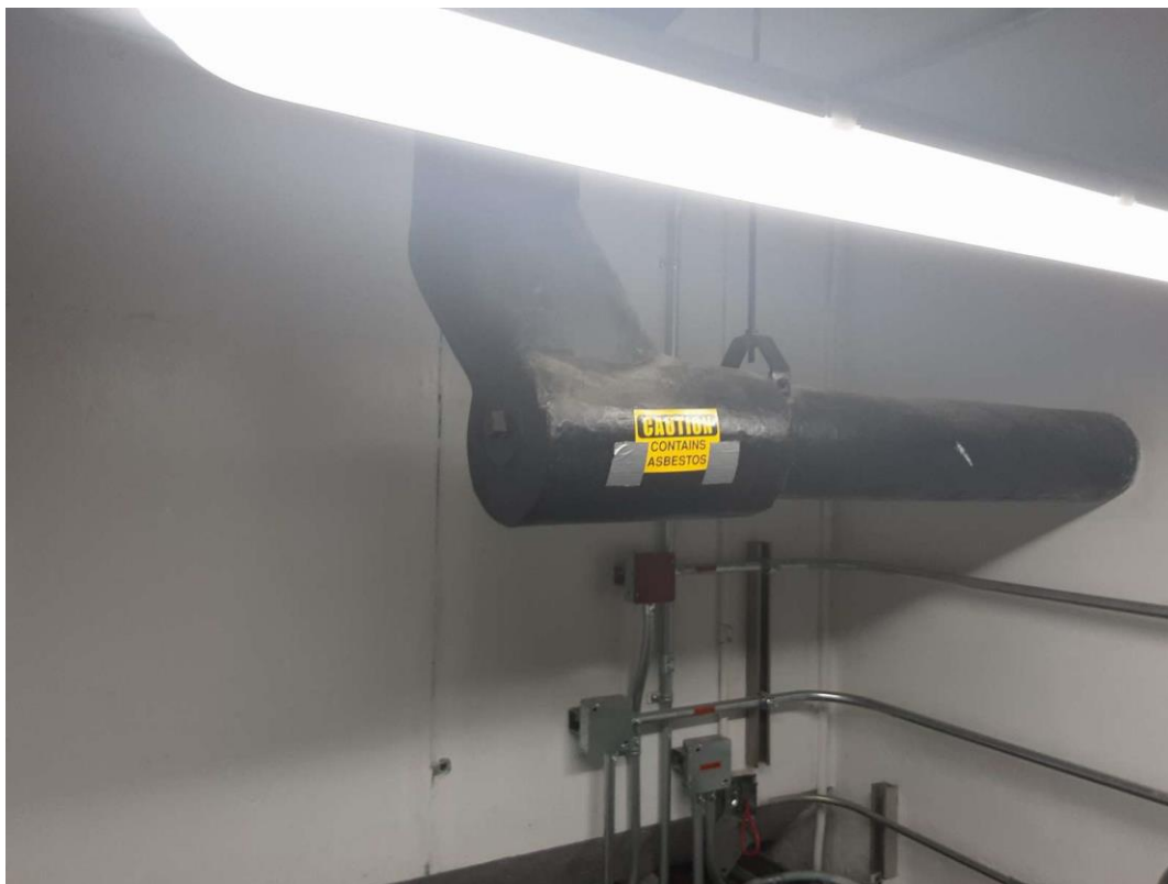
V0007 (Confirmed Asbestos), Piping, Rain Water Leader, Parging over Fibreglass, Chlorine Building - Stairwell (Location #: 11)
