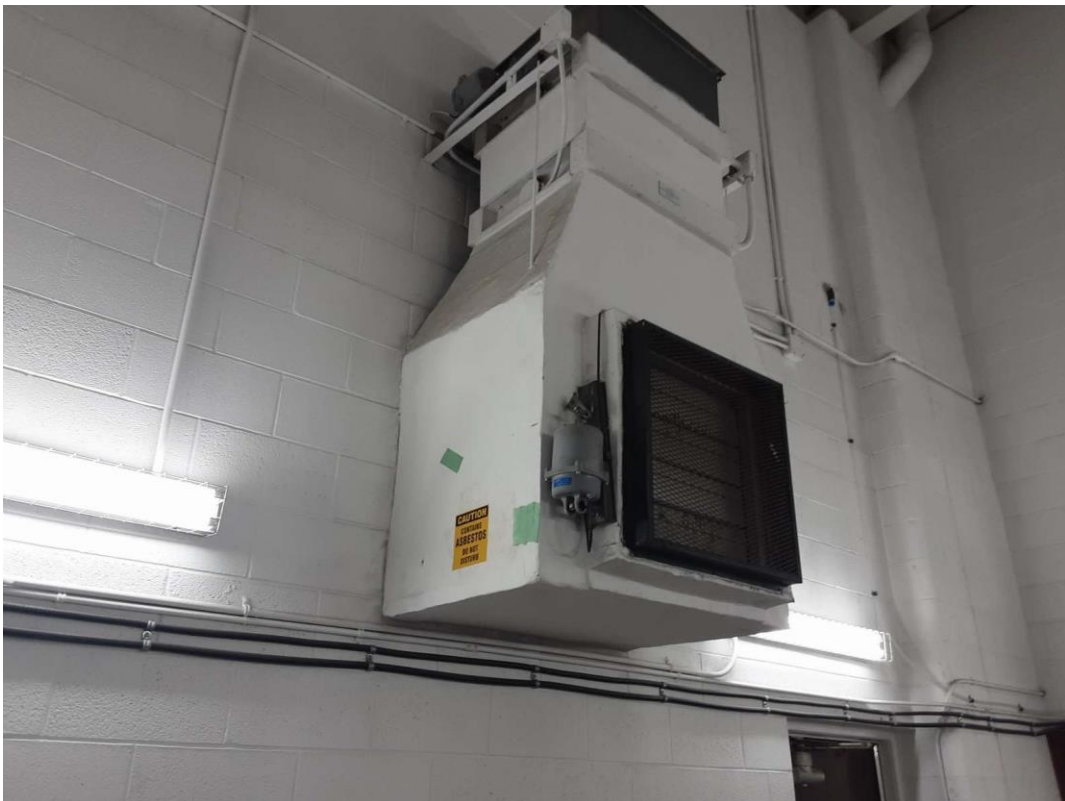
S0005 (Confirmed Asbestos), Duct, Fresh Air Intake, Fiberglass w/Parging, Chlorine Scale Room (Location #: 7)
