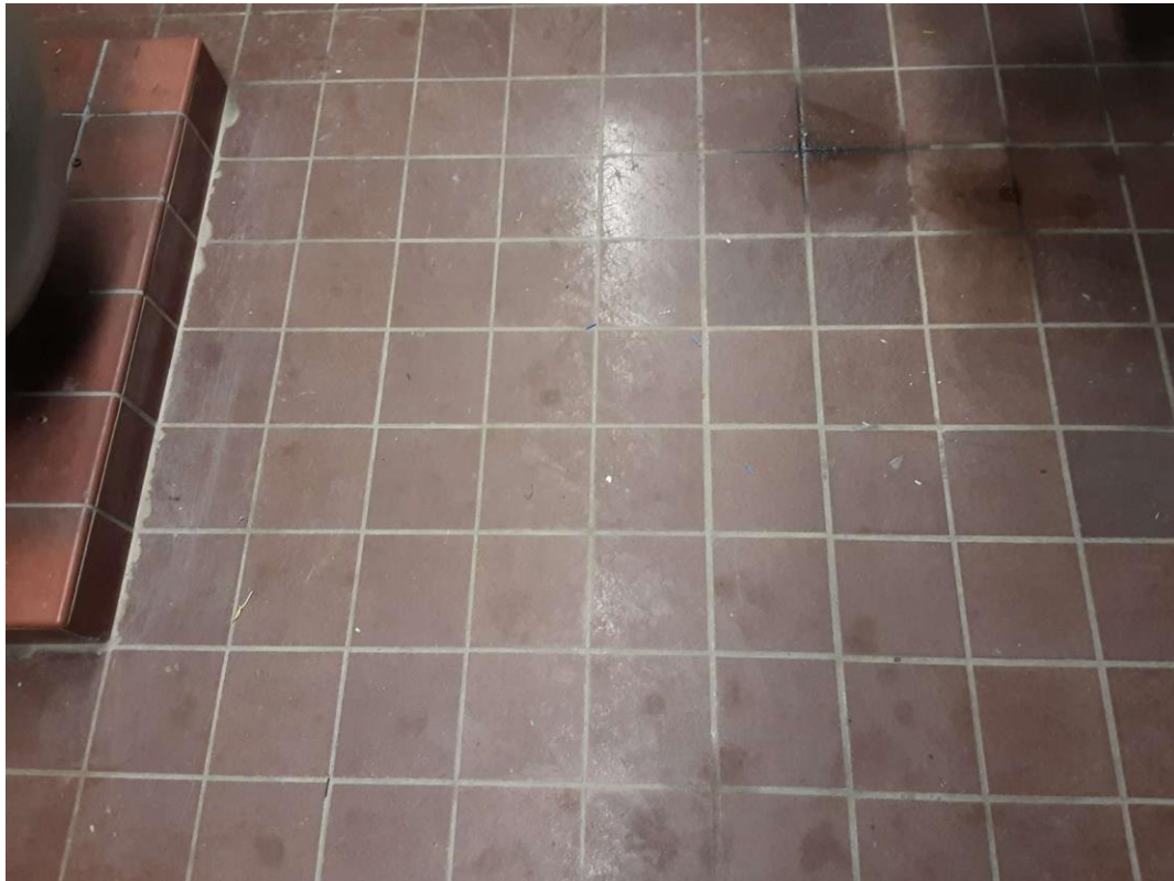
V9500 (Presumed Asbestos), Floor, All, Mortar, Main Building - Pump Room (Location #: 10) Setting compound
