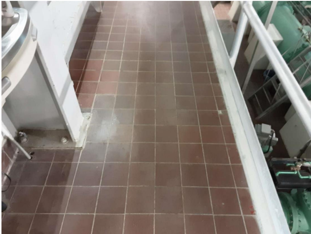
V9500 (Presumed Asbestos), Floor, All, Mortar, Main Building - Walkway (Location #: 4)
