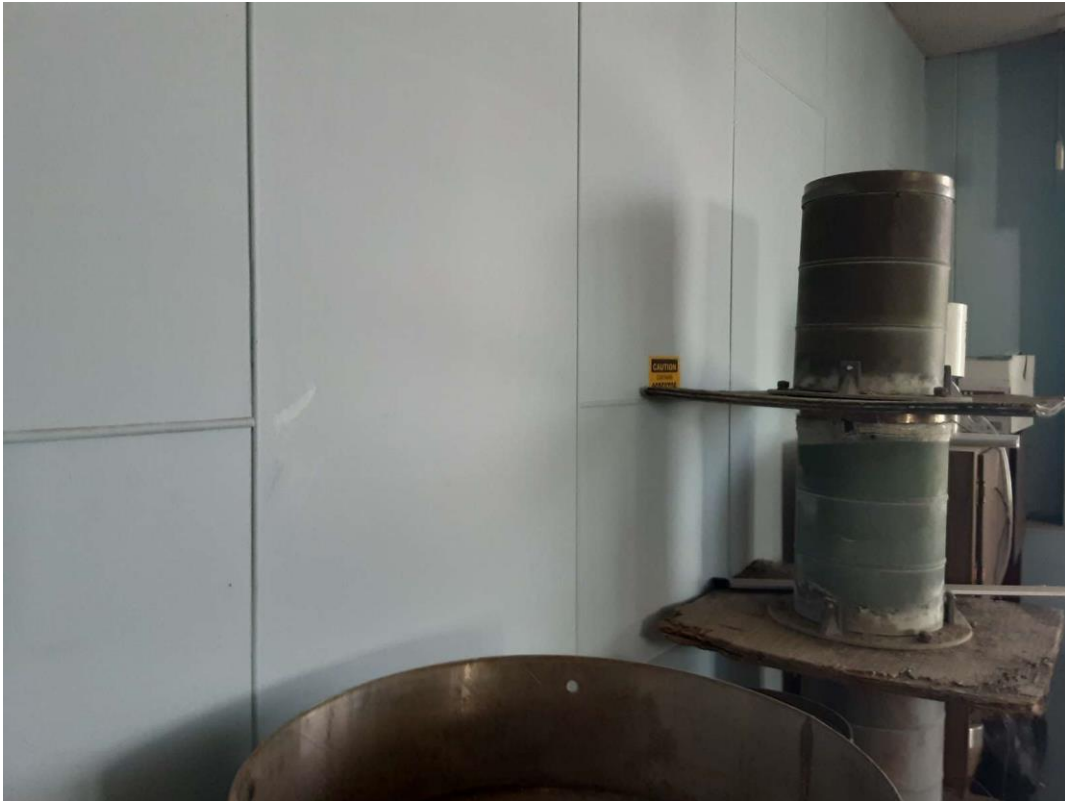
V9000 (Confirmed Asbestos), Wall, Cement Product, Old Pump Building - Dispatch (Location #: 13)
