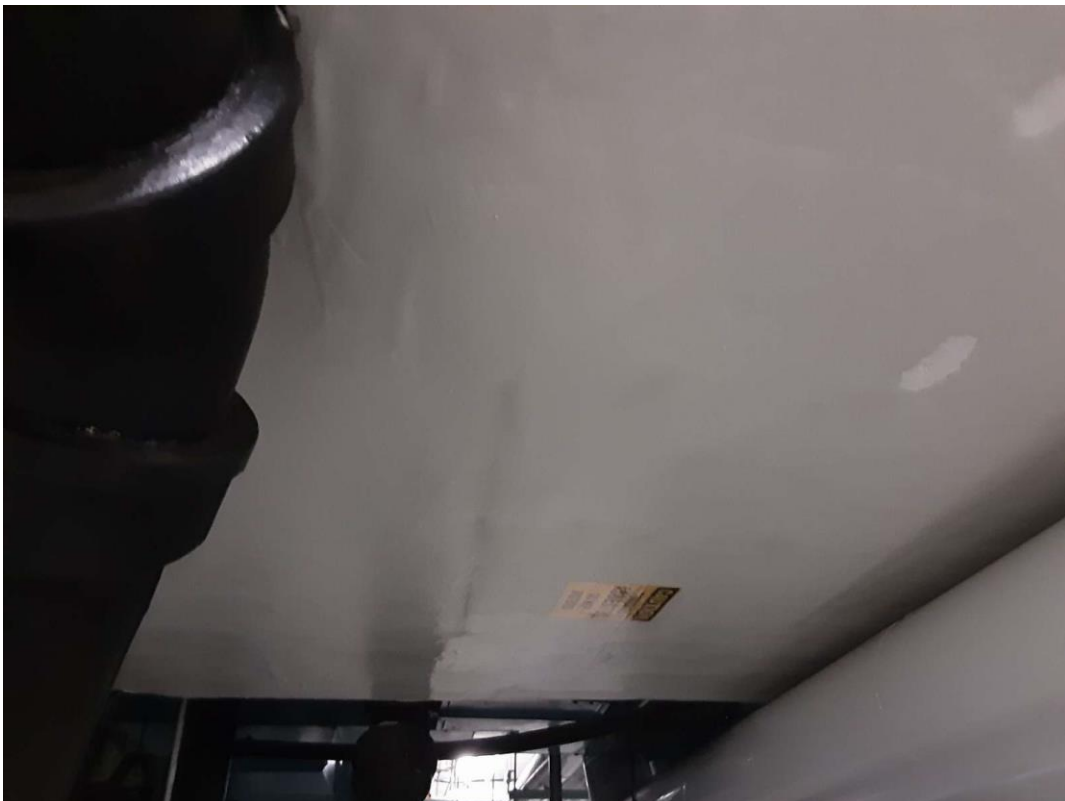
V0005 (Confirmed Asbestos), Duct, Fresh Air Intake, Fiberglass w/Parging, Fan Room (Location #: 16)
