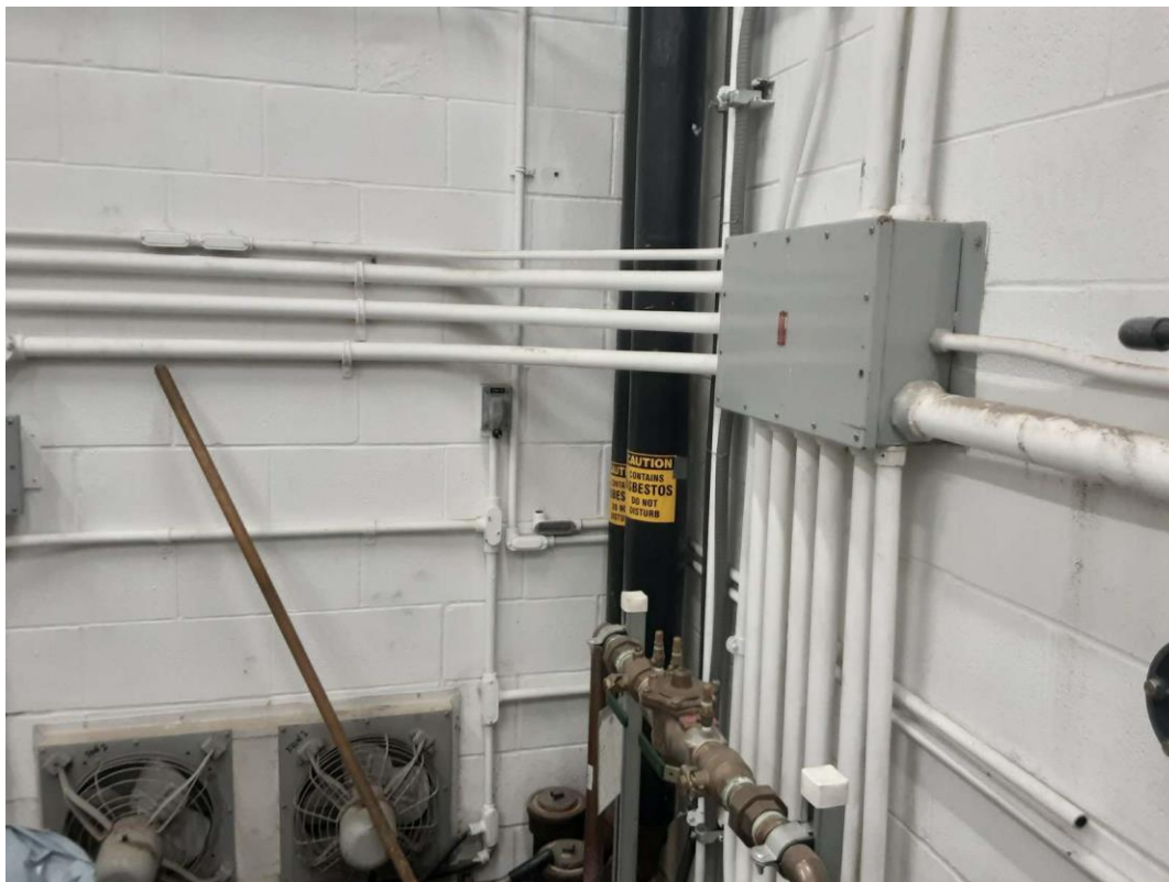
V0001 (Confirmed Asbestos), Piping, Rain Water Leader, Chlorine Building - Chlorinator Room (Location #: 9)
