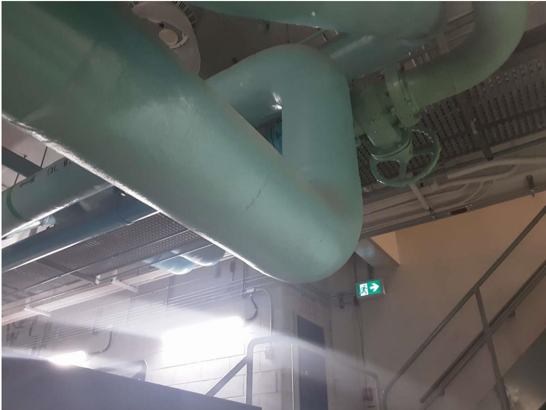
V0004 (Confirmed Asbestos), Piping, Chilled Water Return, Parging Cement, Pump Building - Basement (Location #: 1)
