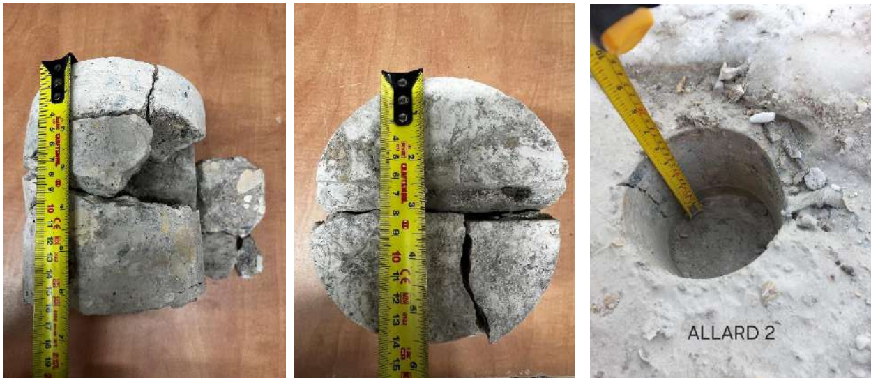
CH2 - Side of House # 502 St. Charles Street
