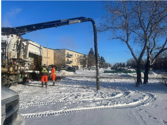
Photo 7: Soft digging with hydrovac at MW26-LM-02 on January 19
