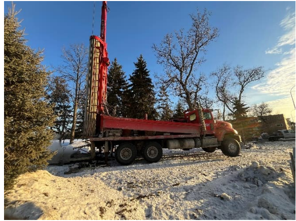
Photo 2: Drilling MW26-AM-02 at the Eastern (Zone 3) Site on January 14, 2026
