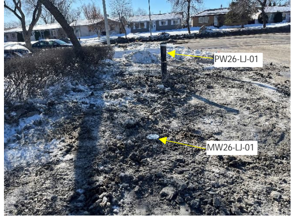
Photo 14: View of PW26-LJ-01 and MW26-LJ-01 (stick-up removed and flush-mount cover installed) at Western (Zone 1) Site on February 6, 2026.
