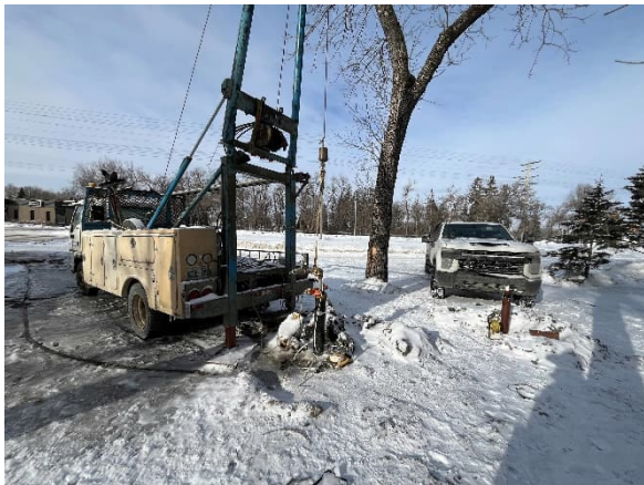
Photo 3: Pumping Test at Eastern (Zone 3) Site on January 16, 2026
