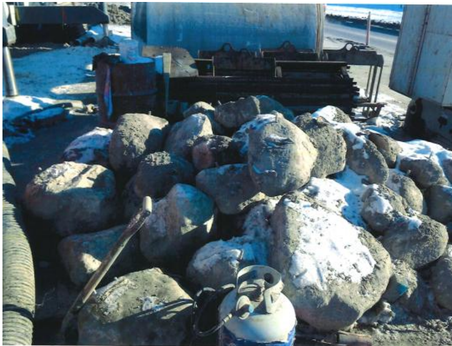
FIGURE 5-1: BOULDERS REMOVED DURING OPEN FACE TUNNELLING FOR THE NW INTERCEPTOR SEWER PROJECT (2015)
