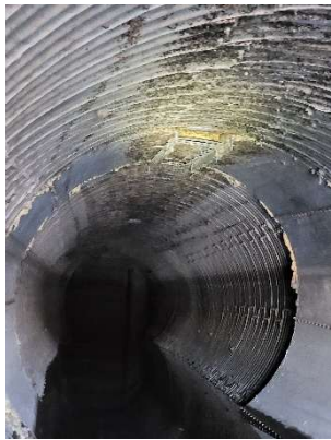
Photo 13: Roland Outfall – emergency repair/slip joint
