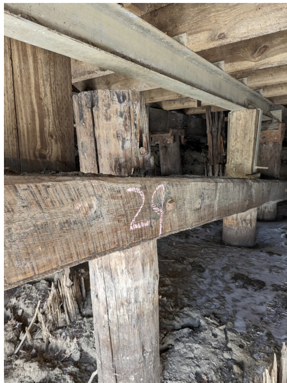
Photograph 28 Typical not bearing/not functional pile.
