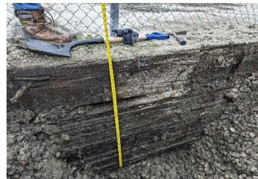
Figure 7: Rotten/split timber backwall
