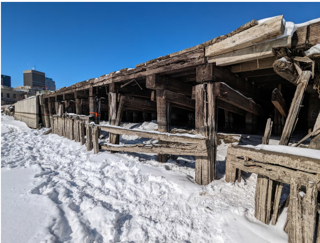
Photograph 20 South of firewall at North section. Note: Missing and deteriorated skirting throughout. Exterior piles deteriorated and not functional.
