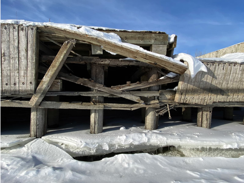
Photograph 17 Vertical face. Note: Severely deteriorated timber skirting and beams.
