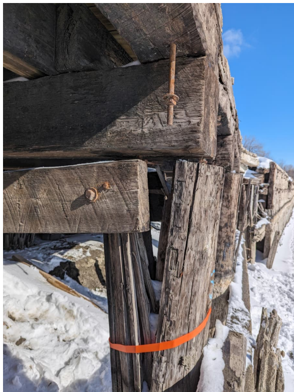
Photograph 24 Typical severely split and not functional pile.
