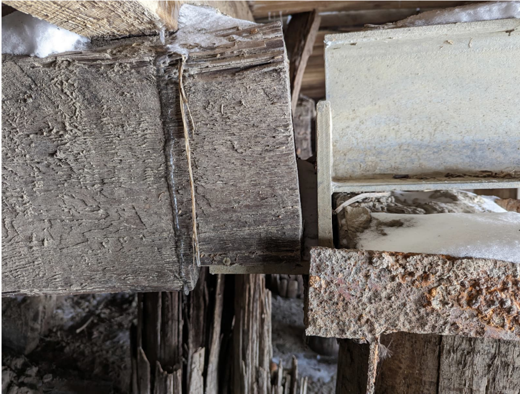
Photograph 33 Typical steel angle bearing at steel pile cap beam and timber pile cap.
