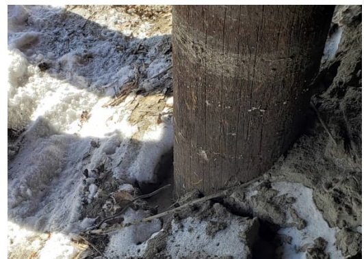
Figure 10: Gap around the piles
