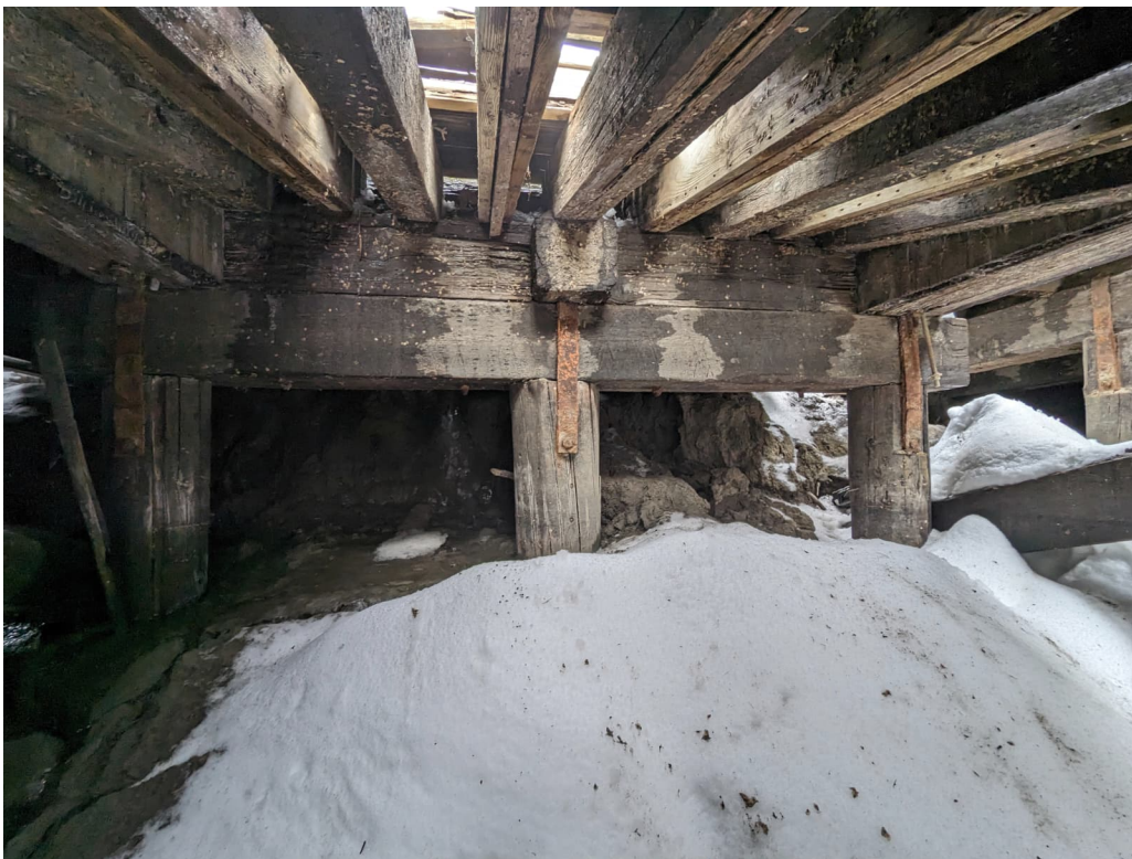
Photograph 34 Typical timber header construction below Slip No. 4.
