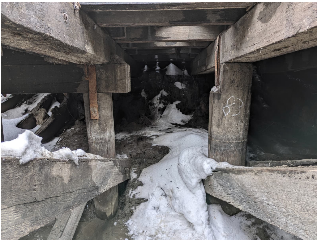
Photograph 38 Typical bay at enclosed North area. Note: Pile C buried due to riverbank height.
