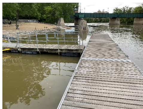
Figure 12: Typical floating dock at the Forks
