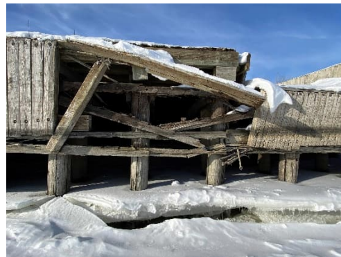
Figure 5: Typical broken and missing timber skirting
