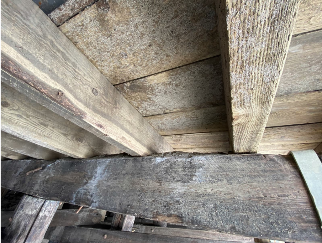
Photograph 21 Typical soffit and stringers.
