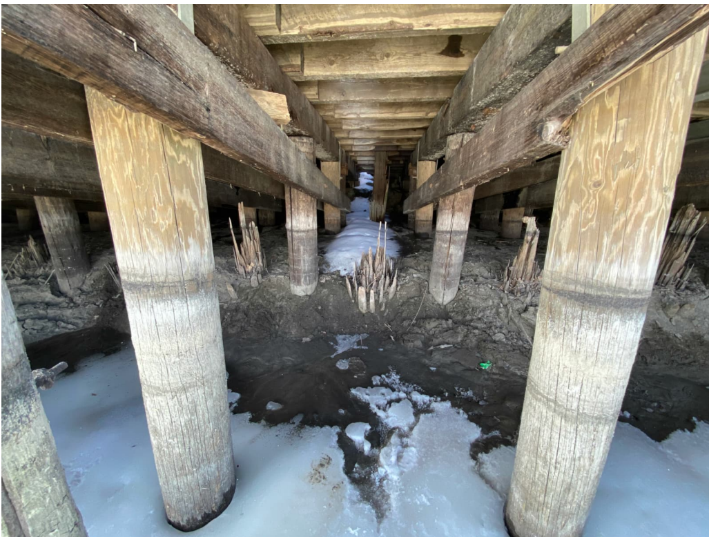
Photograph 22 Typical bay between pile rows. Note: Typical abandoned piles between Piles C and D.
