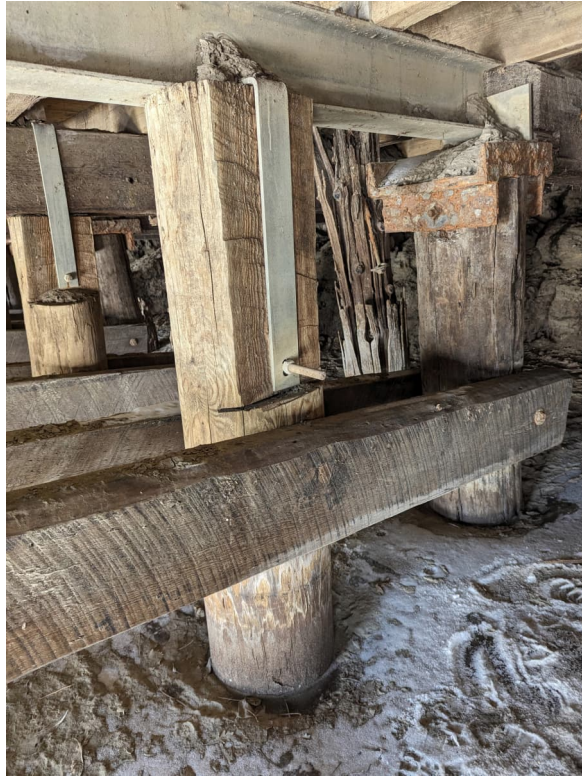
Photograph 29 Typical pile with section removed for connection.
