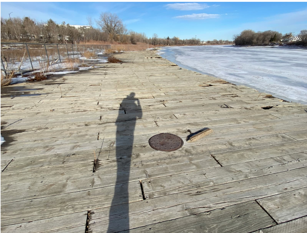
Photograph 12 Deck top. Note: Manhole cover for access.
