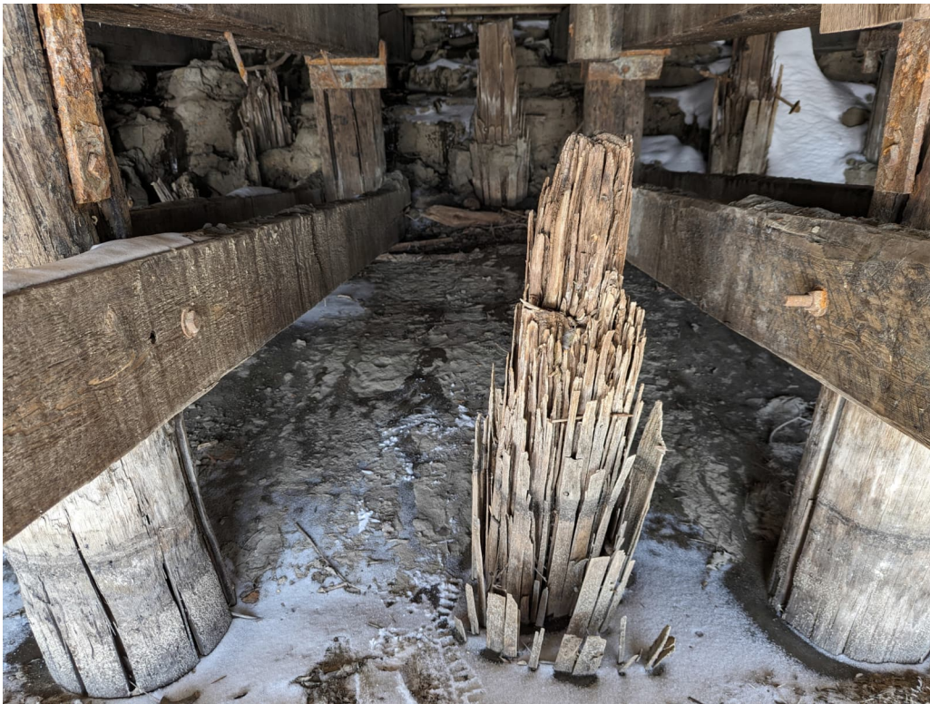
Photograph 26 Typical abandoned pile between existing piles.
