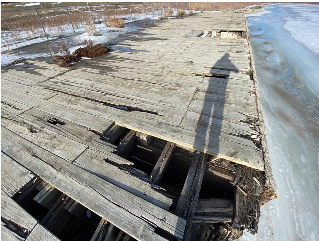
Photograph 14 Deck top. Note: Typical deteriorated planks and stringers with holes in deck.
