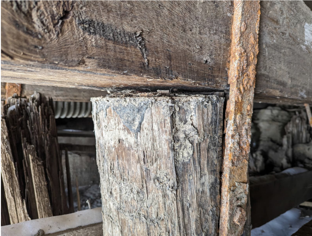
Photograph 27 Typical partailly bearing pile.
