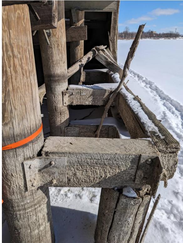
Photograph 23 Typical beam construction at Rows 35 to 46.
