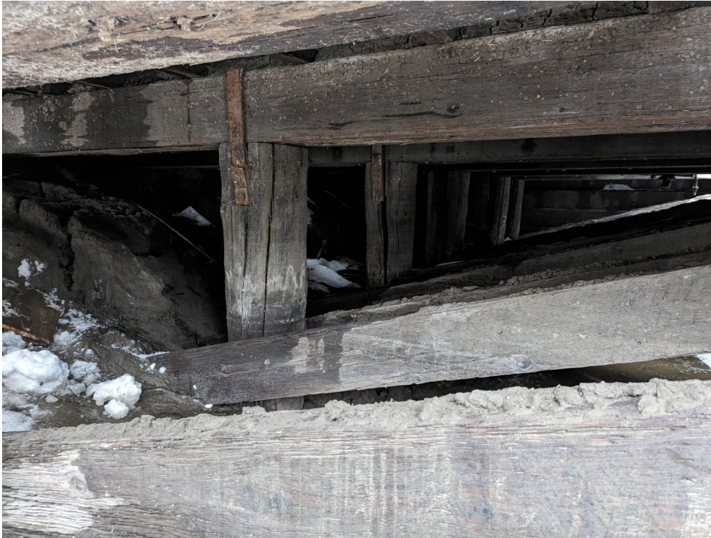
Photograph 37 Looking into enclosed North area. Note: Typical split piles.
