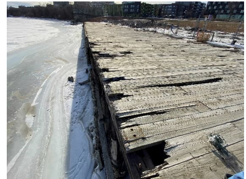
Figure 2: Typical deteriorated timber deck planks
