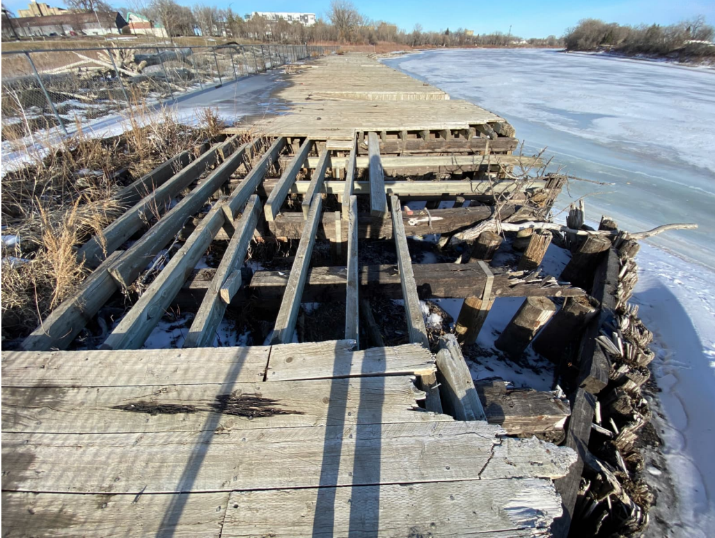
Photograph 11 Deck top. Note: Deck planks removed.
