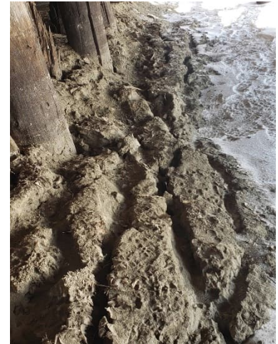
Figure 9: Erosion between Pile D1 and E
