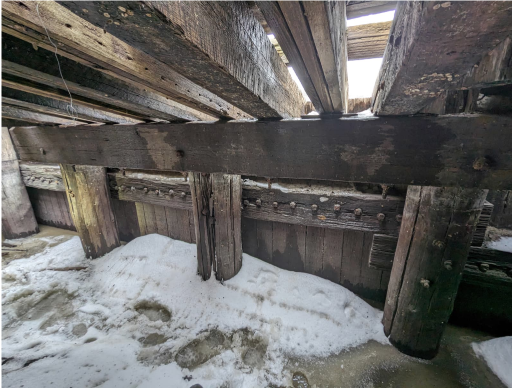
Photograph 35 Typical timber header construction below Slip No. 4.
