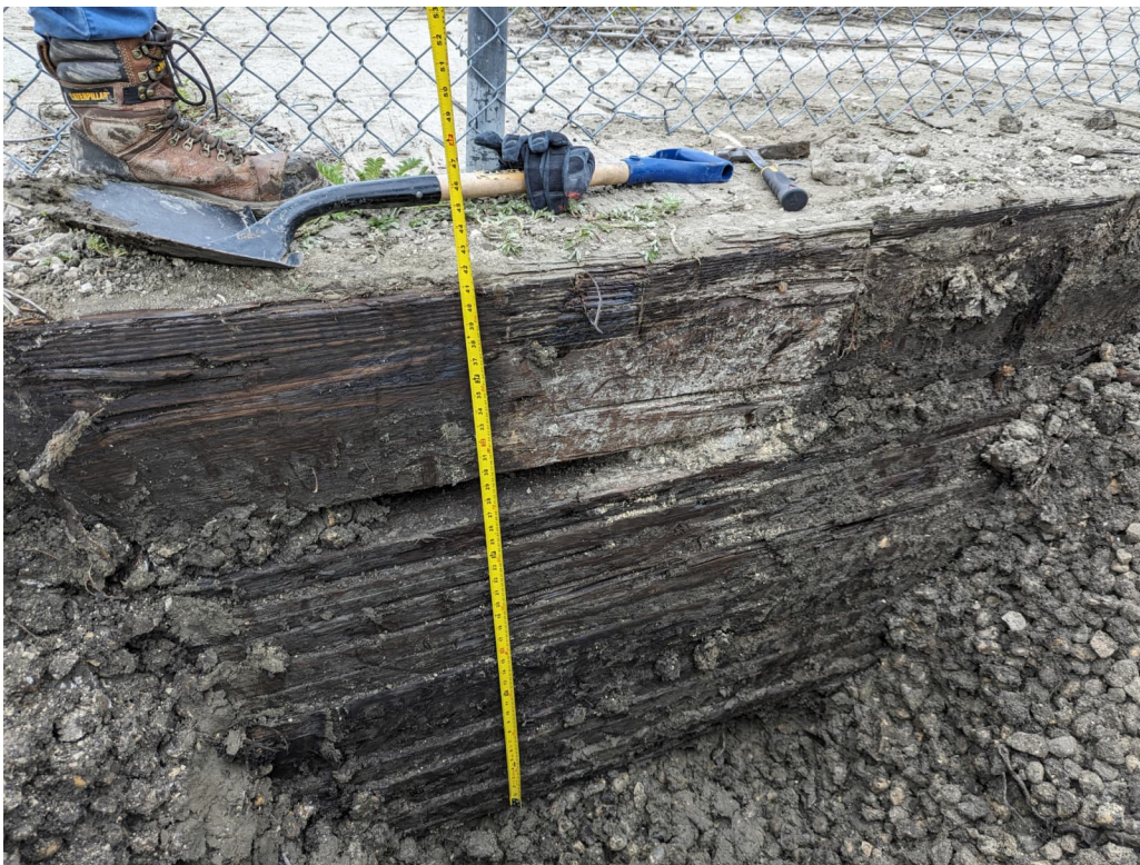
Photograph 40 Timber backwall at test pit excavation. Note: Typical rotten/split members.
