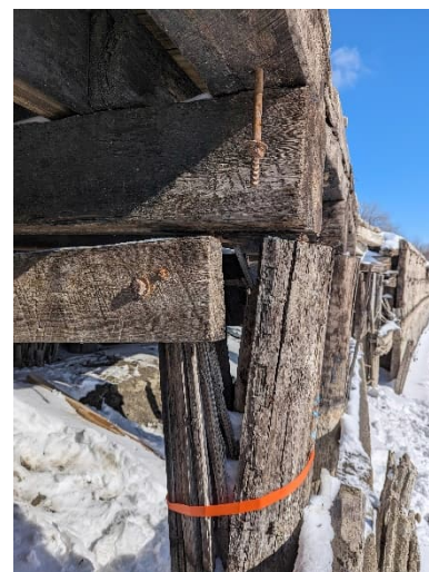
Figure 3: Deteriorated timber pile with minimal bearing (Pile E shown)
