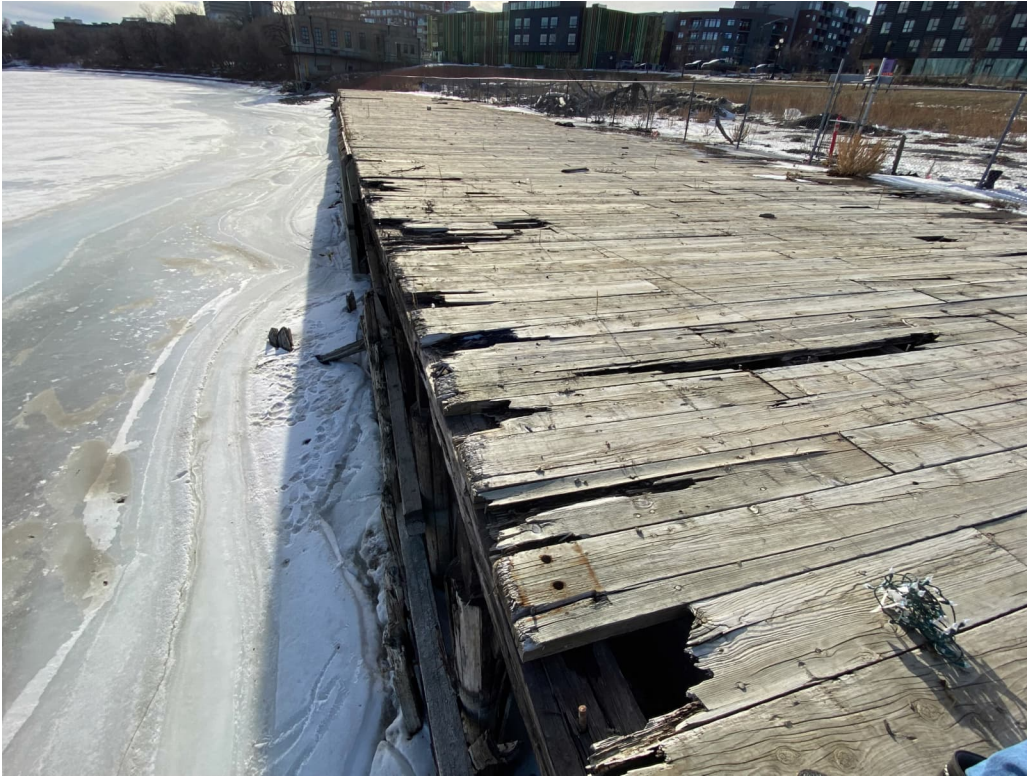
Photograph 13 Deck top. Note: Typical deteriorated planks with holes in deck.
