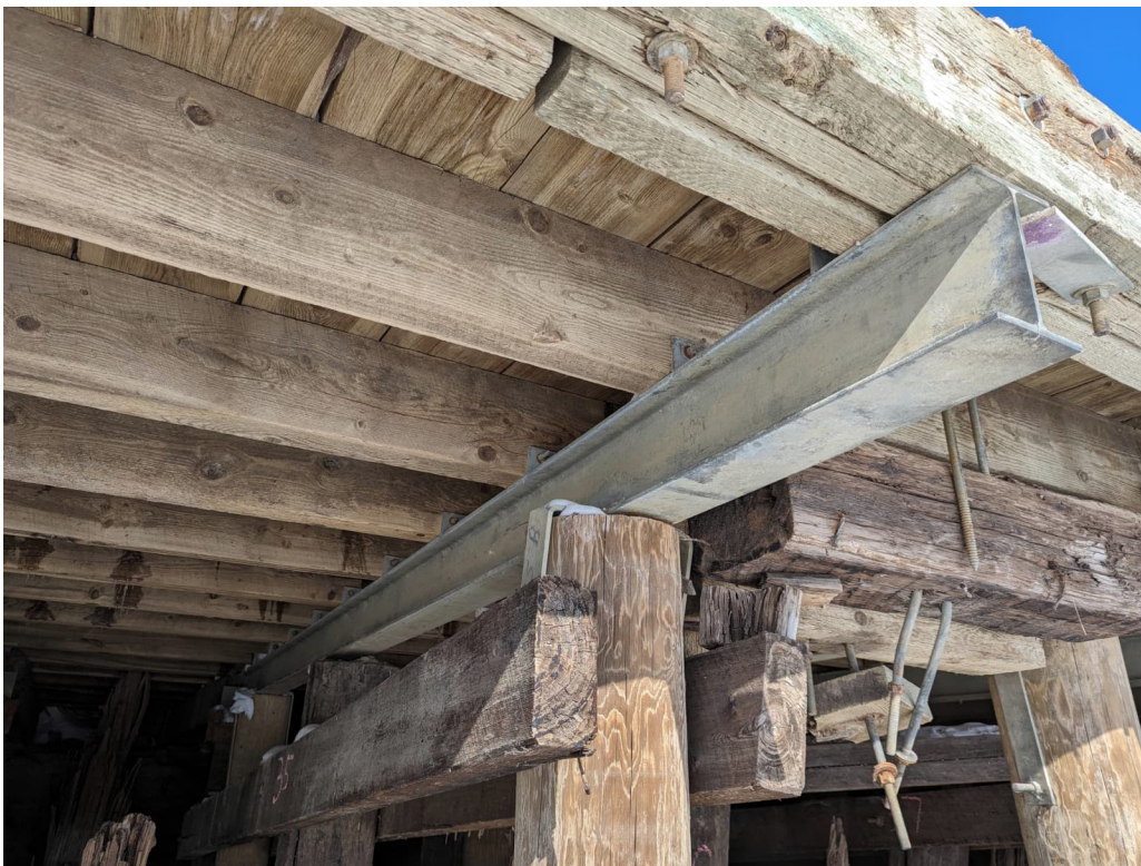
Photograph 32 Typical steel pile cap beam.
