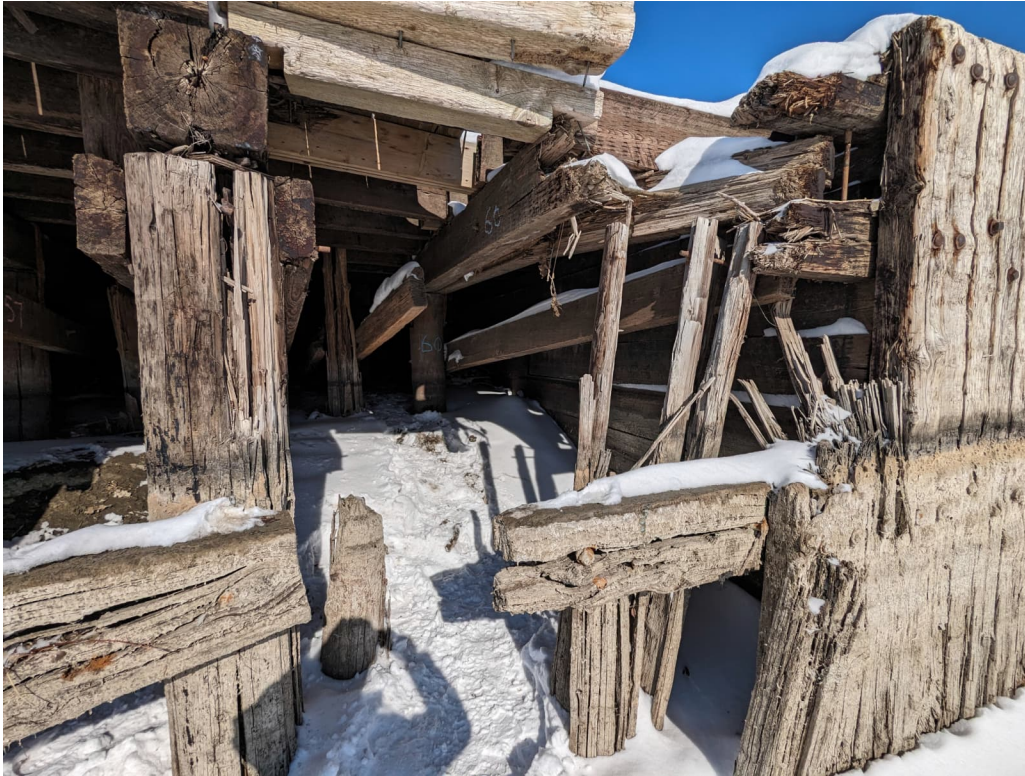
Photograph 19 Firewall separating North and centre section of structure.
