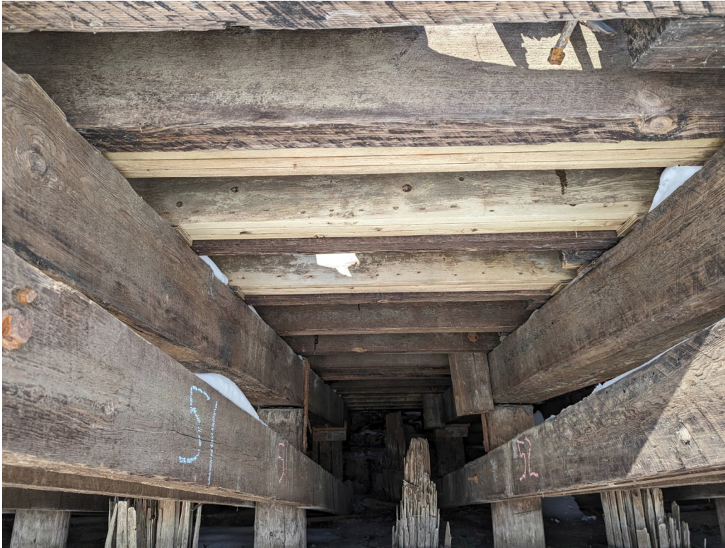
Photograph 31 Showing stringers with fire damage paired with newer built-up stringers.
