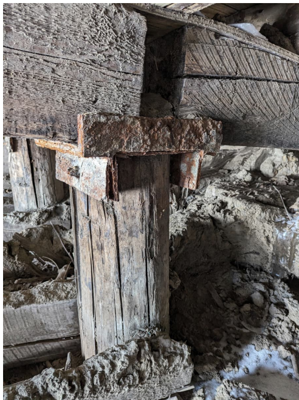
Photograph 30 Typical steel shoe at Pile C. Note: Severe corrosion throughout.
