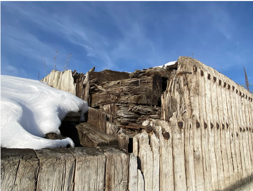
Photograph 18 Slip No. 1. Note: Severely deteriorated timbers.
