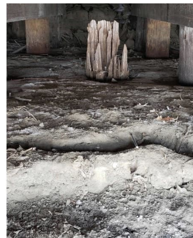
Figure 8: Erosion underside the dock
