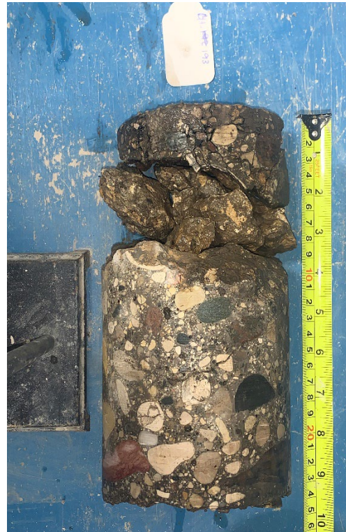
Figure 2 – Core Sample No. 193 – Aikins St
