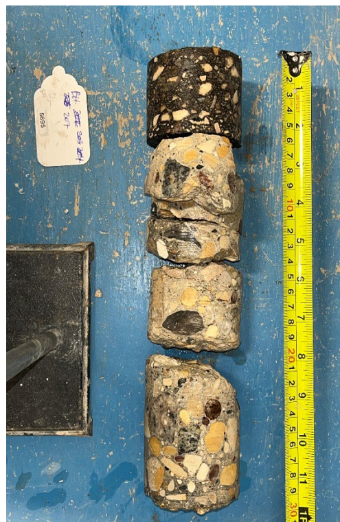
Figure 16 – Core Sample No. 207 – Mountain Ave
