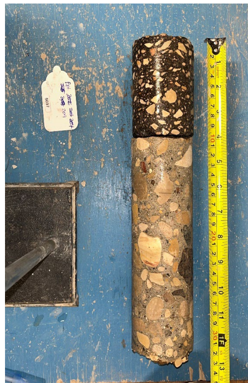
Figure 18 – Core Sample No. 209 – Mountain Ave
