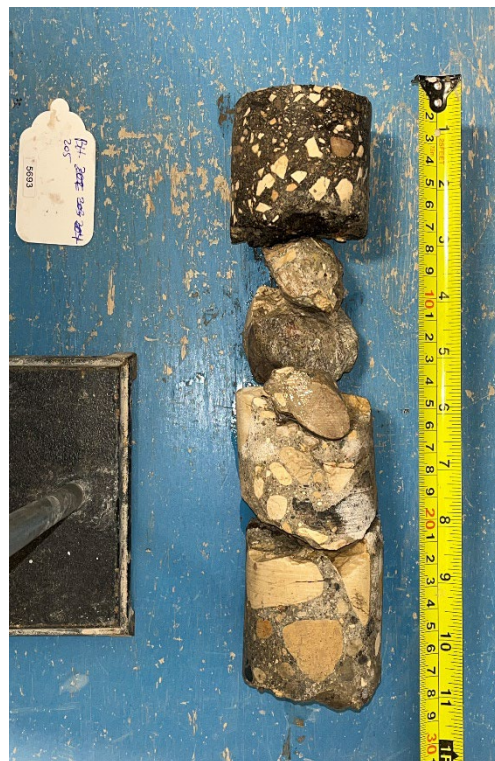
Figure 14 – Core Sample No. 205 – Mountain Ave
