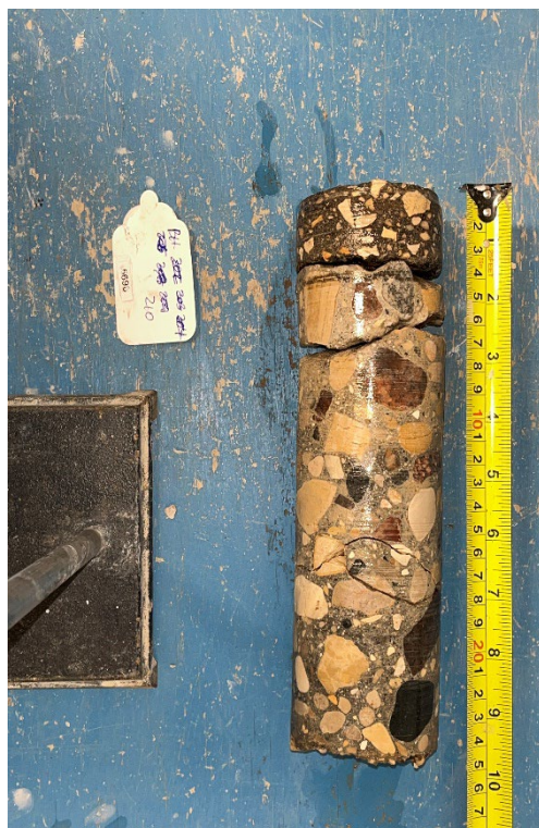
Figure 19 – Core Sample No. 210 – Mountain Ave
