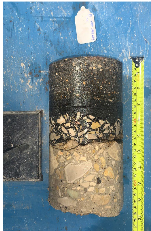
Figure 4 – Core Sample No. 195 – Robinson St
