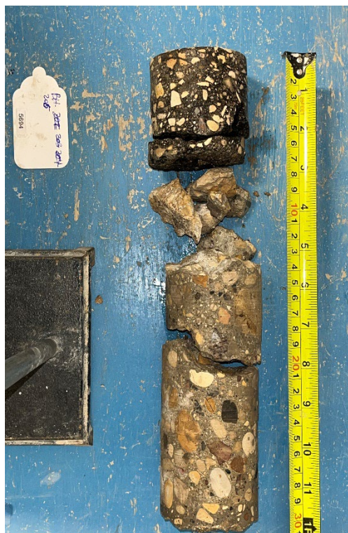
Figure 15 – Core Sample No. 206 – Mountain Ave
