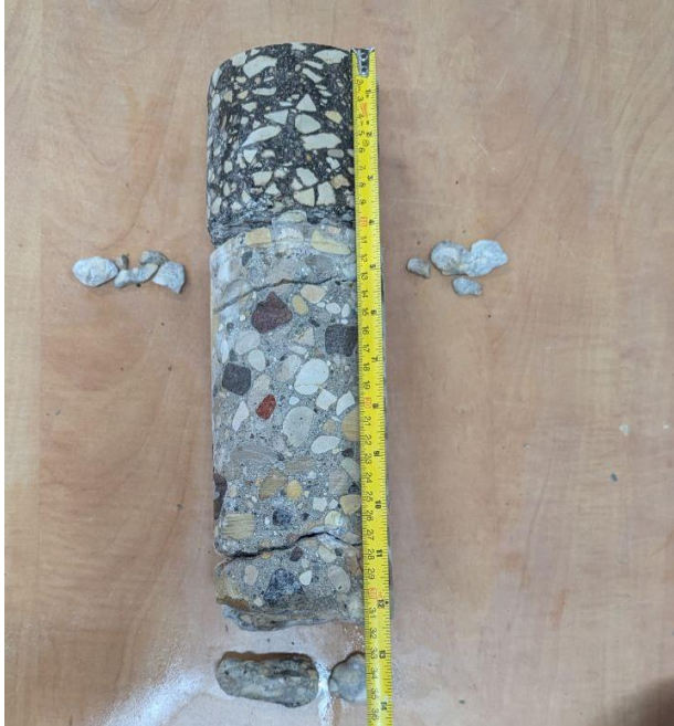
, Core 1 (Asphalt Thk 90mm, Concrete Thk 240mm)
