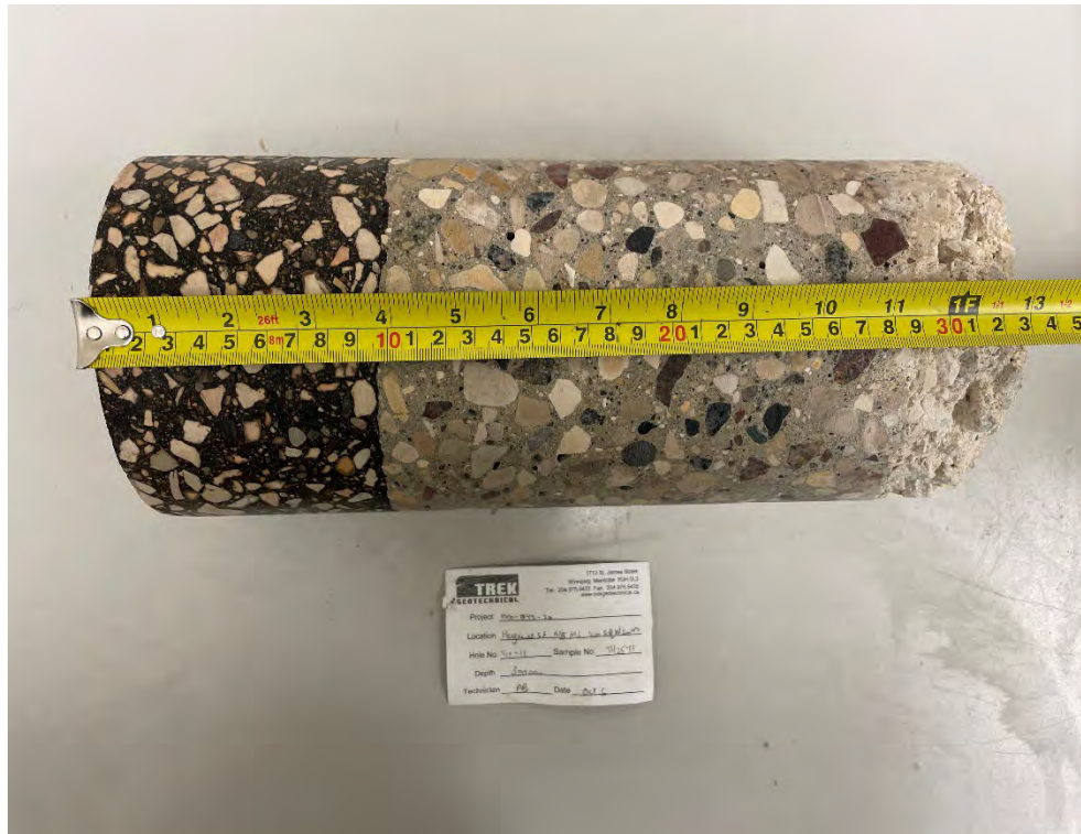
Photo 3: Pavement Core Sample at TH25-11
