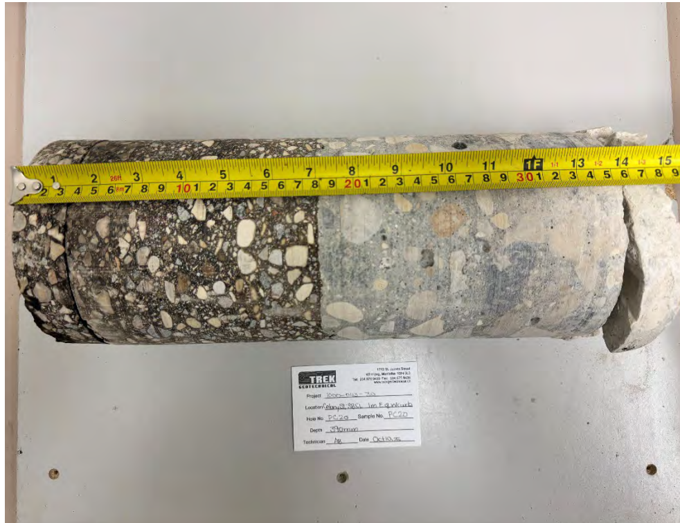
Photo 1: Pavement Core Sample at PC25-20
