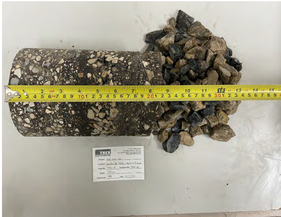
Photo 3: Pavement Core Sample at TH25-14
