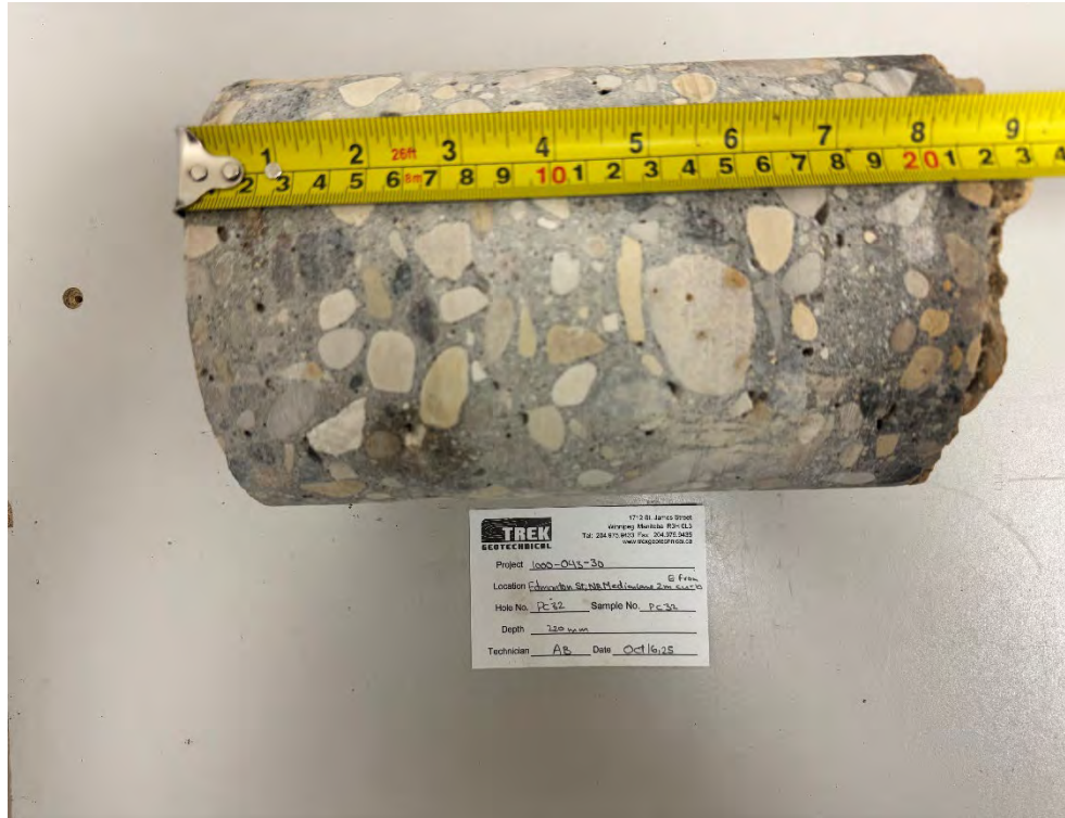
Photo 3: Pavement Core Sample at PC25-32
