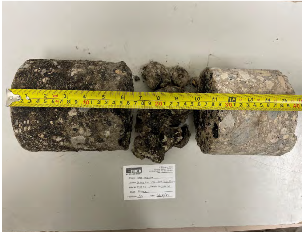
Photo 3: Pavement Core Sample at TH25-32
