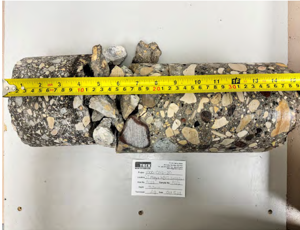
Photo 3: Pavement Core Sample at PC25-23
