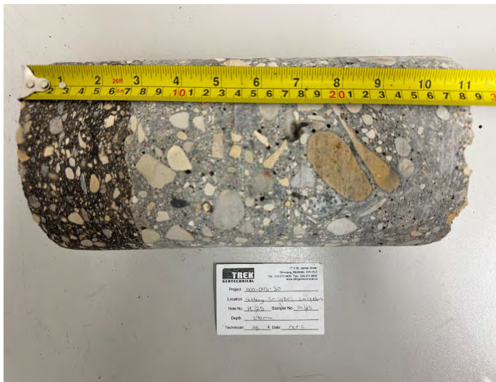
Photo 4: Pavement Core Sample at PC25-25
