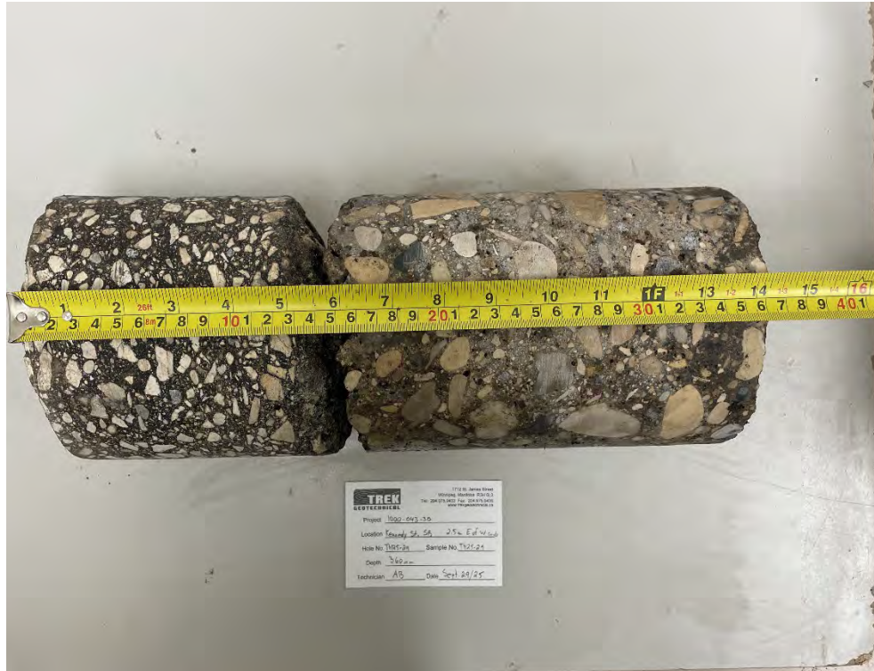
Photo 7: Pavement Core Sample at TH25-29
