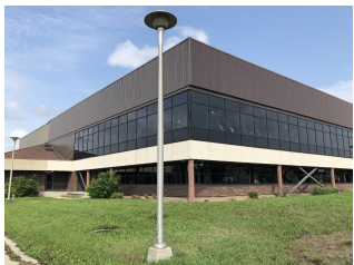
Existing Path Lighting
