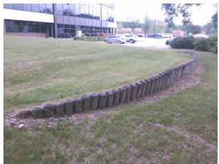
Existing Log Retaining Wall
