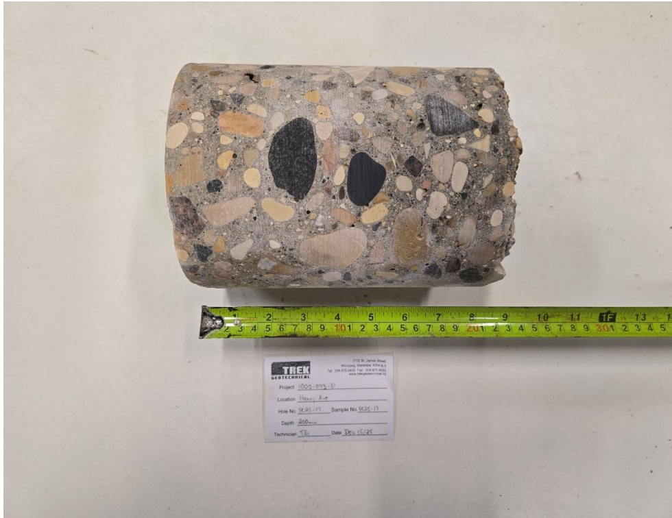
Photo 3: Pavement Core Sample at PC25-17
