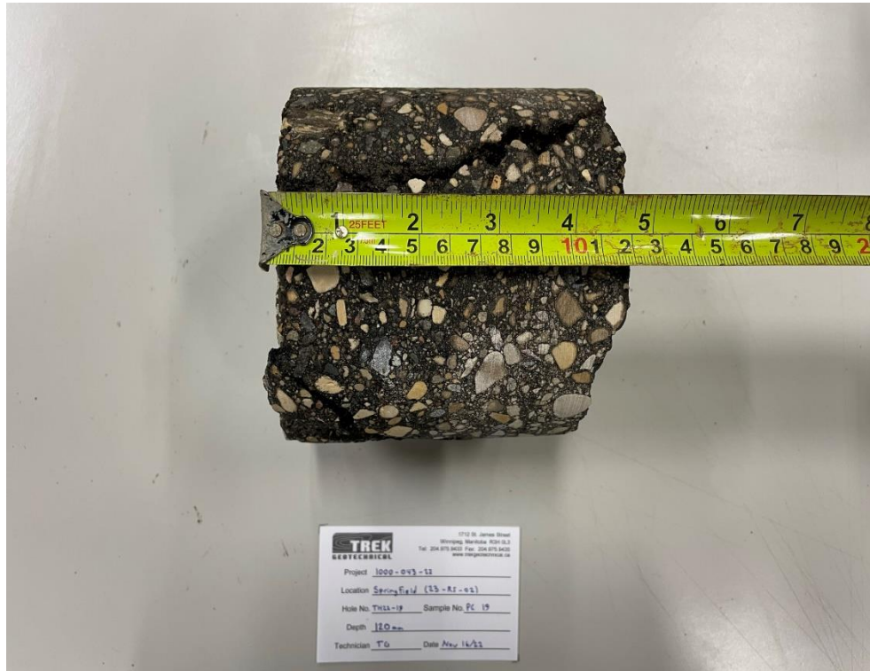
Photo 3: Pavement Core Sample at TH22-19
