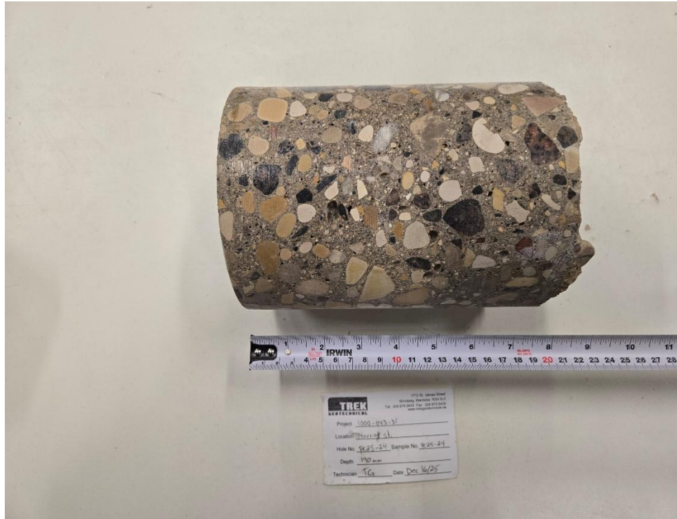
Photo 3: Pavement Core Sample at PC25-24
