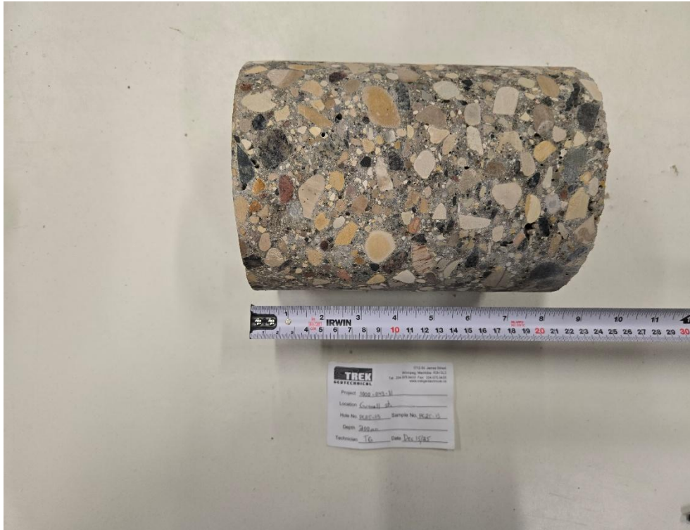
Photo 3: Pavement Core Sample at PC25-13
