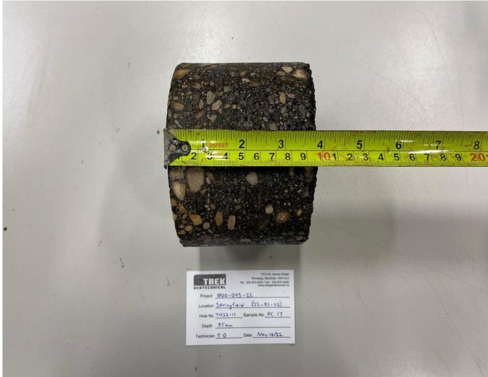
Photo 1: Pavement Core Sample at TH22-17
