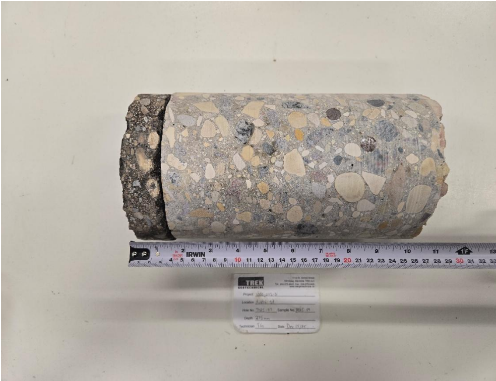
Photo 3: Pavement Core Sample at TH25-07
