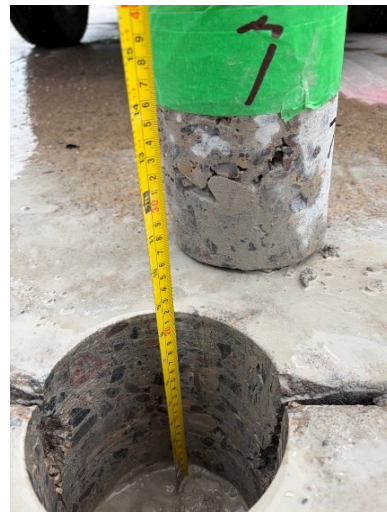
Core 7 - Site Photo
