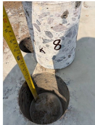
Core 8 - Site Photo
