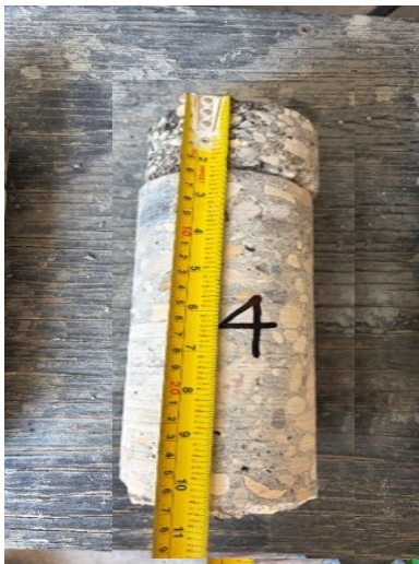
Core 4 - Mid Slab
