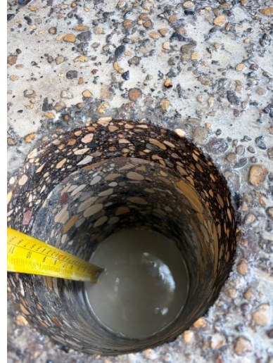
Core 5 - Site Photo
