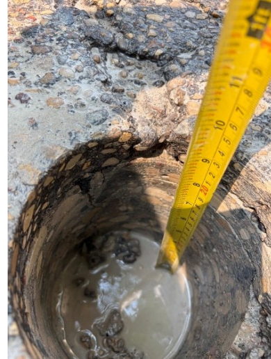
Core 3 - Site Photo
