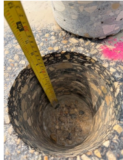
Core 11 - Site Photo
