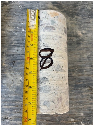
Core 8 - Mid Slab
