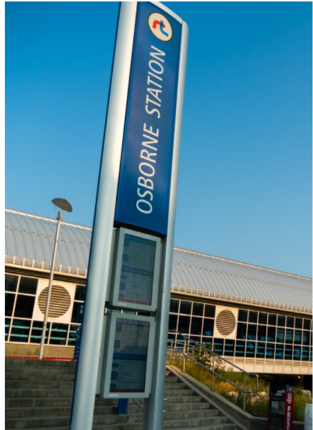
The Osborne Station is a transit hub along the City of Winnipeg's Rapid Transit line. Photo credit: Nathaniel Magbanua.
