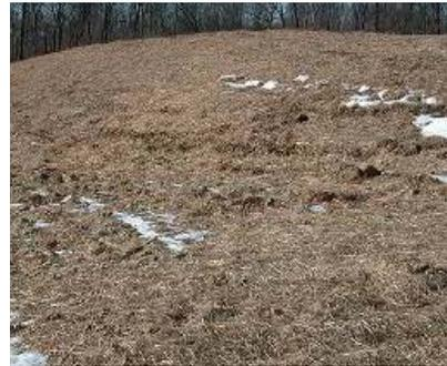
Hydroseeding is a process used to provide a temporary cover and aid revegetation through the spray application of a blended mix of seed, water, fertilizer and mulch.
