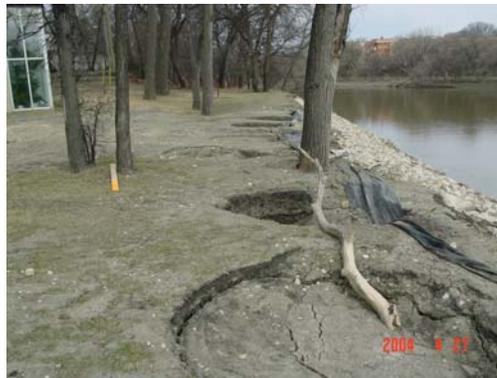
Sediment fence, while intercepting sediment from surface runoff, does little to address larger erosion problems.
