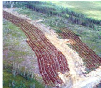
Scarification can be a useful initial sediment control technique when it is used as part of a set of practices. On winter slopes during the construction phase, for example, slope scarification is an easy way to help reduce the risk of sediment moving during short melt periods that may occur while construction is underway.
