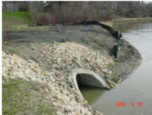
Sediment fence used below exposed soil at a culvert outfall.
