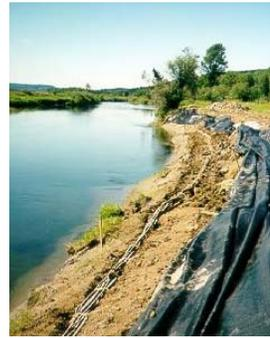
Bioengineering can be used to provide vegetative cover in areas where planting and seeding is not possible. It is a technique that will require initial erosion control measures such as seeding and mulching vegetation grows.
