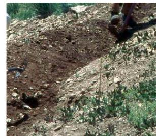
Very little maintenance is required when water-bars are properly constructed and placed in the right locations. Water bars can be constructed of compacted soil, gravel, rocks, or logs partially buried into the road or trail bed, placed at a 30° angle across the right-of-way. The material chosen should be durable enough to withstand expected traffic.
