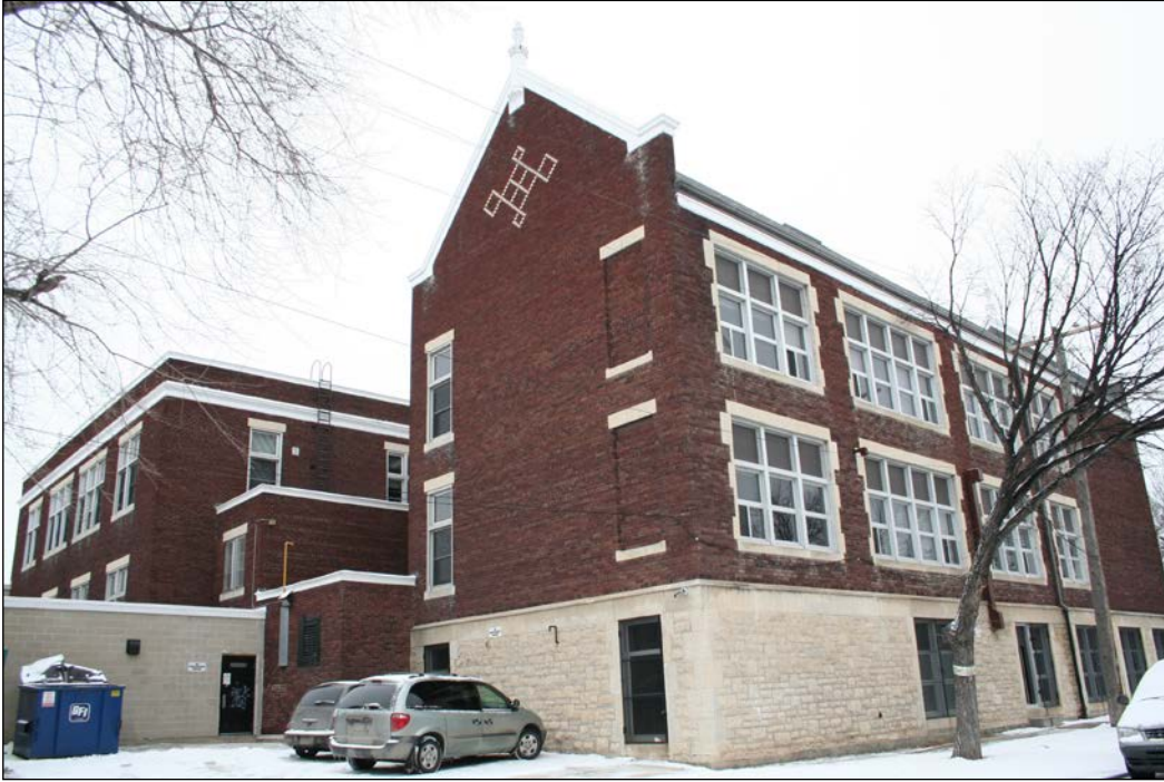
Rear (west) and south façades, 2009
