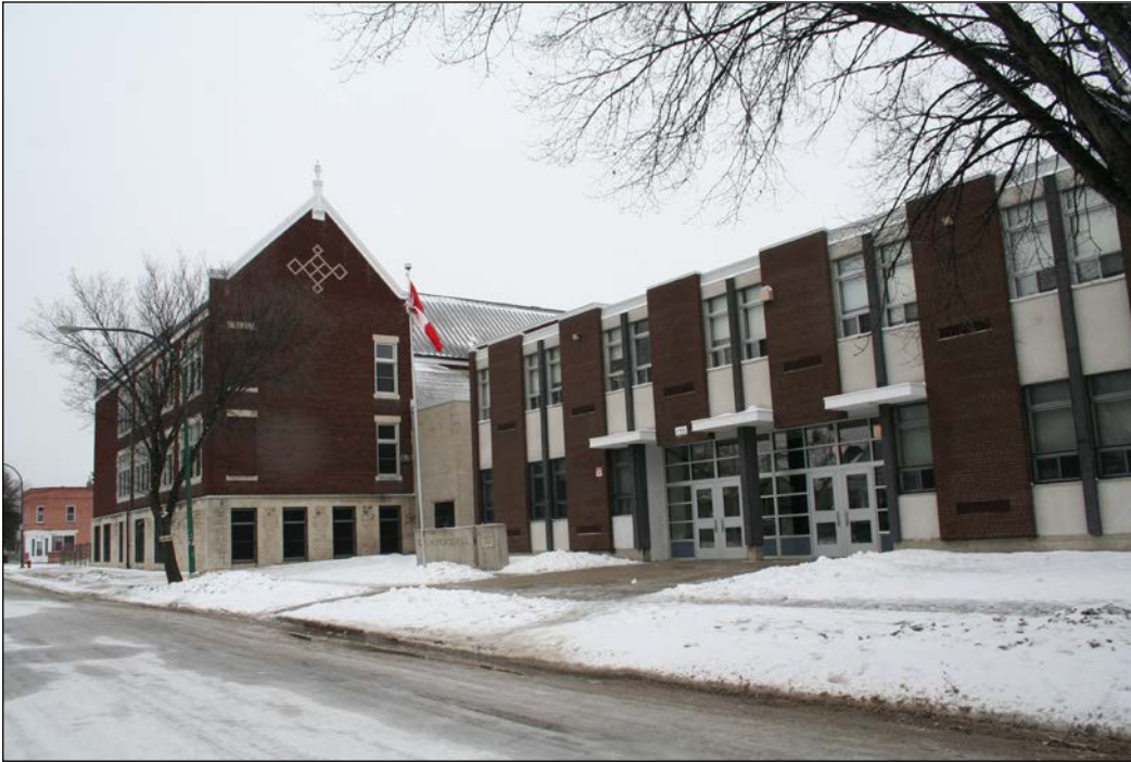
Rear (west) and north façades, 2009
