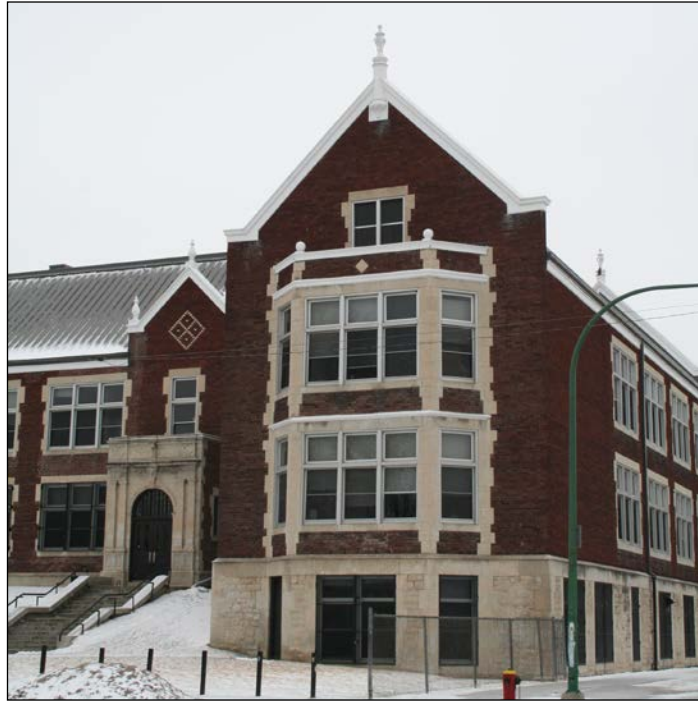
Northeast corner detail, 2009
