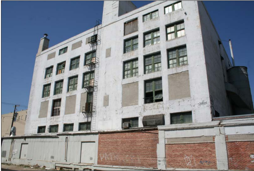
Rear (north) and east façades, 2006
