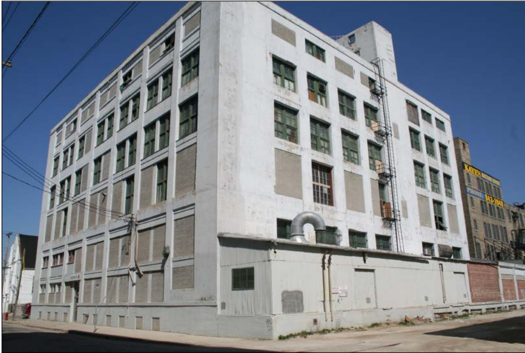
Front (south) and east façades, 2006
