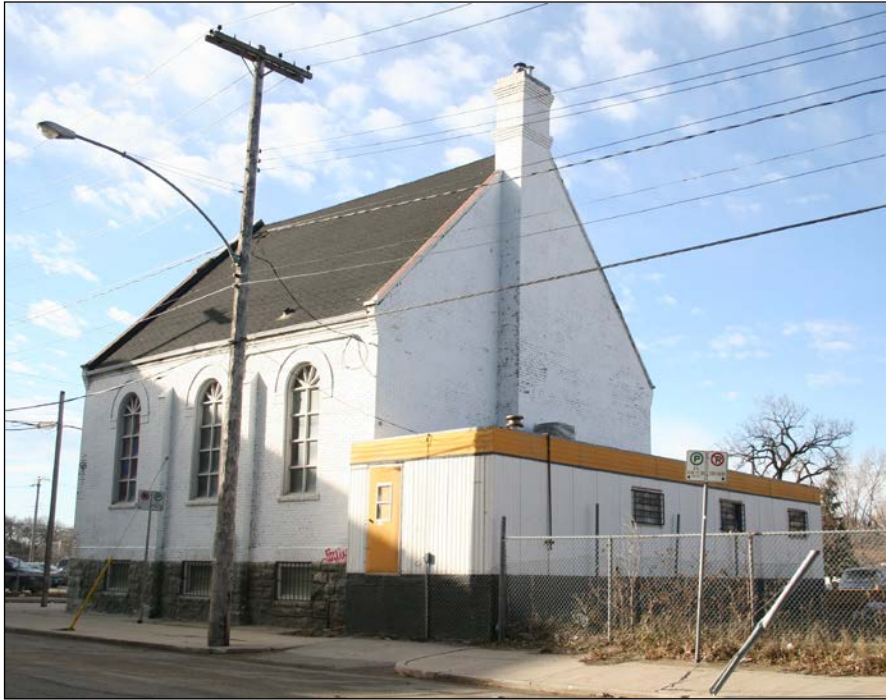
East and rear (north) façades, 2006
