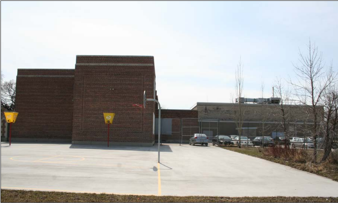
South façade and addition, 2008
