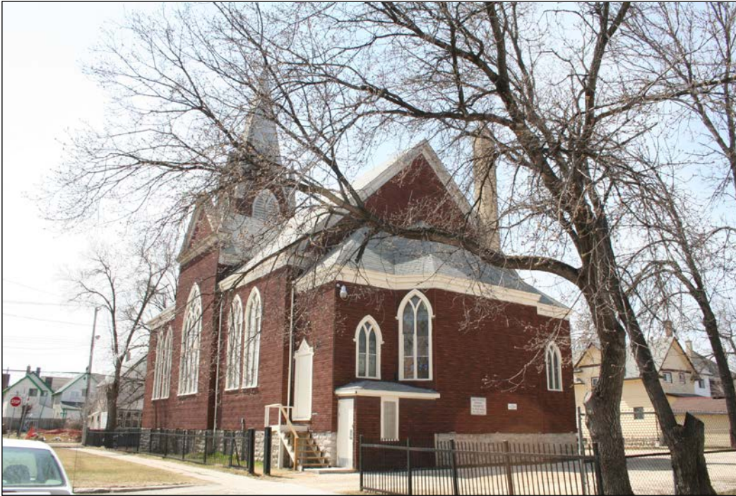
Rear (north) and east façades, 2009
