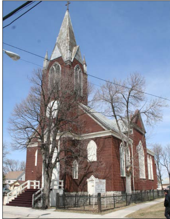
Front (south) and east façades, 2009
