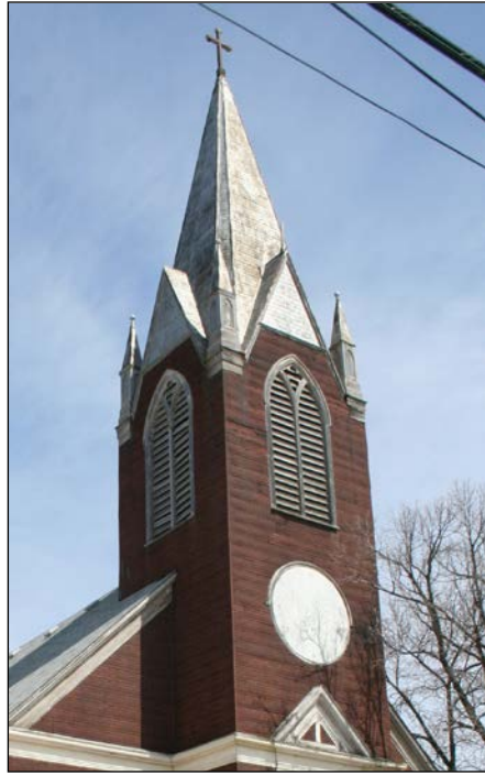
Detail of tower, 2009
