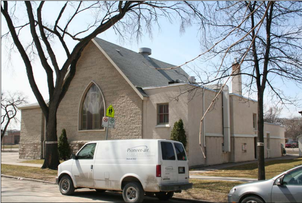
Rear (north) and east façades, 2009
