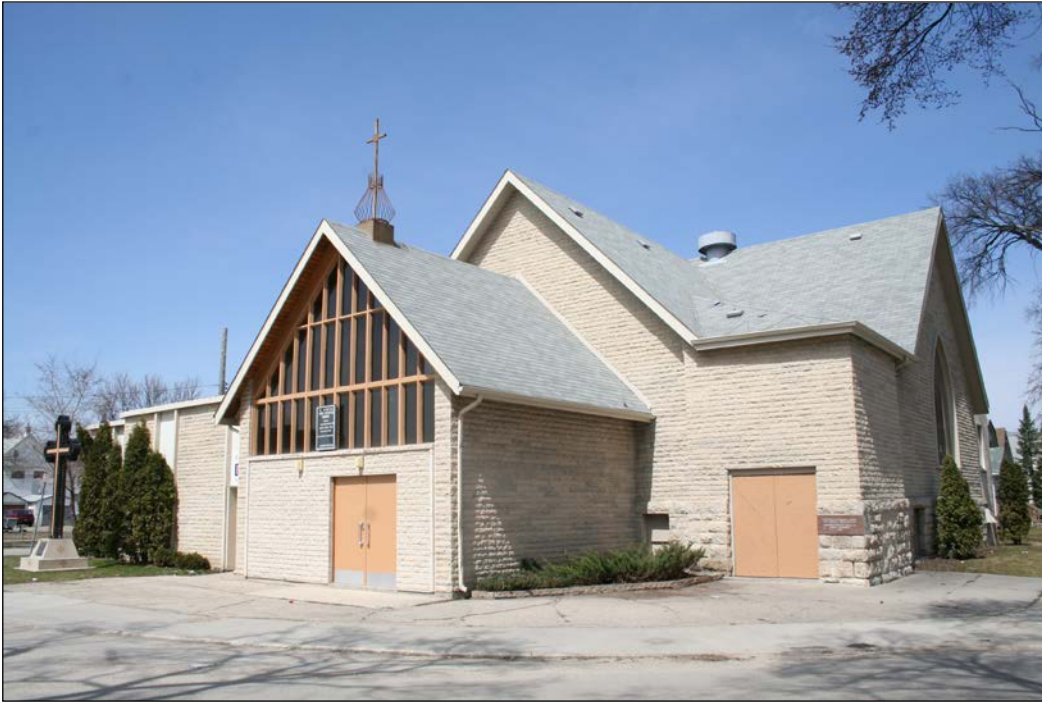
Front (south) and east façades, 2009
