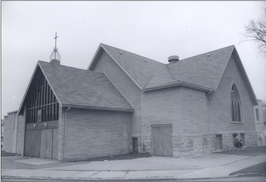
Front (south) and east façades, 1978
