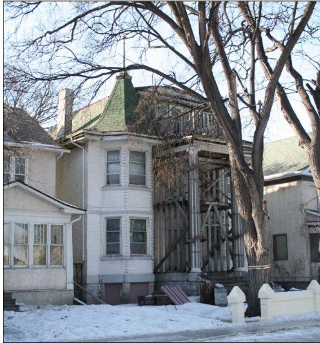
Front (east) and south façades, 2009
