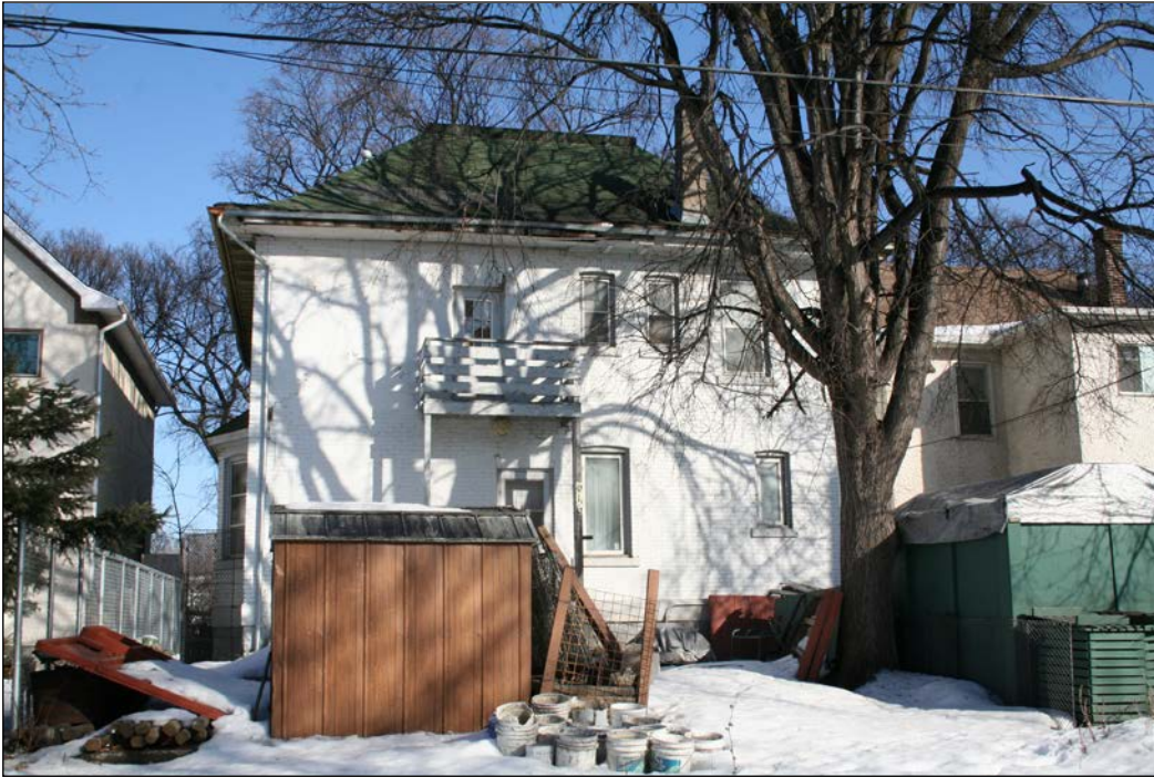
Rear (west) façade, 2009
