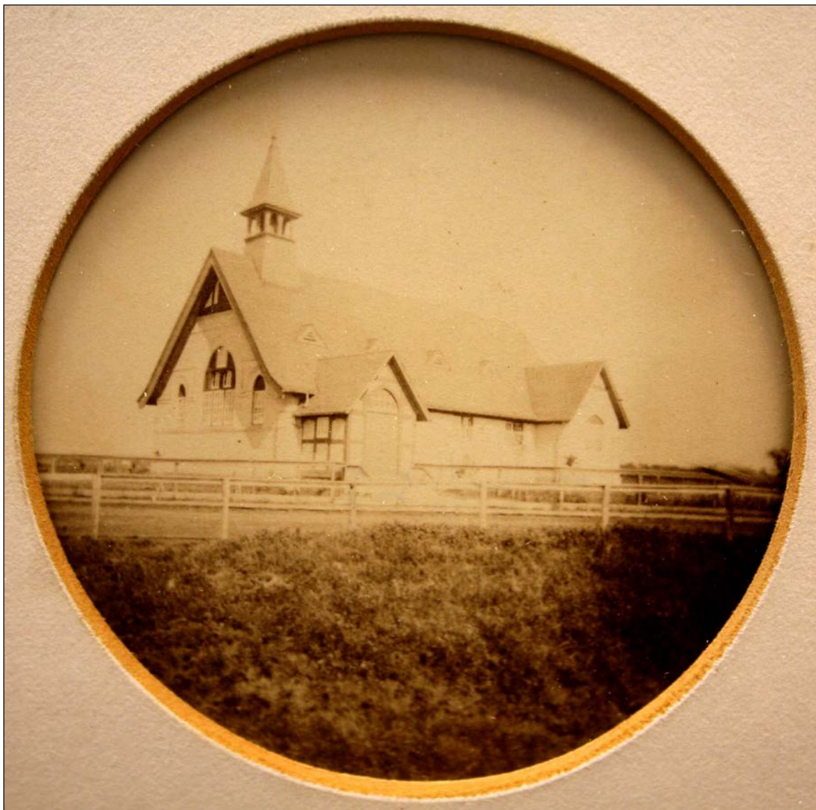
Plate 6 – The Parish Hall (originally known as the Sunday School Building, pictured shortly after construction in 1887. Original elements no longer extant include the small gable dormers and the bell tower. The picture also shows the west end that would be covered by the 1915 addition. (Courtesy of St. John’s Cathedral Archives, Code Collection.) )
