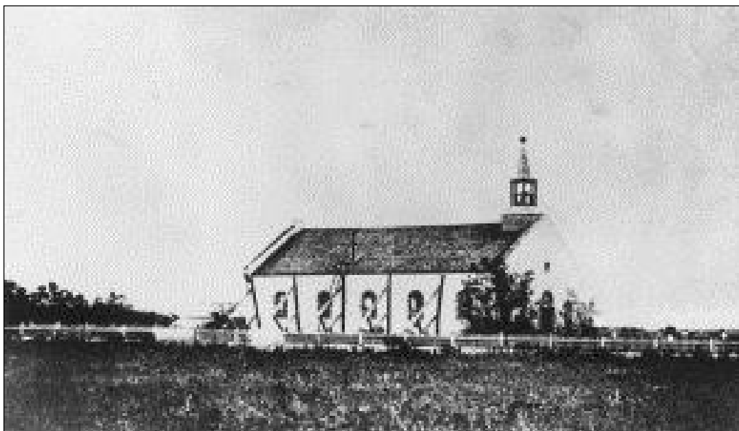
Plate 3 – St. John’s Anglican Church and later Cathedral, ca.1853. The wood buttresses were necessitated by the severe flood of 1852 that structurally damaged the building. ( St. John’s Cathedral website. )
