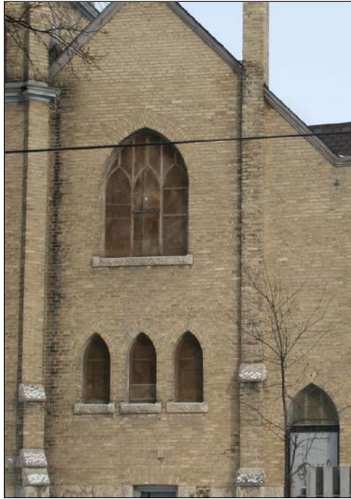
South façade detail, 2009
