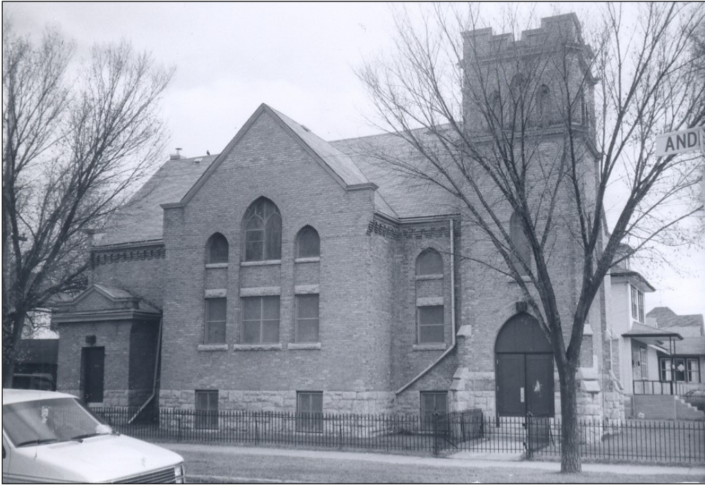
Front (east) façade detail, 1978
