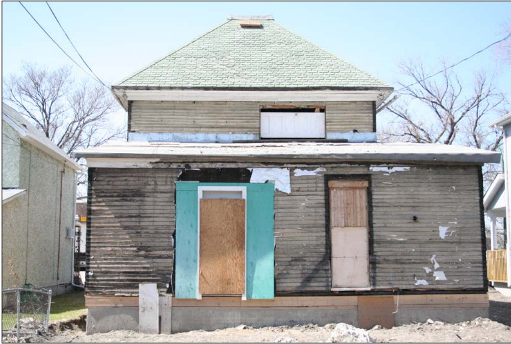
Rear (east) façade, 2007
