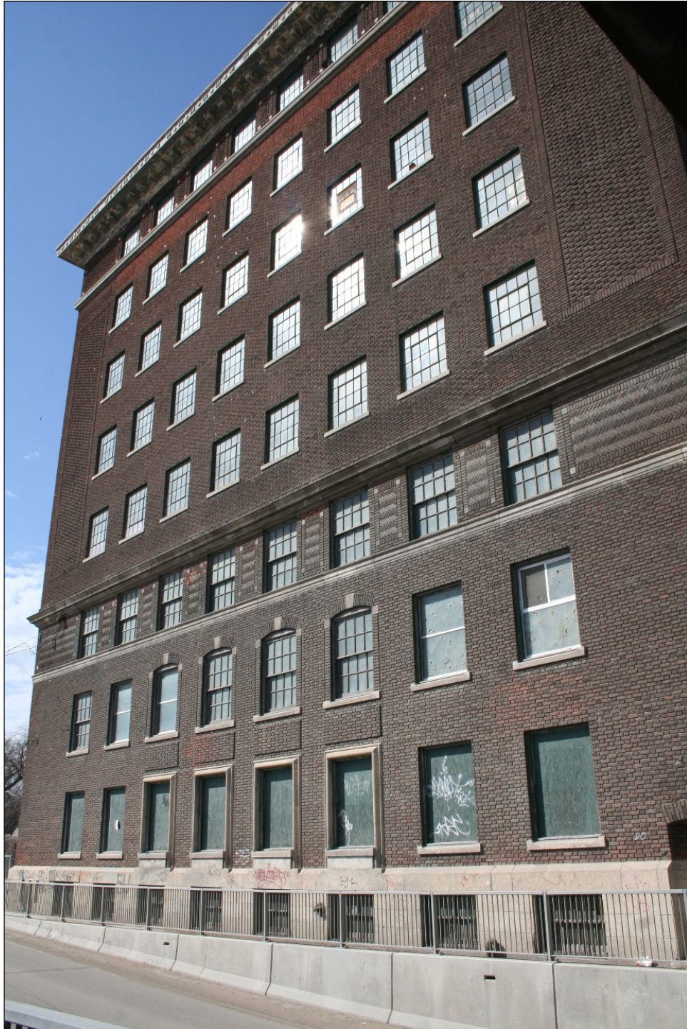
Plate 8 – J.R. Watkins Company Warehouse, 90 Annabella Street, east façade (facing Annabella Street), 2015. (M. Peterson, 2015.)
