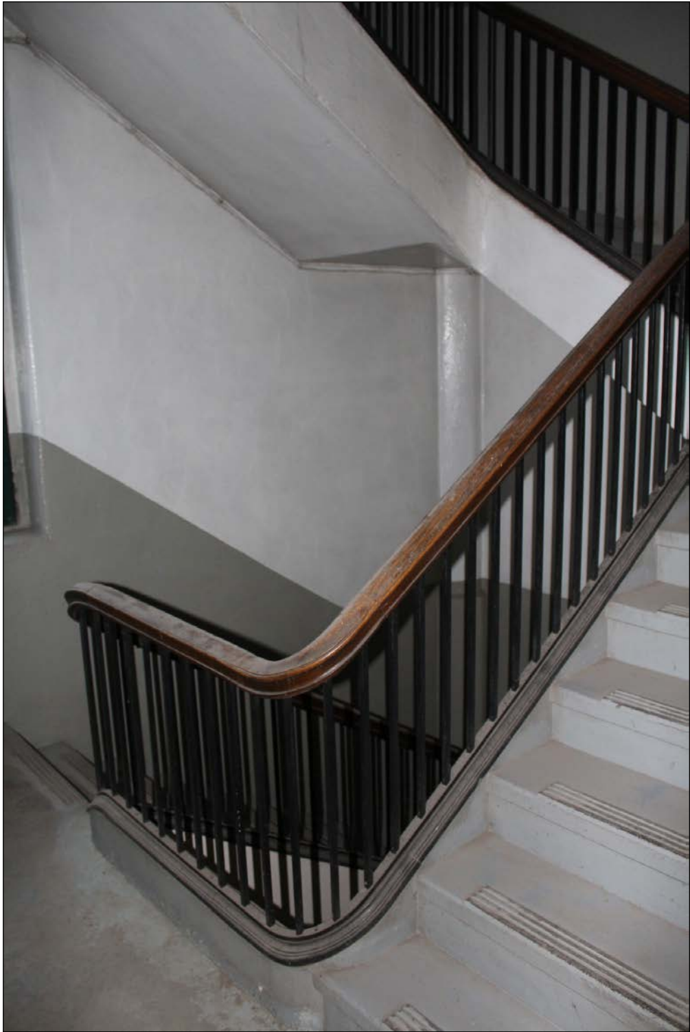
Plate 16 – J.R. Watkins Company Warehouse, 90 Annabella Street, east side staircase, 2016. (M. Peterson, 2016.)
