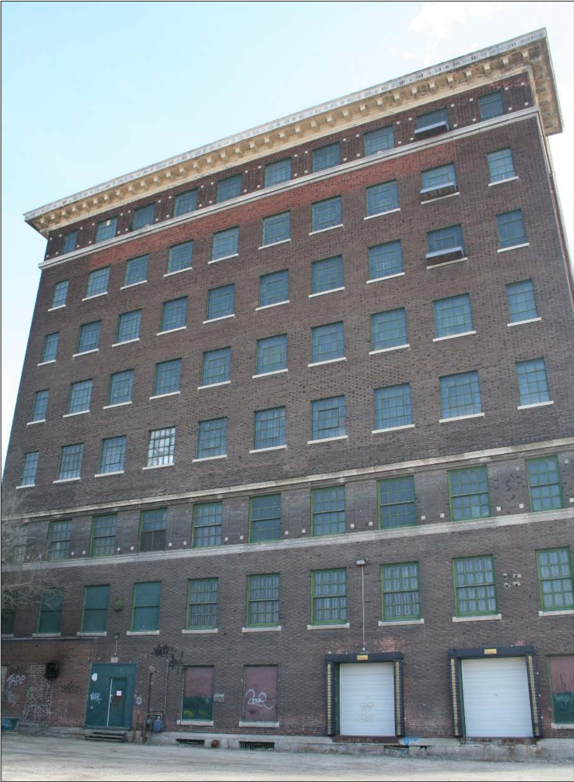
Plate 11 – J.R. Watkins Company Warehouse, 90 Annabella Street, west façade, 2015. (M. Peterson, 2015.)
