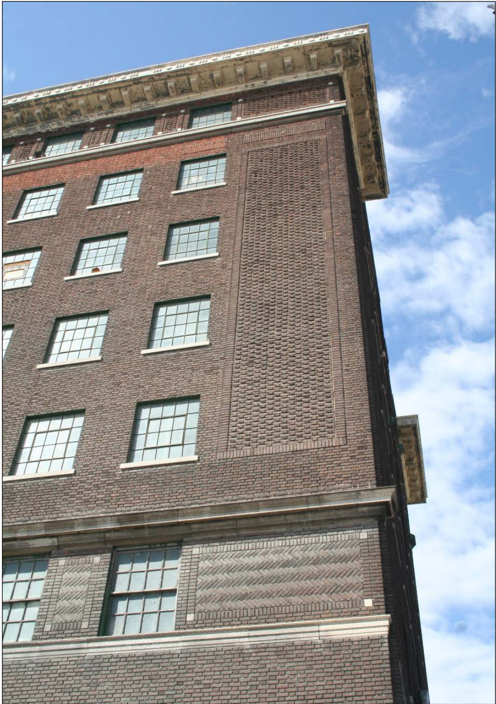
Plate 9 – J.R. Watkins Company Warehouse, 90 Annabella Street, detail of east façade showing herringbone and checkerboard brick panels, 2015. (M. Peterson, 2015.)
