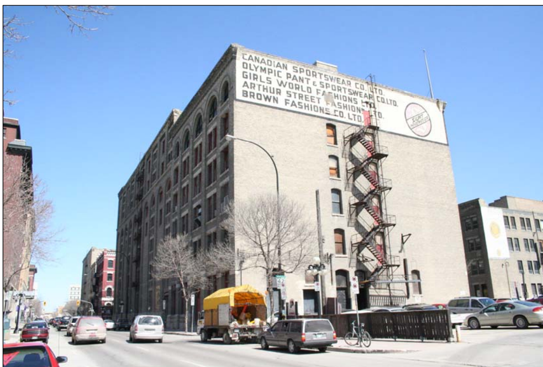
Plate 12 – Robinson, Little & Company Building, 54 Arthur Street, west and south sides, 2007. (M. Peterson, 2007.)
