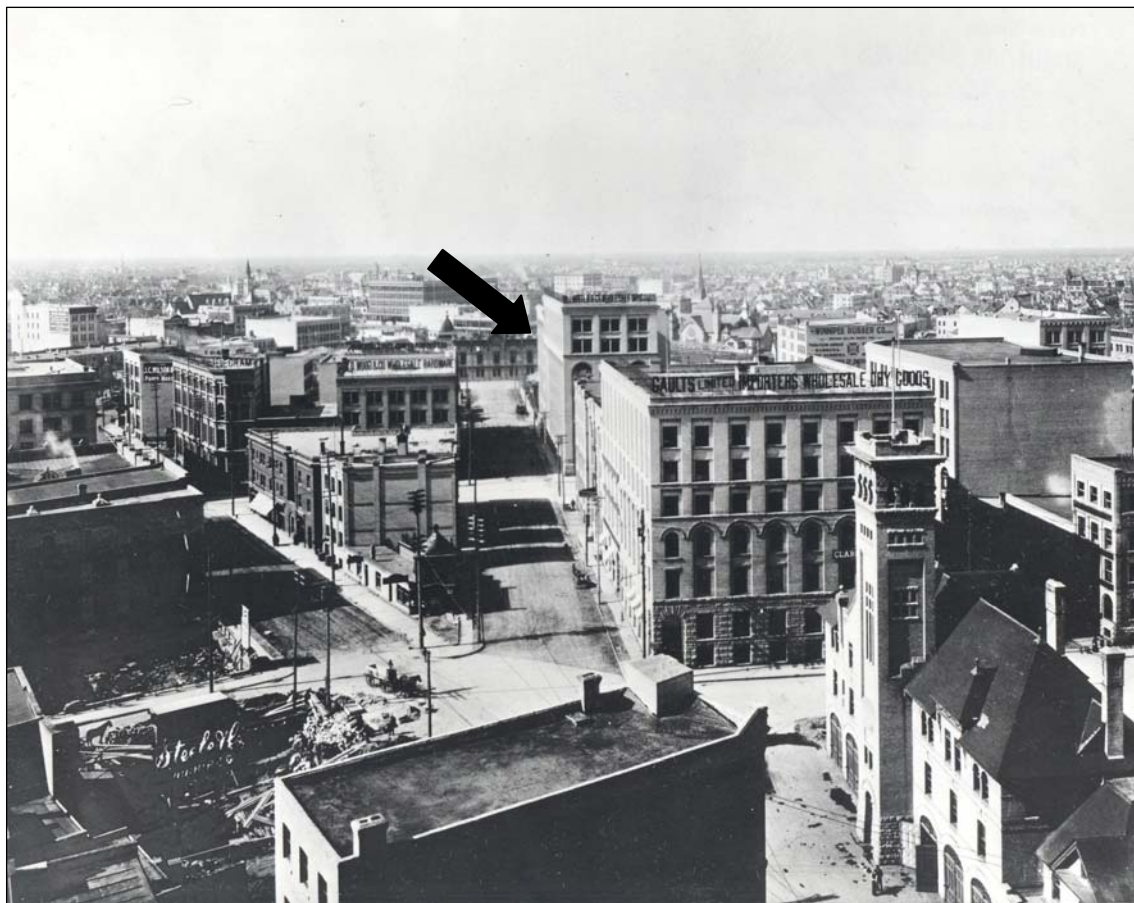
Plate 1 – Looking south along Arthur Street from Bannatyne Avenue into the heart of Winnipeg’s Exchange District west of Main Street, ca.1905. The newly completed Robinson, Little & Company Building (arrow) is just visible behind the R.J. Whittle Building. ( Courtesy of the Archives of Manitoba, Winnipeg- Views c1905- 2. )
