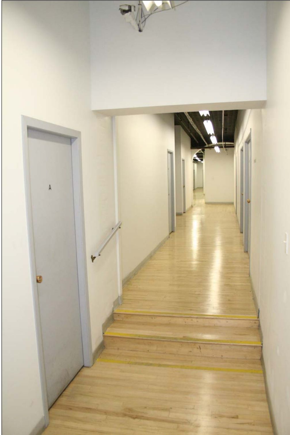
Plate 17 – Robinson, Little & Company Building, 54 Arthur Street, 6 th floor hallway. Similar to the other storeys, the original wood flooring has been refinished and the open warehouse space converted into offices. In almost all cases, the original high ceilings and ornamental tin cladding is unchanged. This view looks north, the two steps mark the join between the two buildings, #54 Arthur Street in the foreground and #70 Arthur Street beyond the steps. (M. Peterson, 2007.)
