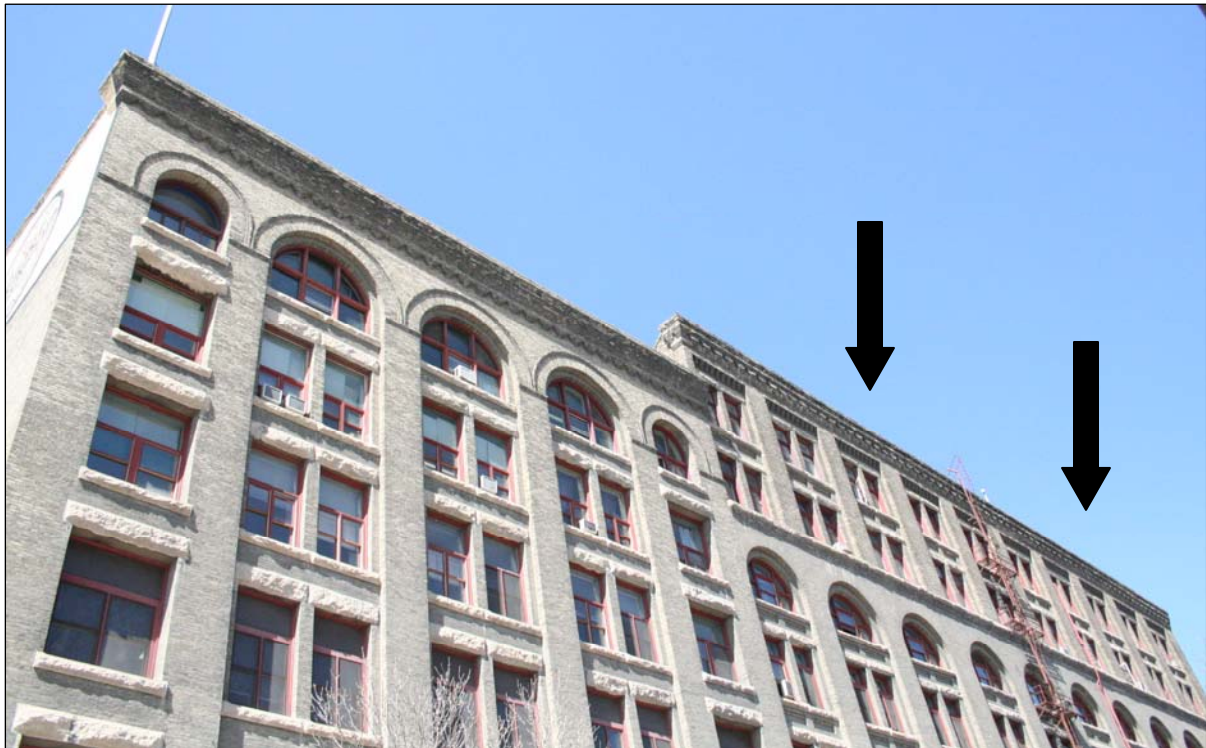
Plate 16 – Robinson, Little & Company Building, 54 Arthur Street and R.J. Whitla & Company Building, 70 Arthur Street, east side upper storey detail, 2007. Note that the upper two floors of the later building (arrows) were completed in 1904, after the construction of the Robinson, Little & Company Building. (M. Peterson, 2007.)
