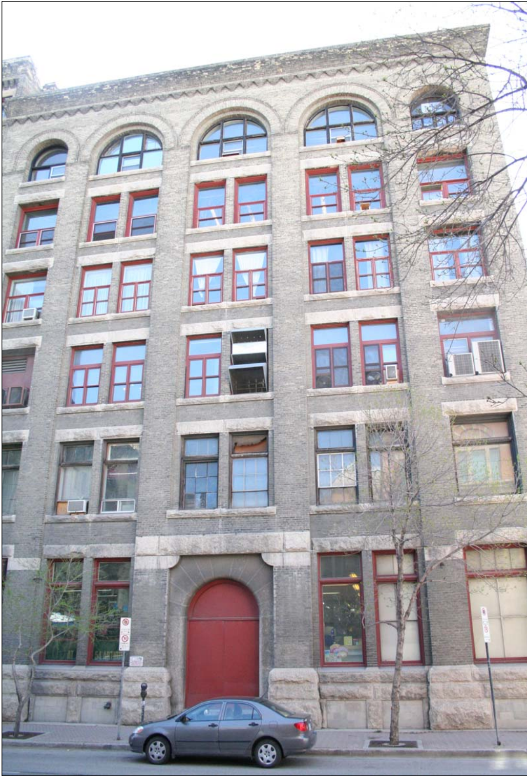
Plate 5 – Robinson, Little & Company Building, 54 Arthur Street, west façade, 2007. (M. Peterson, 2007.)
