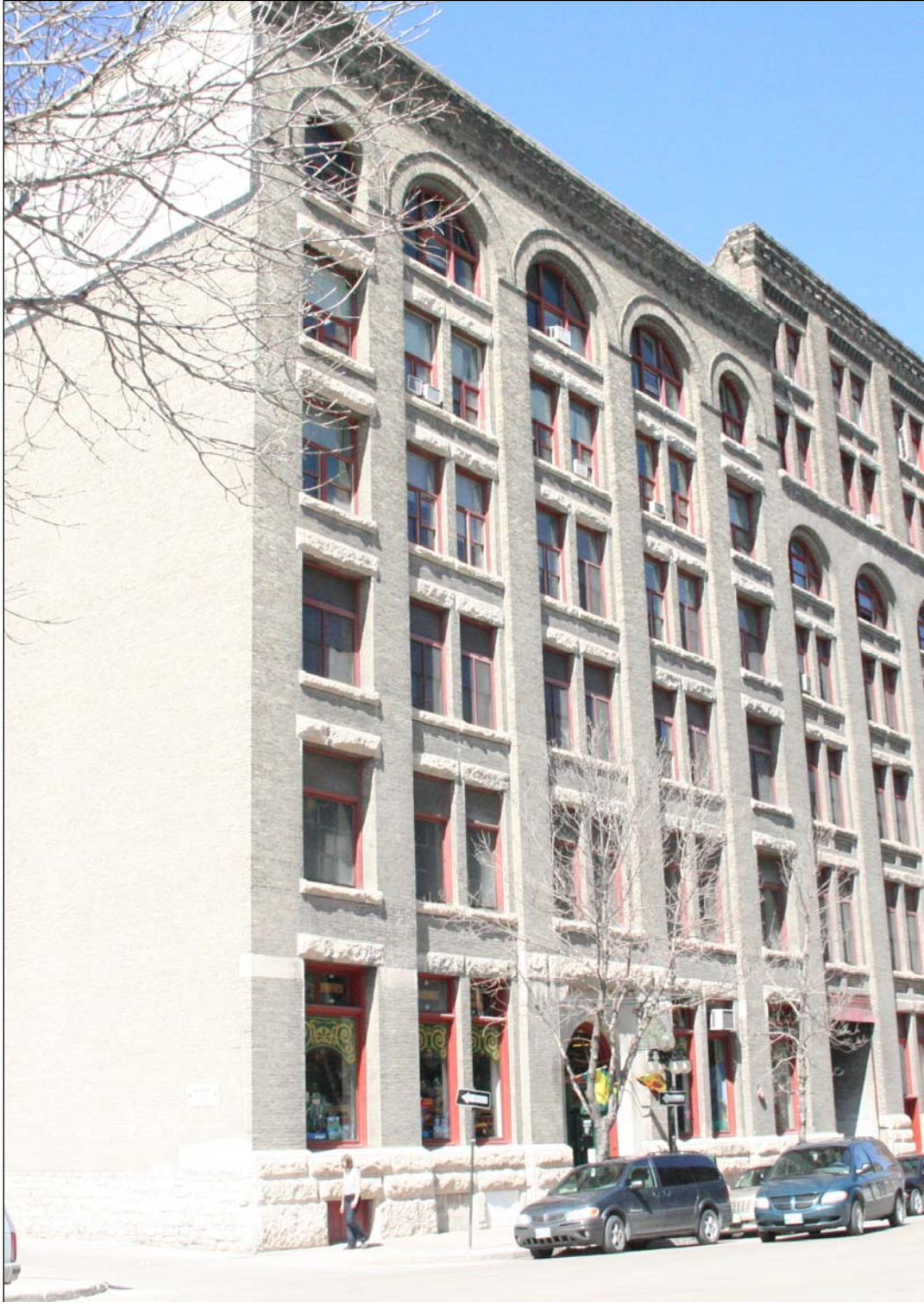
Plate 4 – Robinson, Little & Company Building, 54 Arthur Street, east façade, 2007. ( M. Peterson, 2007. )
