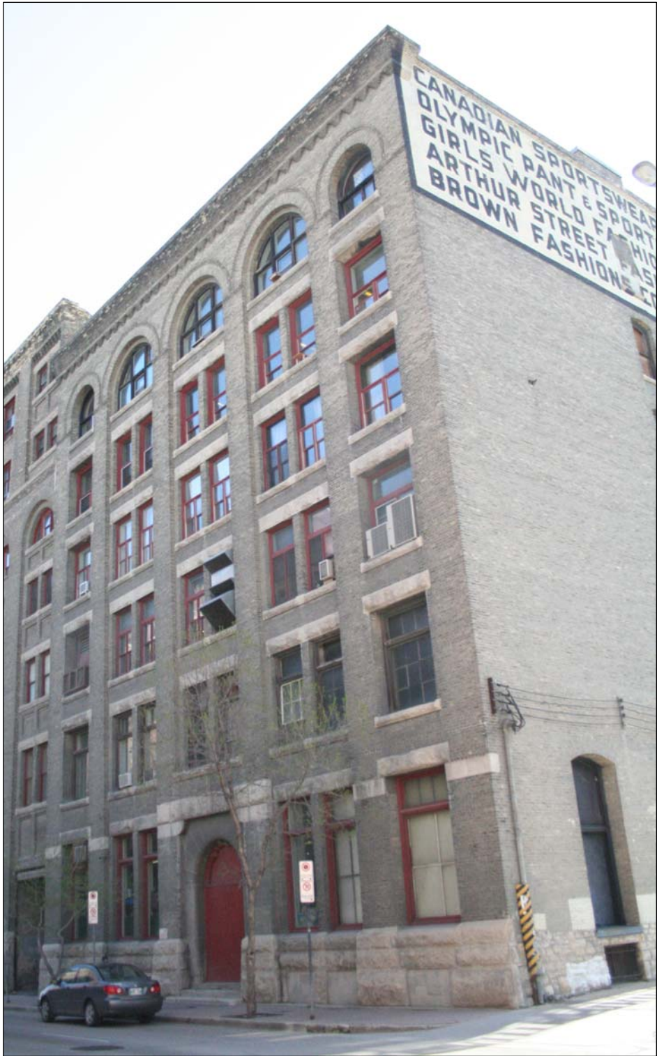
Plate 9 – Robinson, Little & Company Building, 54 Arthur Street, west side, 2007. (M. Peterson, 2007.)
