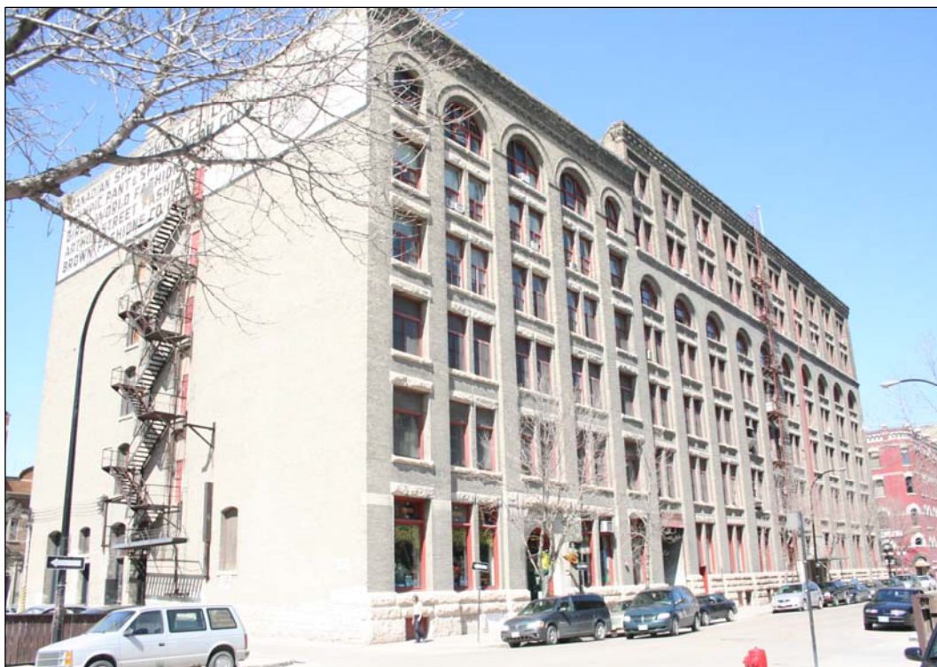
Plate 11 – Robinson, Little & Company Building, 54 Arthur Street and R.J. Whitla & Company Building, 70 Arthur Street, east sides, 2007. (M. Peterson, 2007.)
