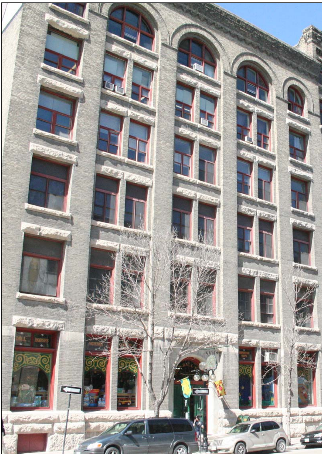
Plate 7 – Robinson, Little & Company Building, 54 Arthur Street, detail of east side, 2007. ( M. Peterson, 2007. )
