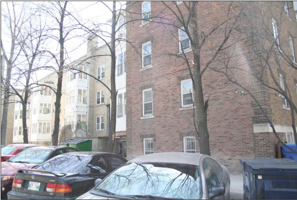
Front (north) and east façades, 2007
