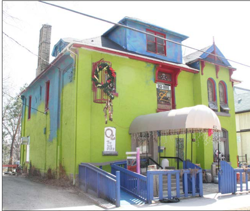
Front (north) and east façades, 2007
