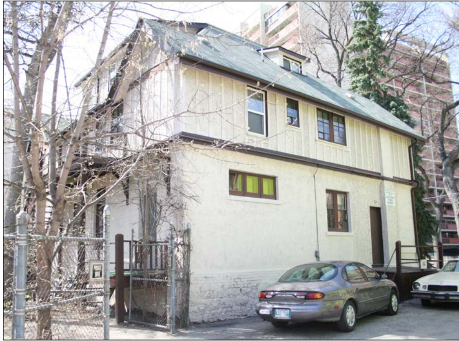
Front (north) and east façades, 2007
