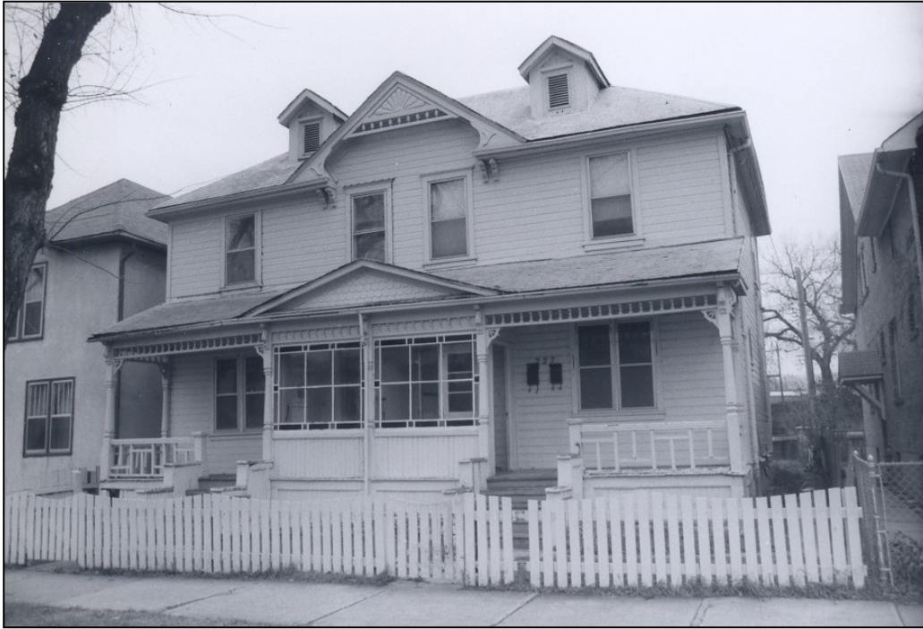
Front (west) façade, 1978
