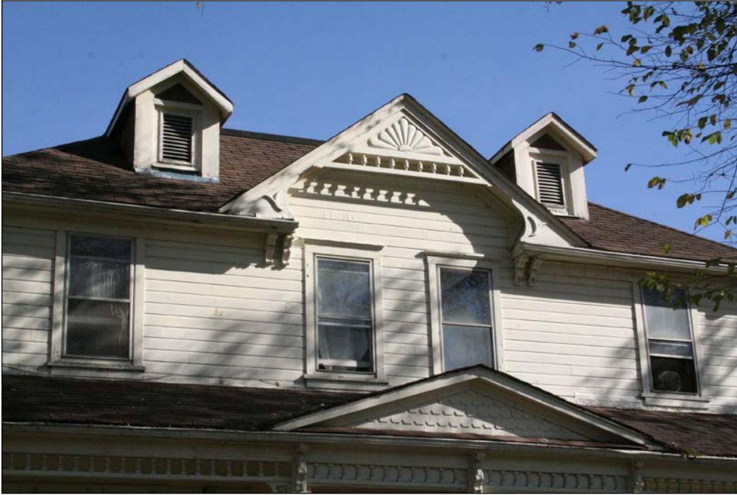
Detail of front (west) façade, 2007
