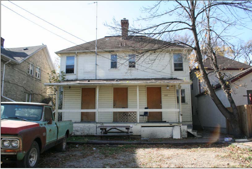
Rear (east) façade, 2007
