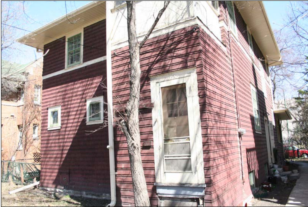
Rear (west) and south façades, 2007
