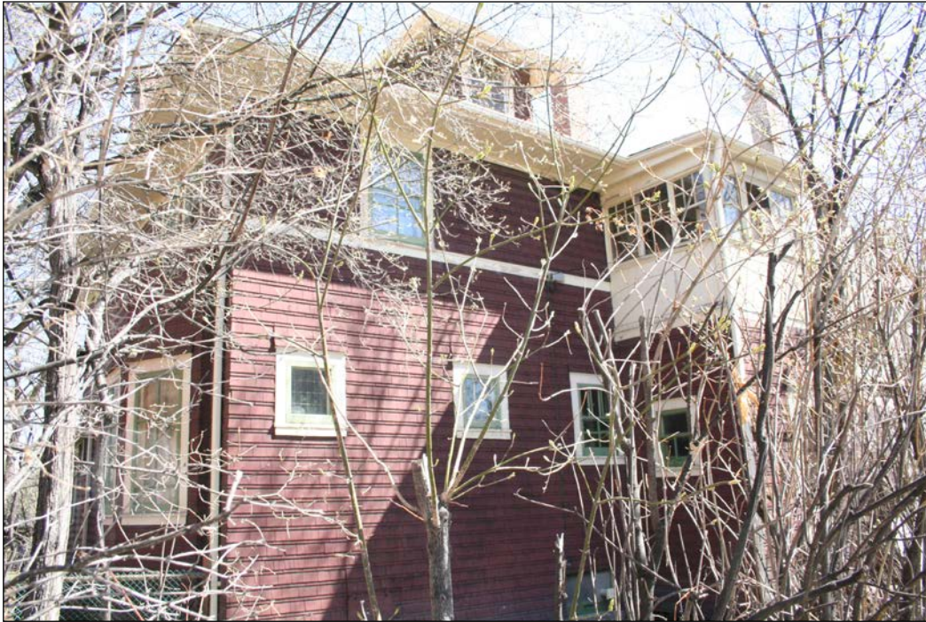
Rear (west) and north façades, 2007
