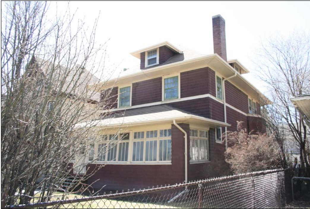
Front (east) and north façades, 2007
