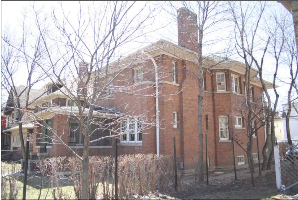
Front (east) and north façades, 2007
