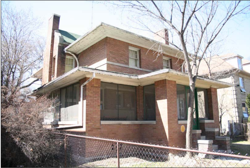
Front (east) and south façades, 2007
