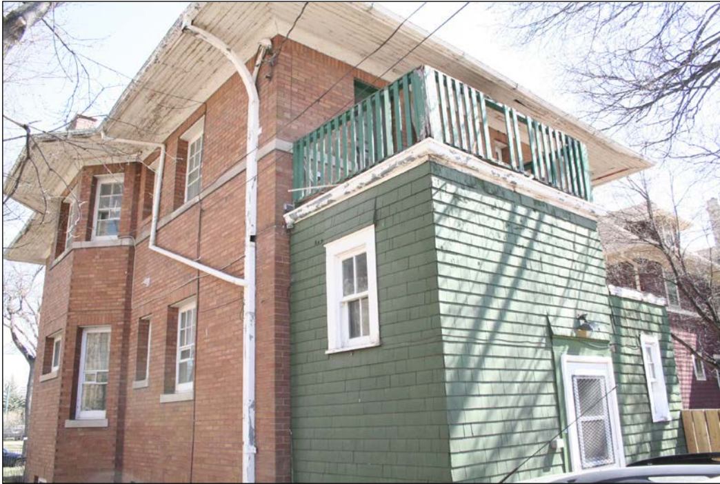
Rear (west) and north façades, 2007
