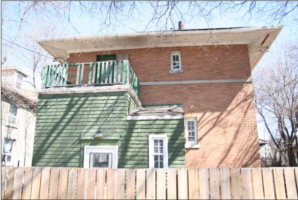
Rear (west) façade, 2007
