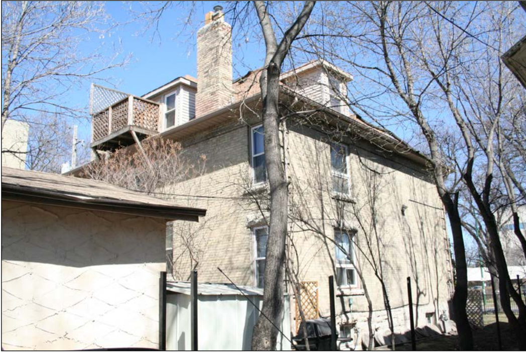
Rear (west) and south façades, 2007
