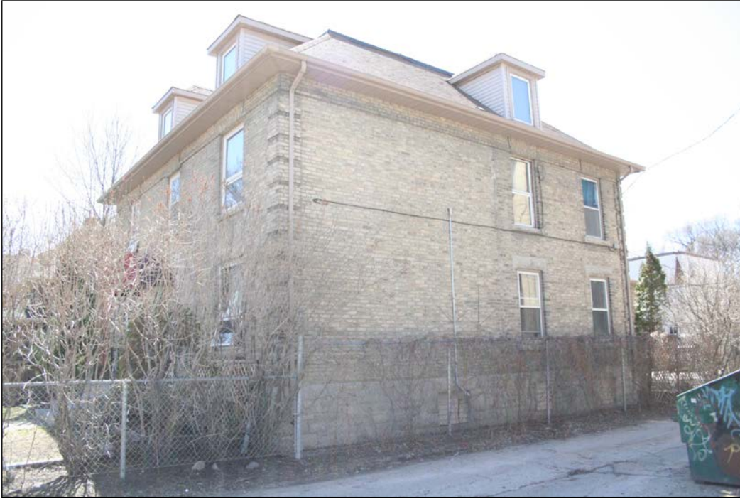
Front (east) and north façades, 2007
