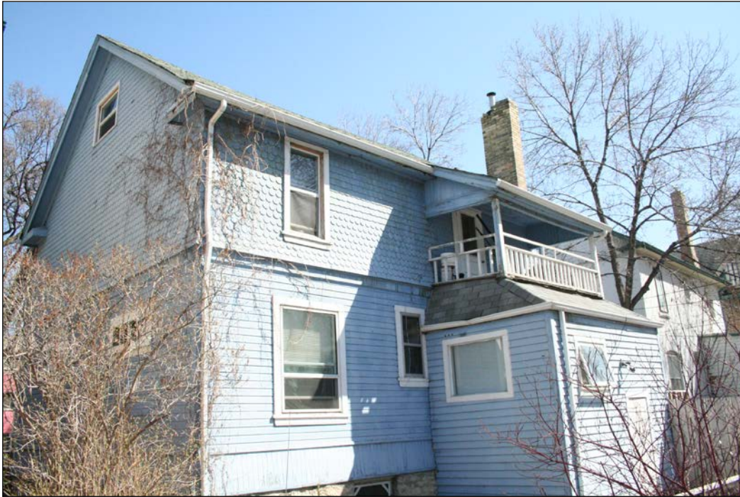
Rear (west) and north façades, 2007
