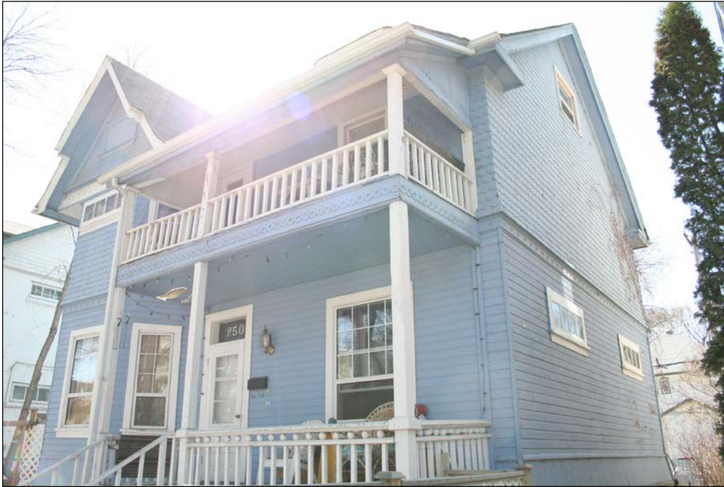
Front (east) and north façades, 2007
