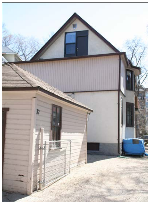
Rear (north) and west façades, 2007
