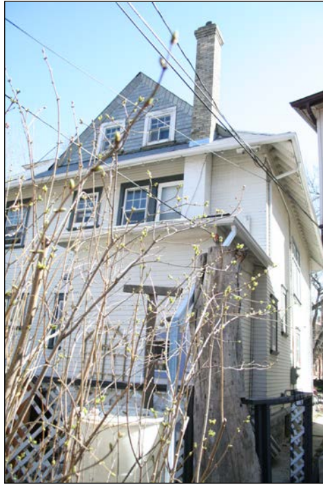
Rear (north) and west façades, 2007
