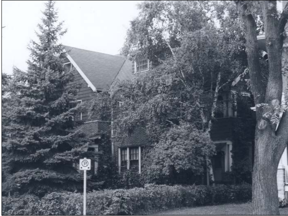
Front (east) façade, 1978
