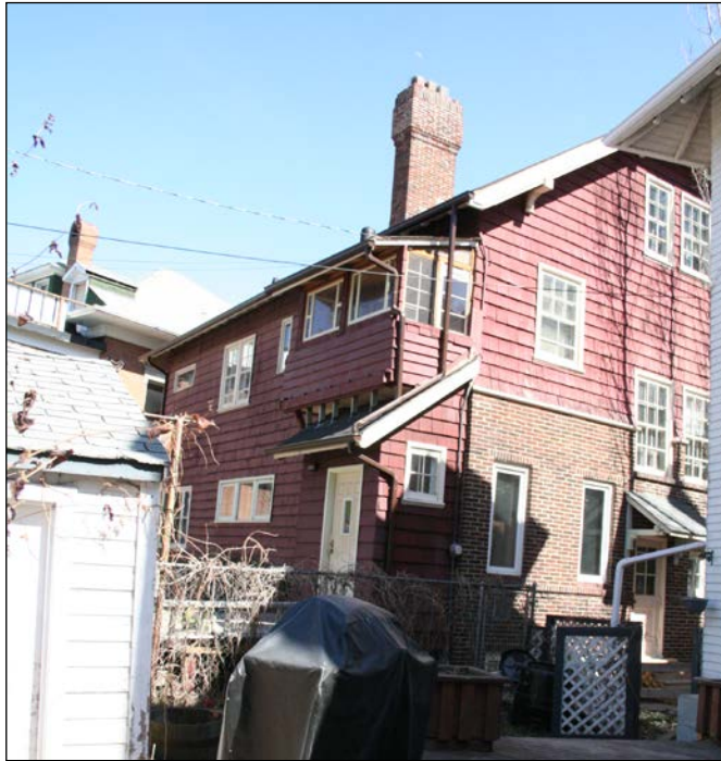
Rear (north) and west façades, 2007
