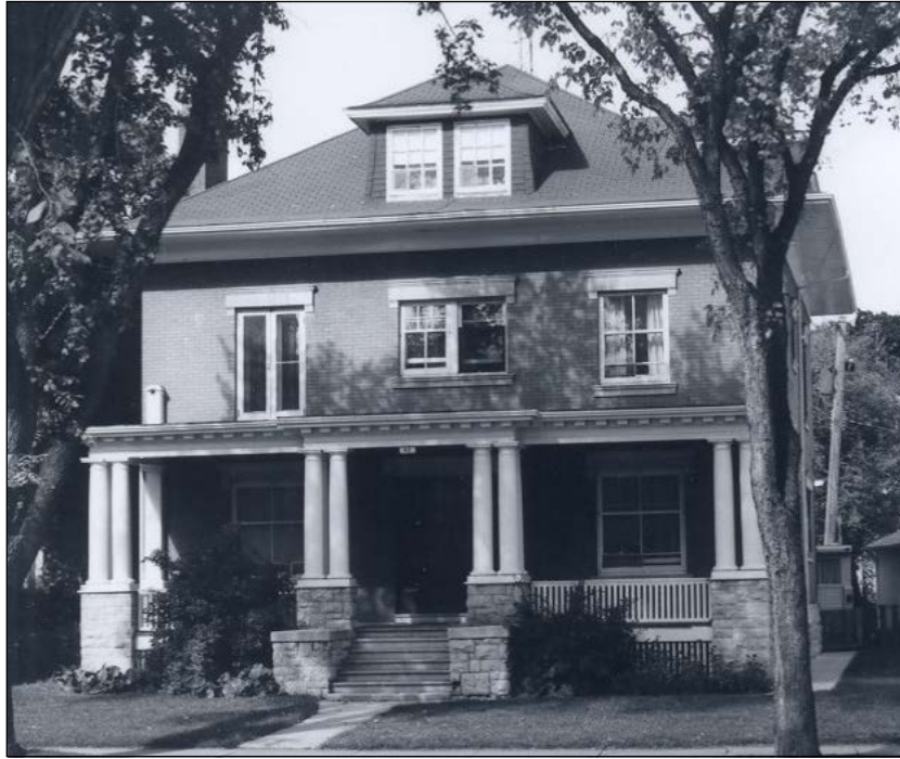
Front (east) façade, 1978
