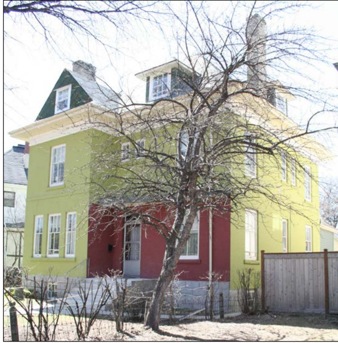
Front (east) and north façades, 2007
