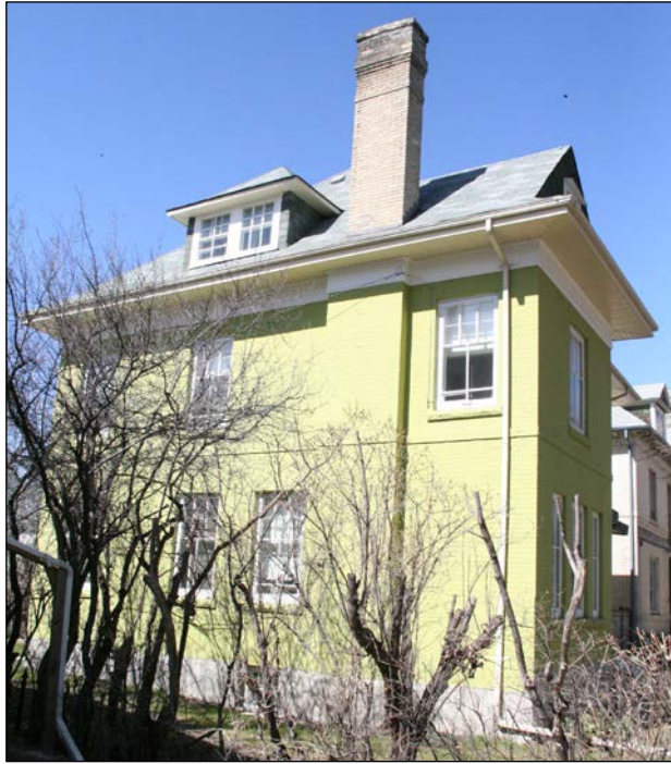
Front (east) and south façades, 2007
