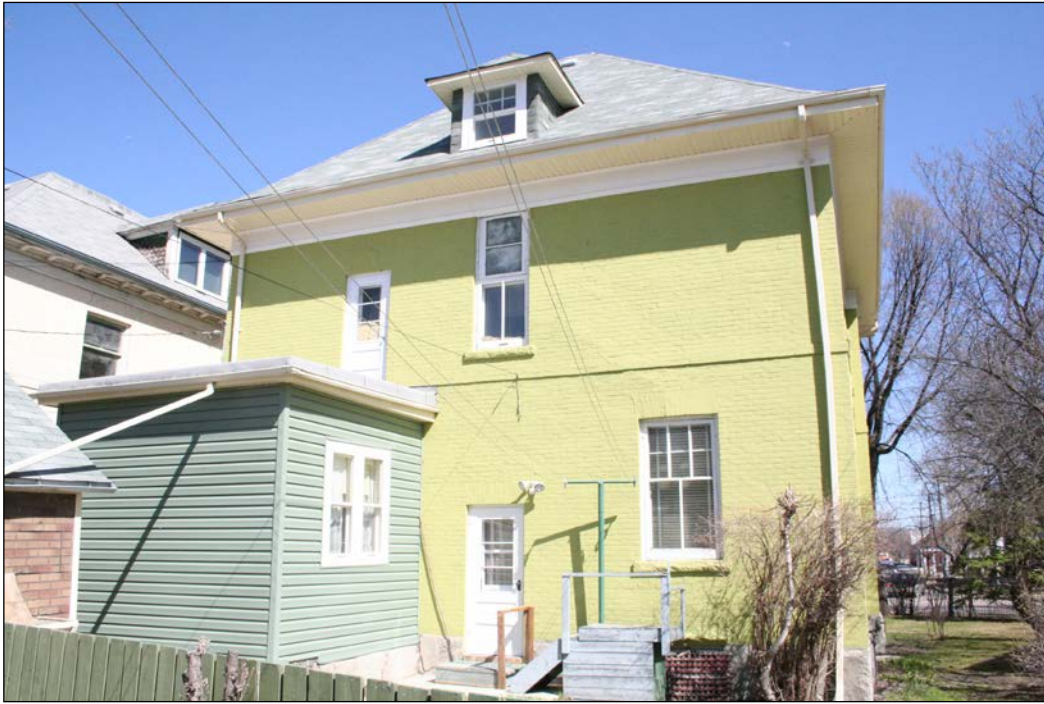
Rear (west) façade, 2007
