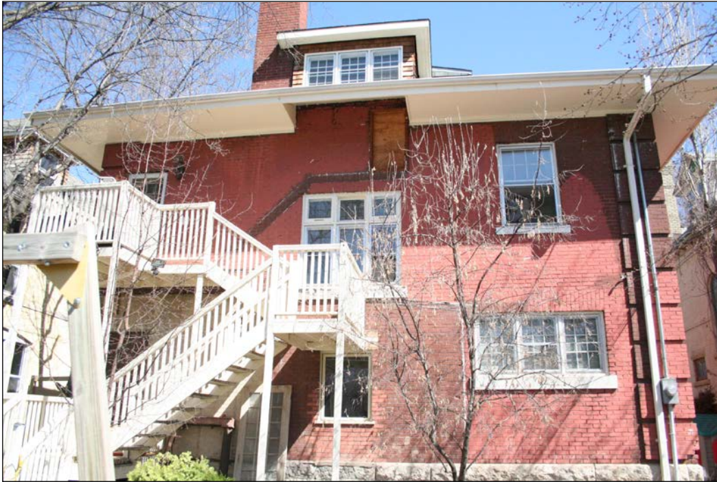
Rear (west) façade, 2007
