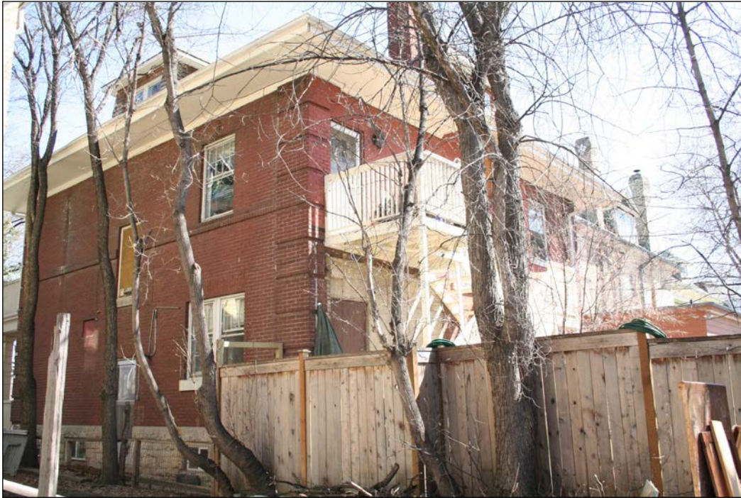
Rear (west) and north façades, 2007
