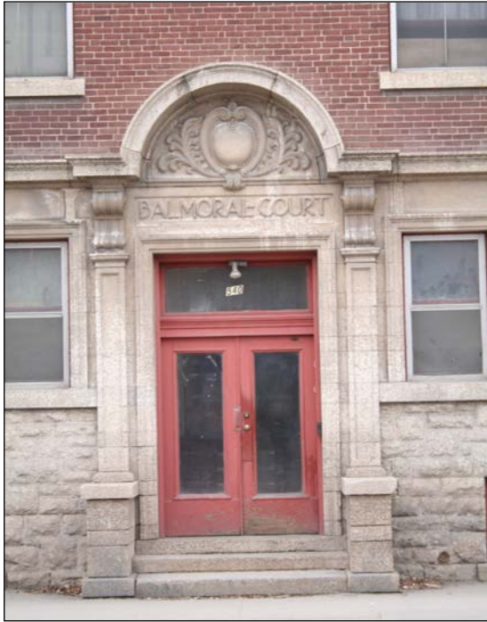
Front (east) façade detail, 2006
