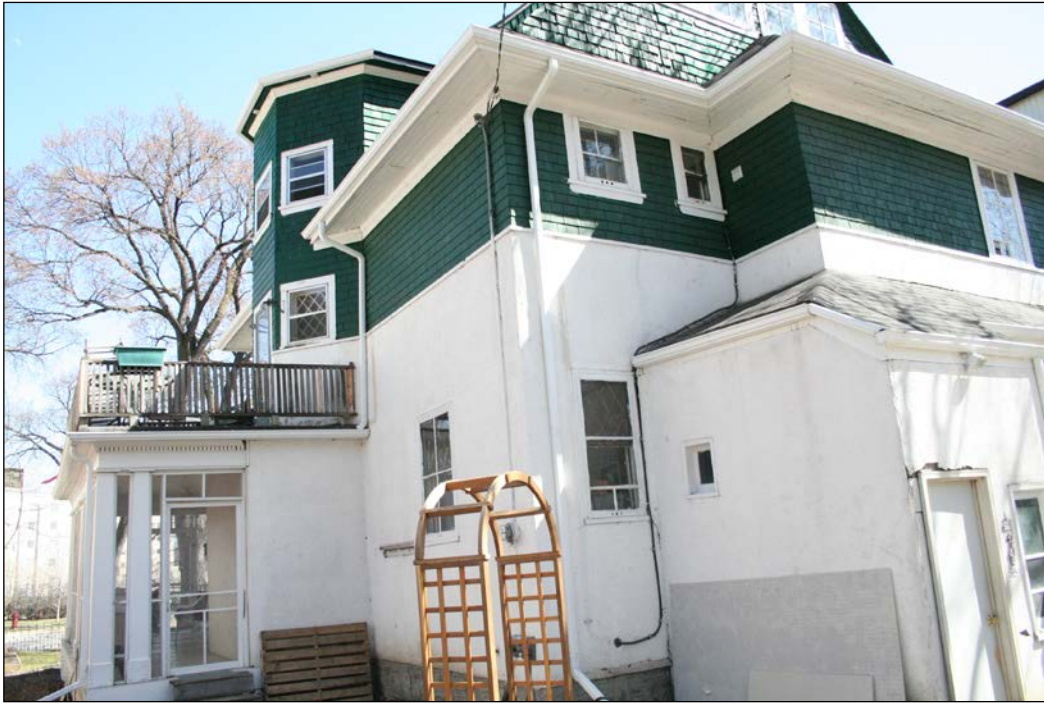
Rear (west) and north façades, 2007
