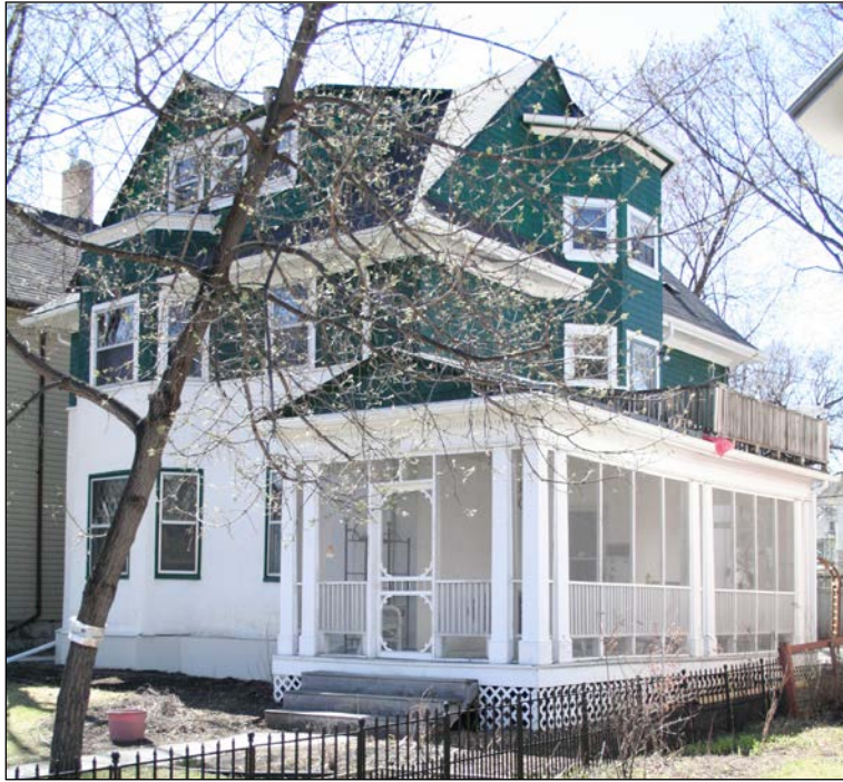
Front (east) and north façades, 2007
