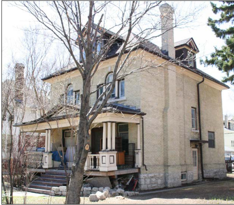
Front (east) and north façades, 2007
