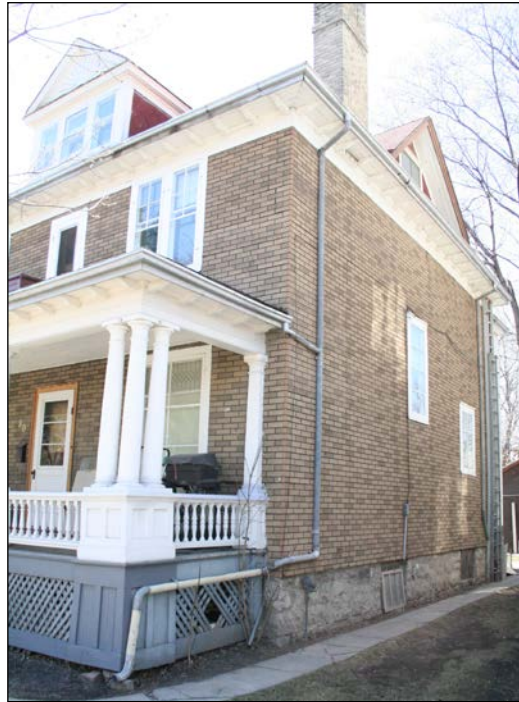
Front (east) and north façades, 2007
